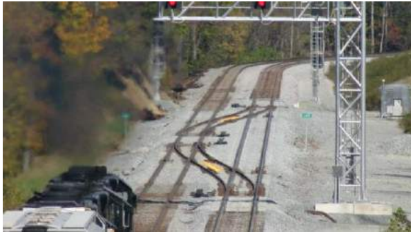
Figure 10. Compacting the Asphalt Layer and the finished Asphalt Underlayment Layer in preparation for placing a No. 24 Crossover (top), a Finished Crossover at CP Lake and the Two WILDs near China Grove (bottom).
