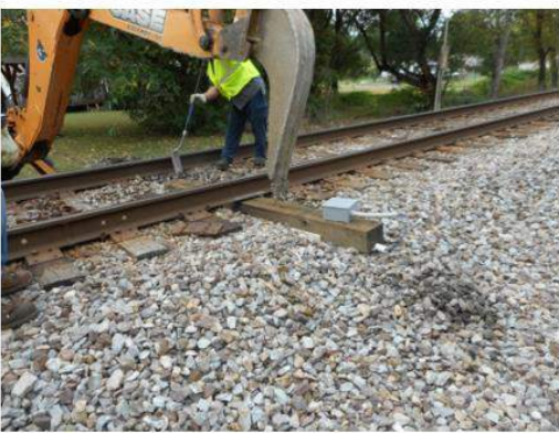
Figure 4.1.2. Inserting instrumented ties in the track.
