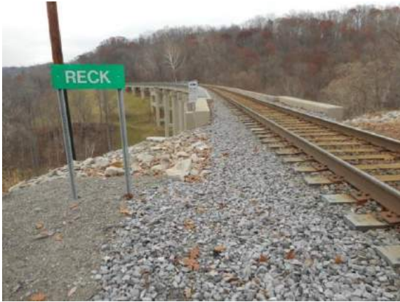
Figure 6.3b. Muldraugh Hill Bridge containing Asphalt Approaches that are 50 ft (15 m) long the full width of the wing walls for 25 ft (7.5 m) and an additional 25 ft (7.5 m). This particular Bridge contains Composite Ties; the other one contains Wood Ties.
