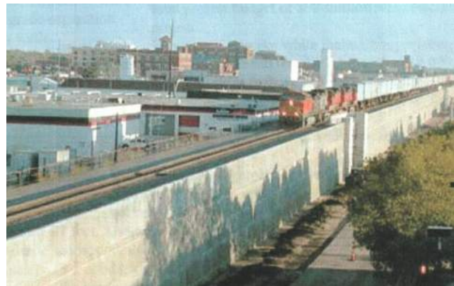
Figure. 11.1. Paving the Elevated Trackbed and the Finished Trackbed are shown in the top views. The bottom views show the exposed asphalt on the north end of the Elevated Track prior to placing the track and the precast concrete T-Walls and Mechanically Stabilized Earth Walls.
