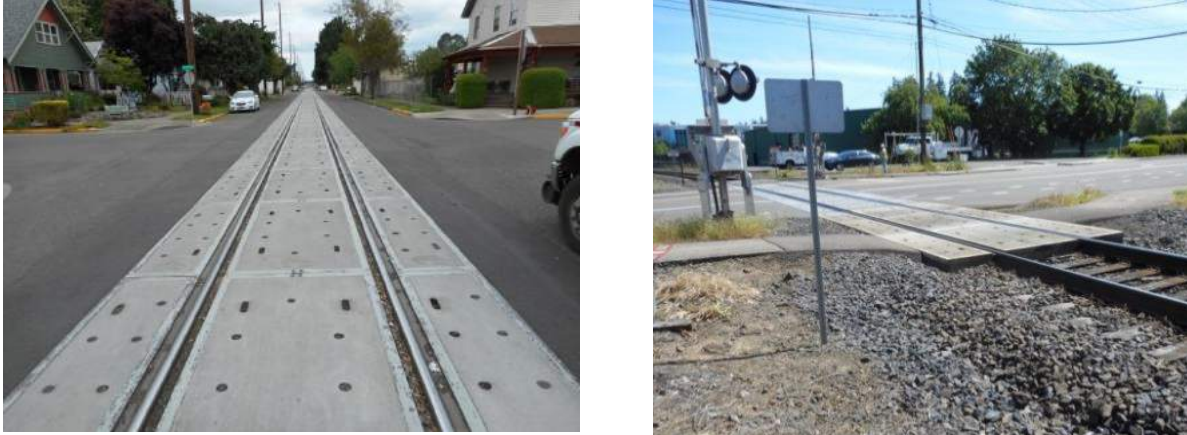
Figure 3.1. The 3,500 ft (1,100 m) long Holly Street Middle-Of-Street Crossing in Junction City (left) containing Asphalt Underlayment. Durham Avenue (right), one of 13 Crossings on the WES Line containing Asphalt Underlayment.
