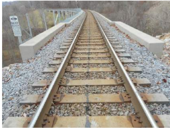
Figure 6.3b. Muldraugh Hill Bridge containing Asphalt Approaches that are 50 ft (15 m) long the full width of the wing walls for 25 ft (7.5 m) and an additional 25 ft (7.5 m). This particular Bridge contains Composite Ties; the other one contains Wood Ties.
