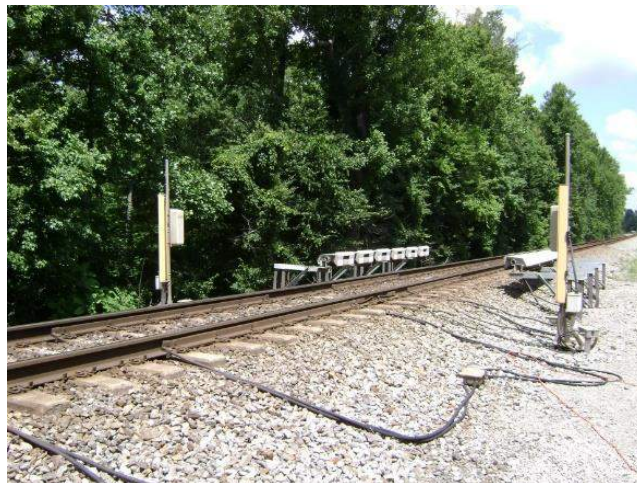
Figure 6b. Typical Salient Mk-III WILD Installation.
