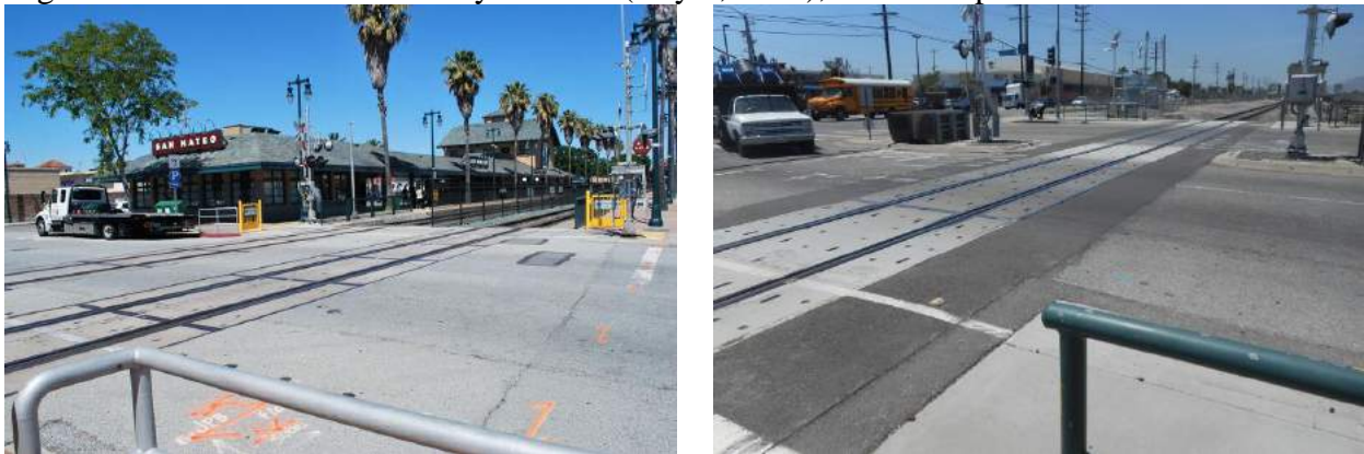
Figure 3.4. Caltrain's San Mateo 1 st Street Crossing and Station Platform (left) placed in 2,000 using Hot-Mix Asphalt Mixture and Metrolink's Osborne Street Crossing (right) in the Sun Valley Area placed in 2013 using a Cold-Mix, Polymerized Emulsion Asphalt Mixture. These Crossings have exhibited Excellent Performance, Typical of all Caltrain and Metrolink Street Crossings Underlain with Asphalt.
