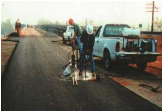
Figure 6.1. Core Drilling the Asphalt Layer in 1998, the day after the Asphalt was placed on the North Approach and a view of the North Approach in 2014, 16 years after Construction of the Bridge.
