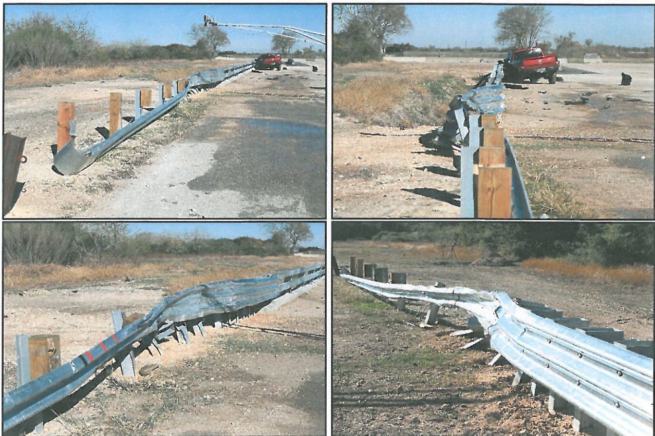
Figure 7.3. Transition after Test No. 608331-01-6.
