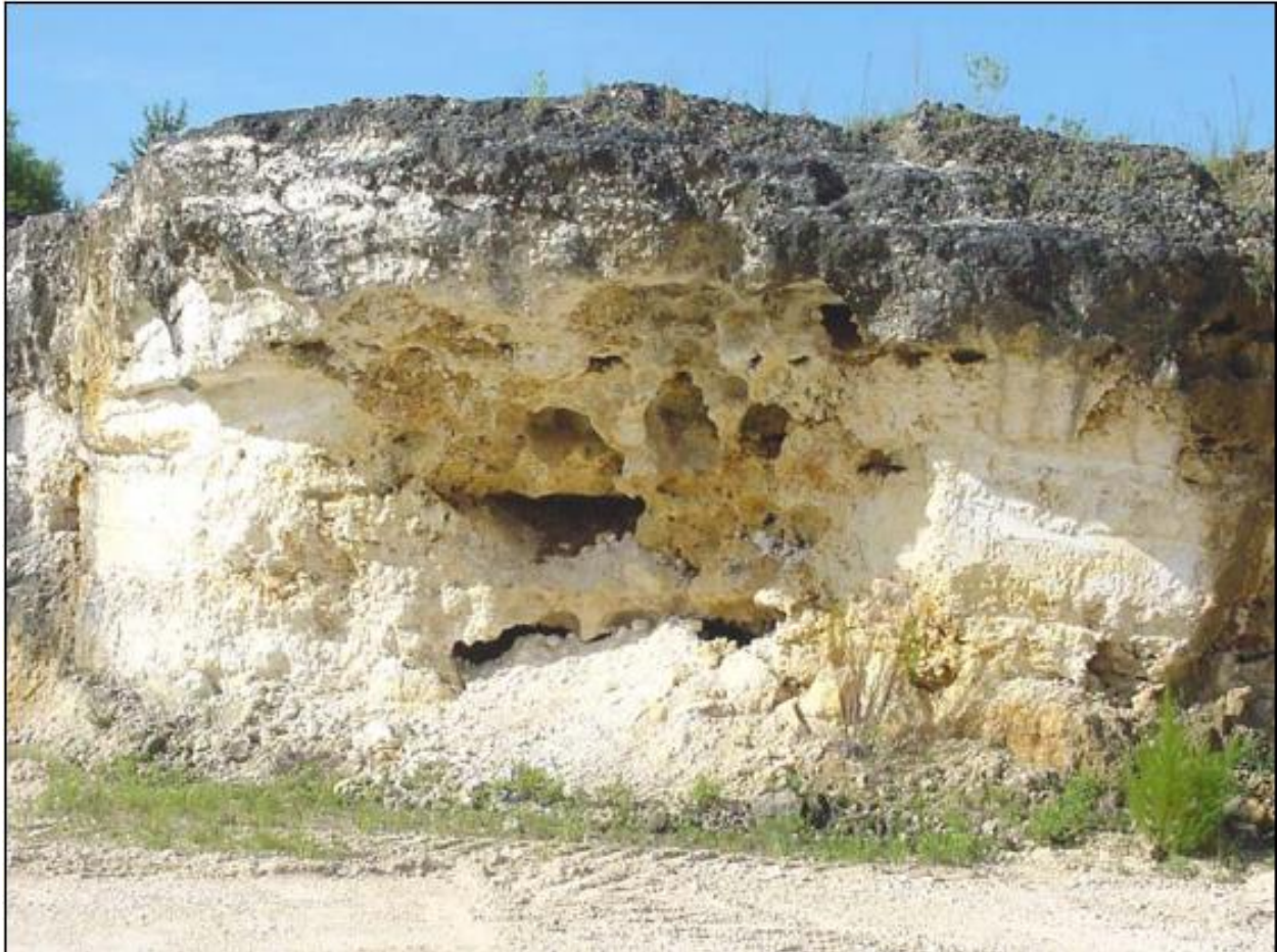
Figure 2-3. Newberry quarry excavation (Bullock, 2004)
