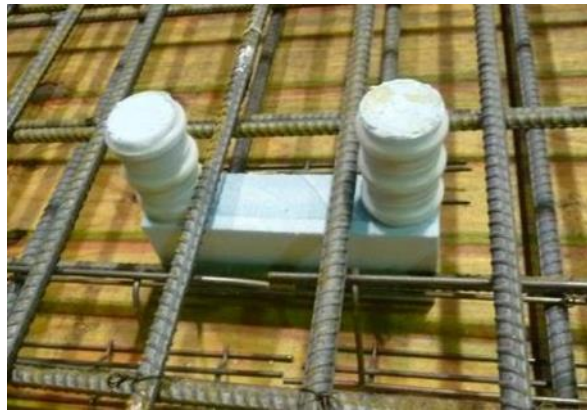
Figure 4.11. U-bar access blocks outs with terminated bottom deck steel and top deck steel positioned to be within a U-bar connection
