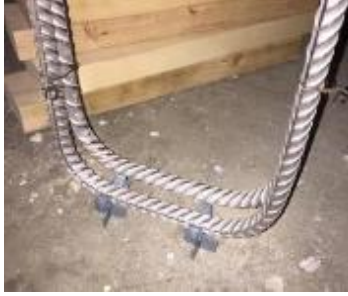
Figure 4.17. Reinforcing steel bar chairs for #5 bars
