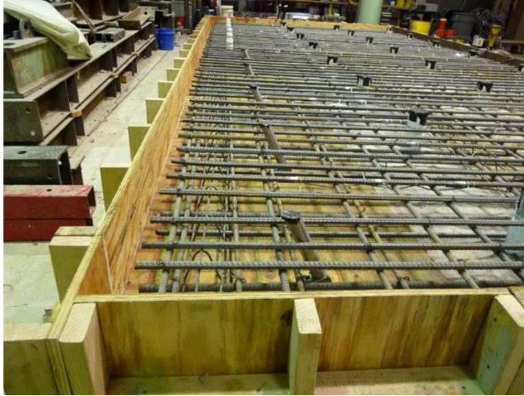
Figure 4.9. Bridge deck reinforcement
