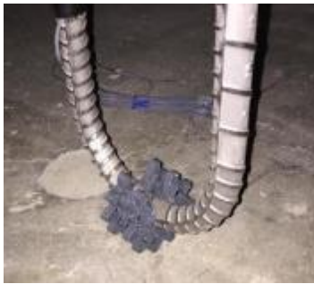
Figure 4.18. Reinforcing steel bar chairs for #7 bars
