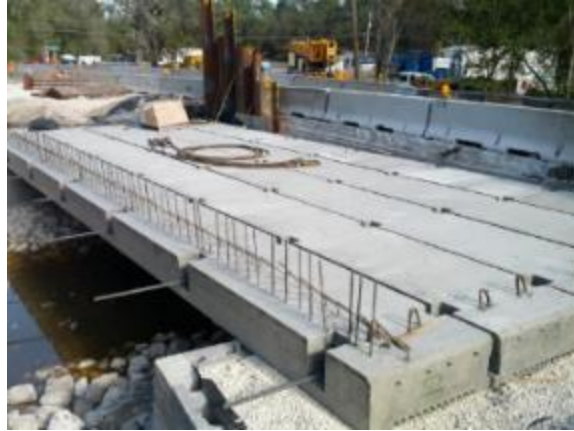
Figure 1.4. Rockridge Road bridge with exposed barrier connection reinforcement
