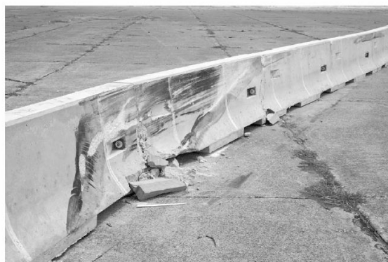
Figure 2.12. Damage to 10-ft long prefabricated barrier with X-bolt connections
