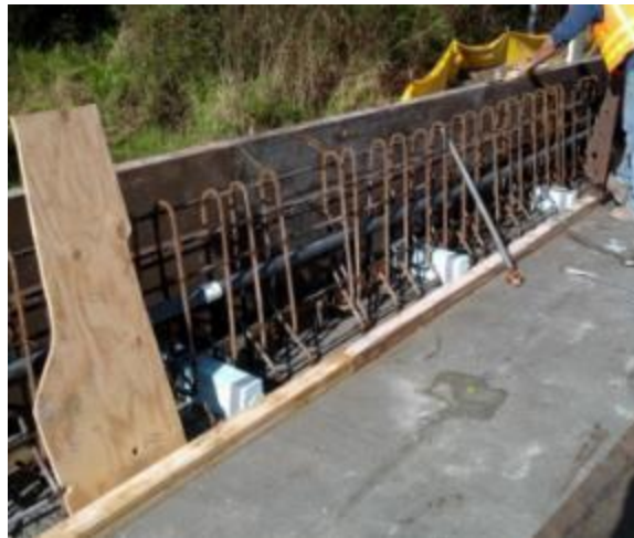
Figure 1.5. Rockridge Road barrier after adding additional reinforcing
