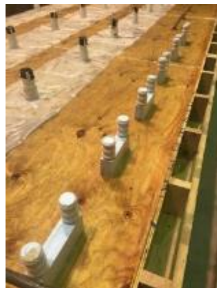
Figure 4.8. Deck block outs to facilitate U-bar installation
