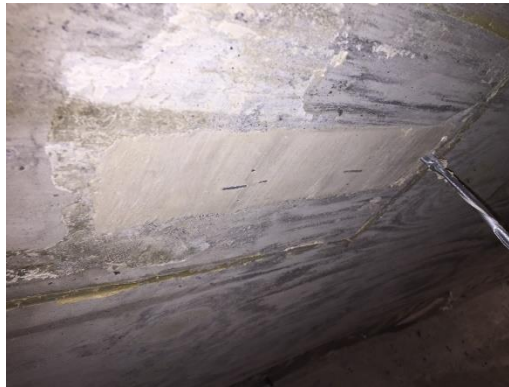
Figure 4.23. Finished U-bar grout pocket
