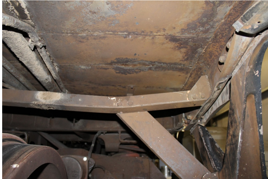
Figure 43. Bent Underframe Member
