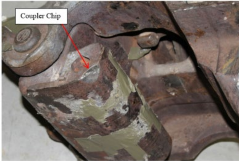
Figure 45. Chipped Locomotive Coupler
