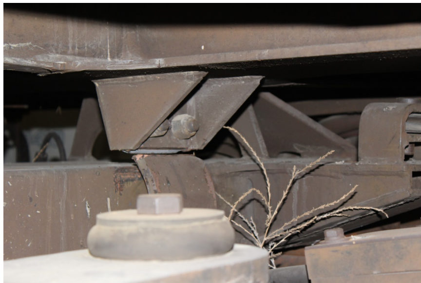
Figure 44. Severed Front Truck Belt Loop
