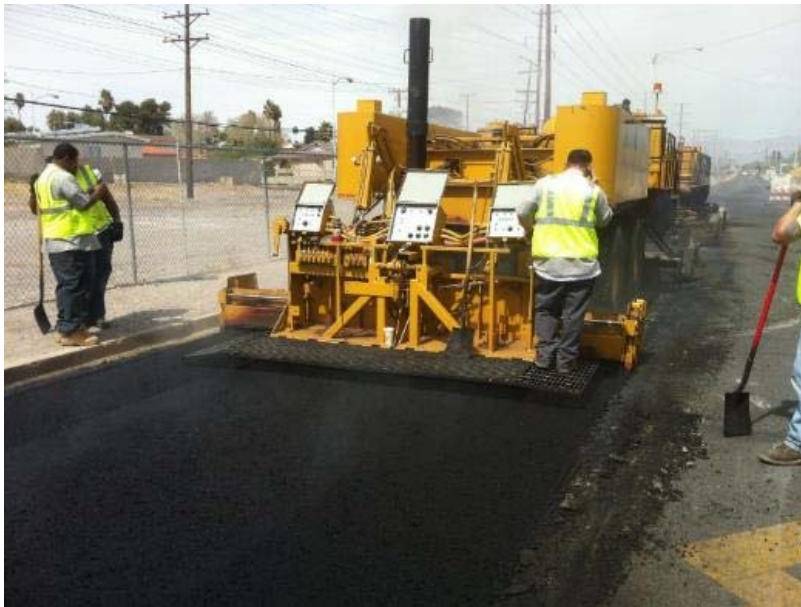
Figure 15. Laydown Screed (photo courtesy of ARRA)
