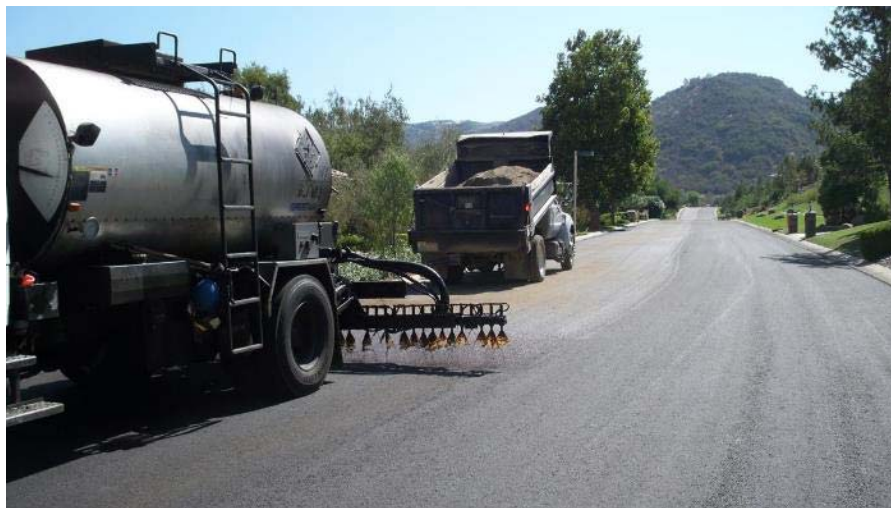
Figure 25. Fog Seal and Sand Treatment over CIR Layer (ARRA, 2015)
