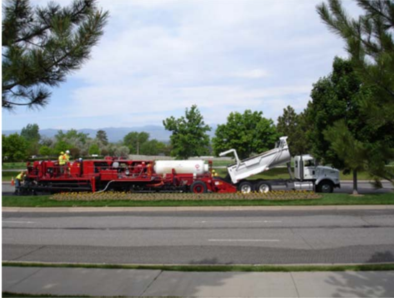
Figure 18. Repaving Process (photo courtesy of ARRA)
