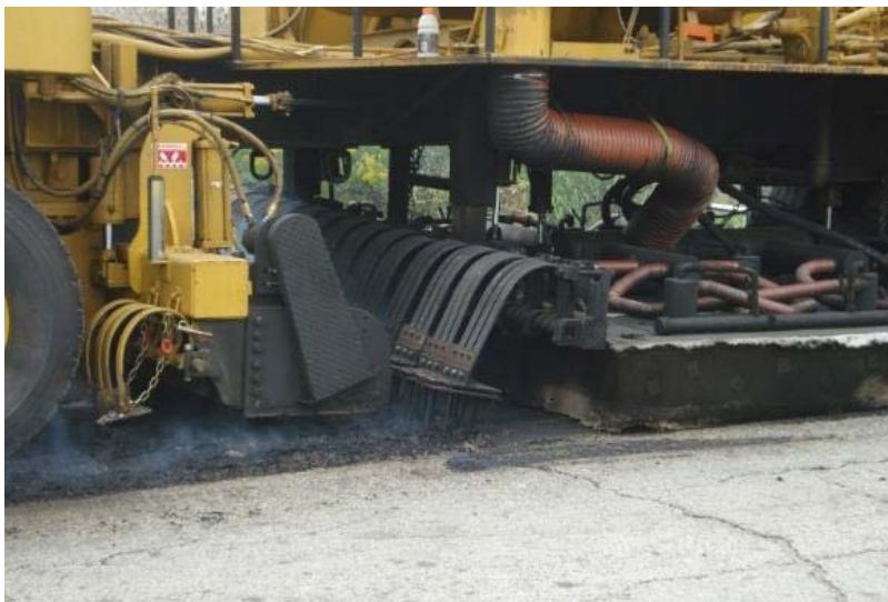
Figure 12. Existing Pavement Loosened by Tines (photo courtesy of ARRA)
