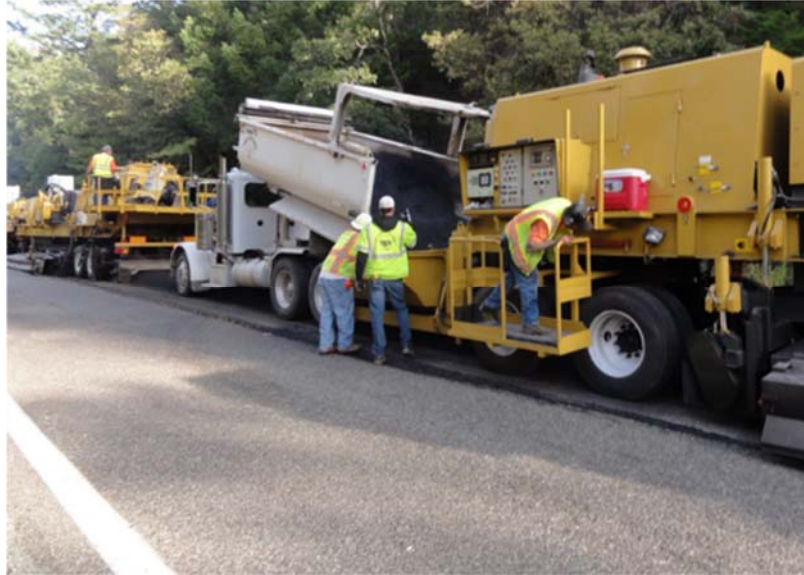
Figure 16. Addition of New Hot Mix (photo courtesy of ARRA)
