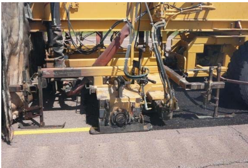
Figure 13. Low Energy Milling Heads (photo courtesy ARRA)
