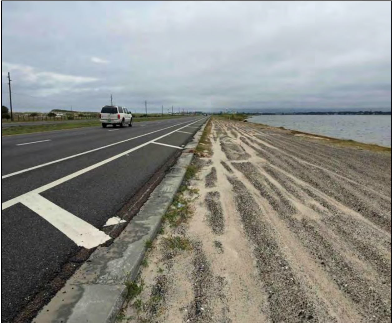
Figure 10.21. Highway shoulder which has been designed to withstand the weir-flow damage during overwashing events (US 98, Okaloosa Island, Florida, 2016)
