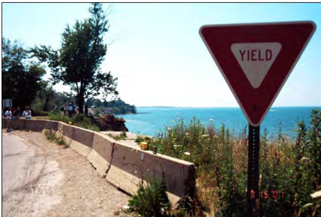
Figure 8.3. A local road being undermined by bluff erosion and long-term shoreline recession on the Great Lakes (Painesville, Ohio, 2001)
