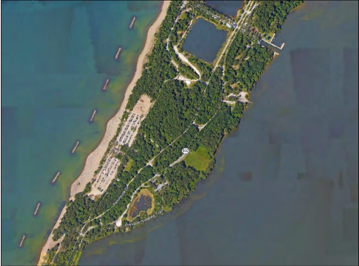
Figure 8.14. Offshore segmented breakwater system at Presque Isle, Pennsylvania
