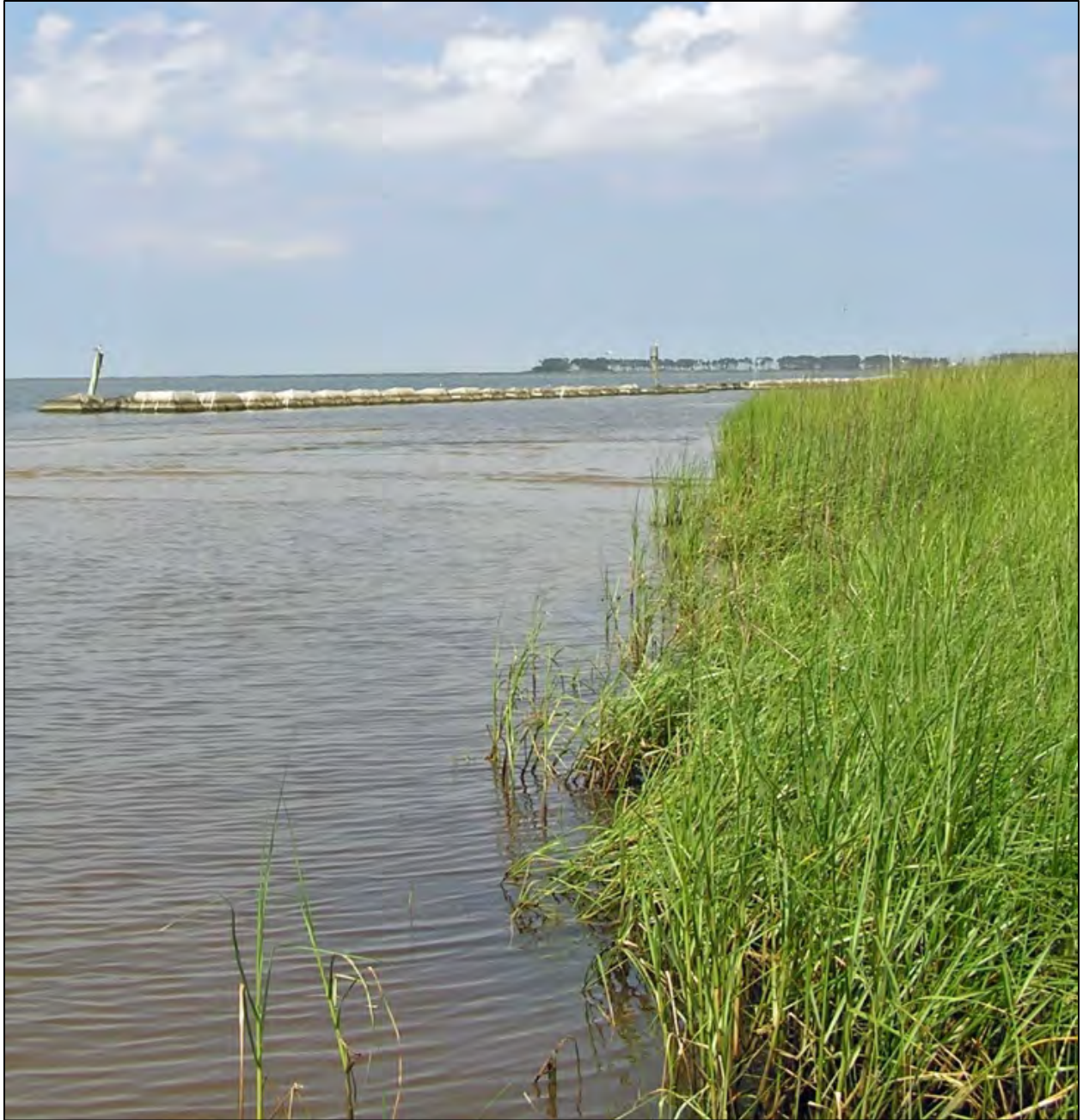
Figure 8.19. Example of a constructed marsh stabilized with a nearshore breakwater (Little Bay, Bayou LaBatre, Alabama)
