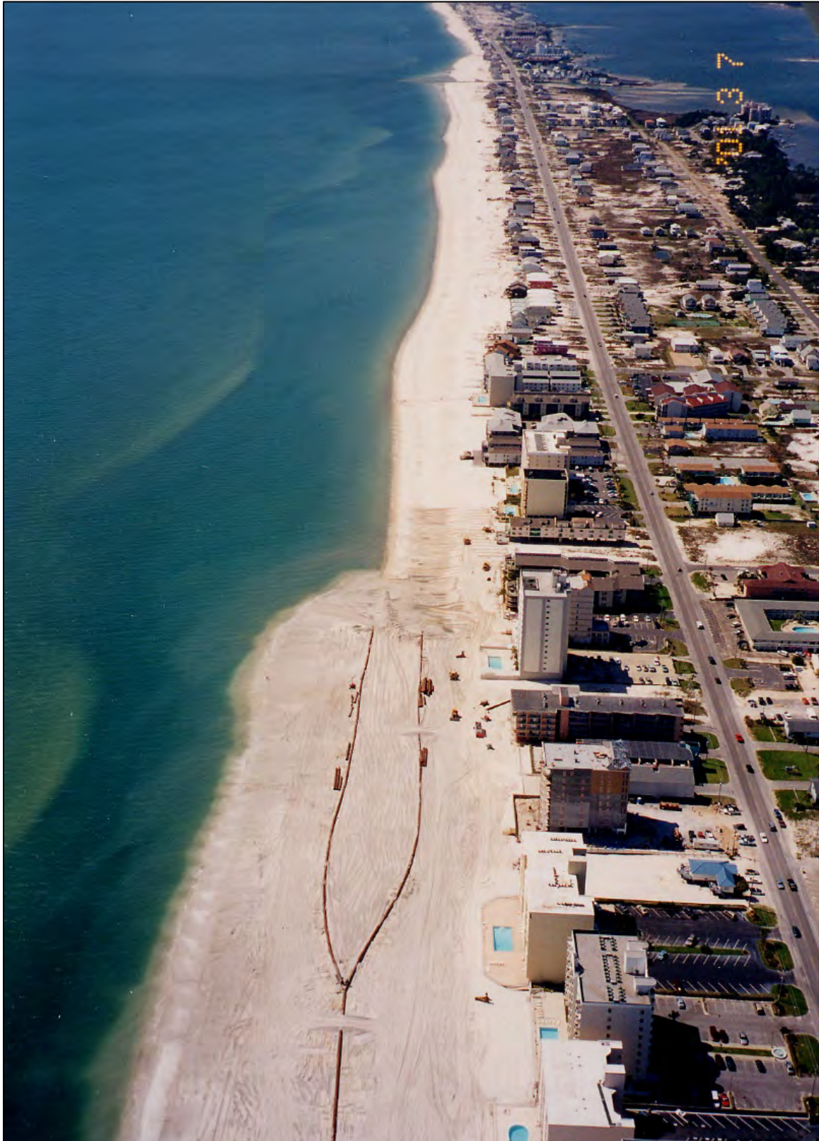
Figure 8.9. A beach nourishment project under construction in Gulf Shores, Alabama (2001)
