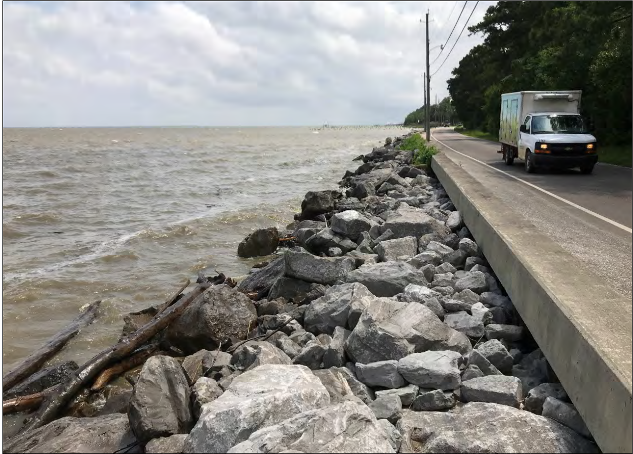
Figure 7.1. A revetment protecting a coastal highway (Bayfront Road, Mobile, Alabama, 2019)
