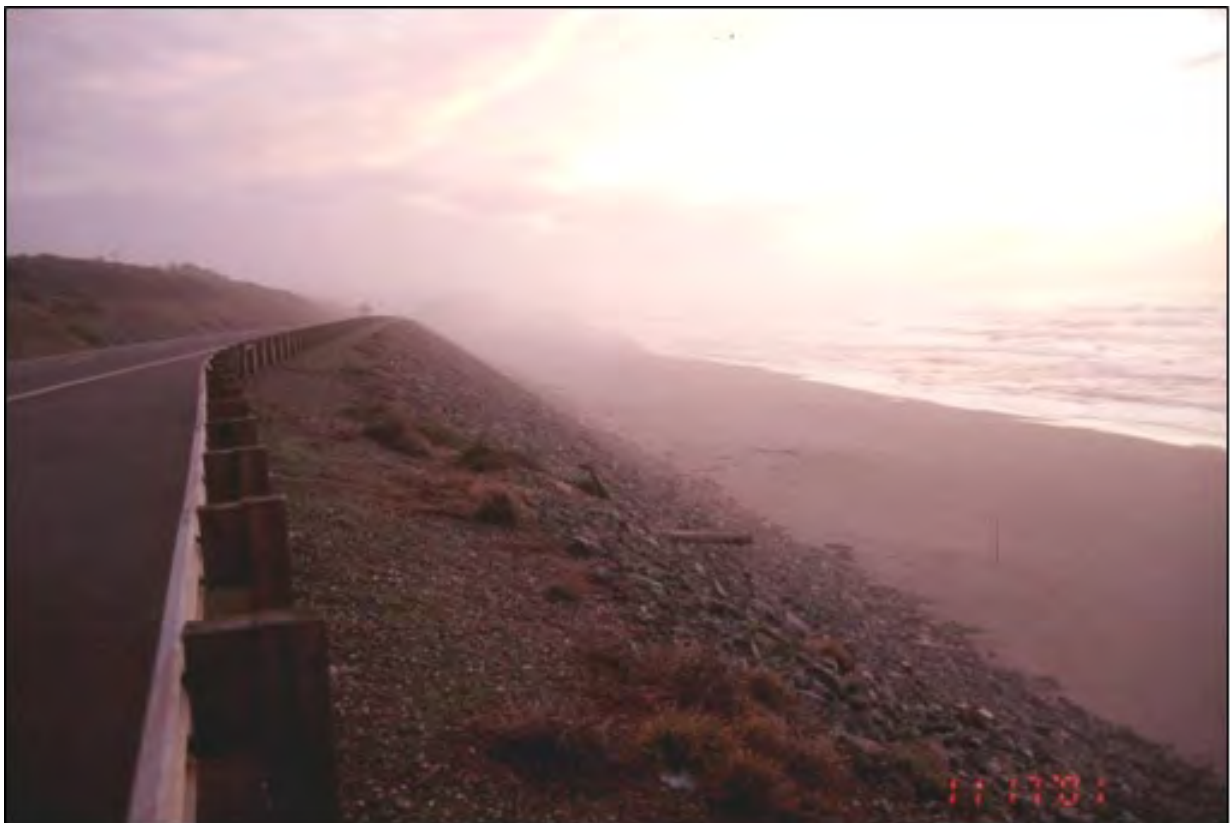
Figure 7.8. Seawall protecting a coastal highway (US 101, Curry County, Oregon, 2001)
