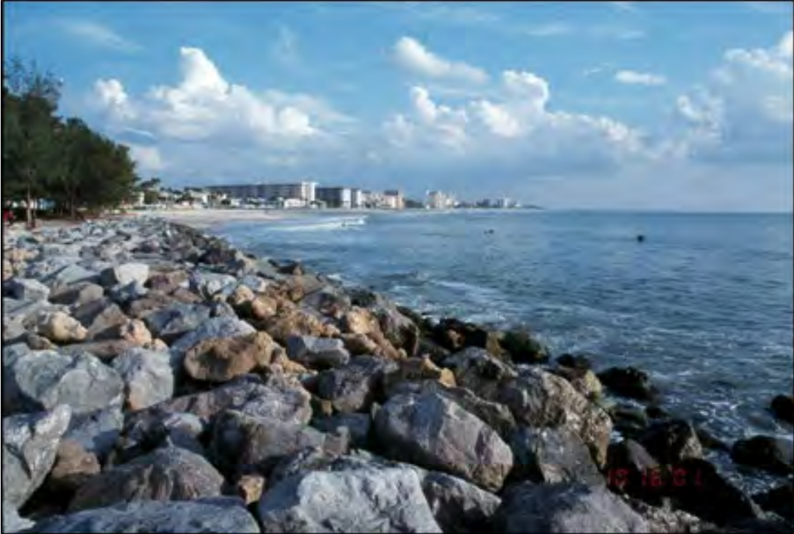
Figure 7.5. Seawall protecting a coastal highway (Venice, Florida, 2001)
