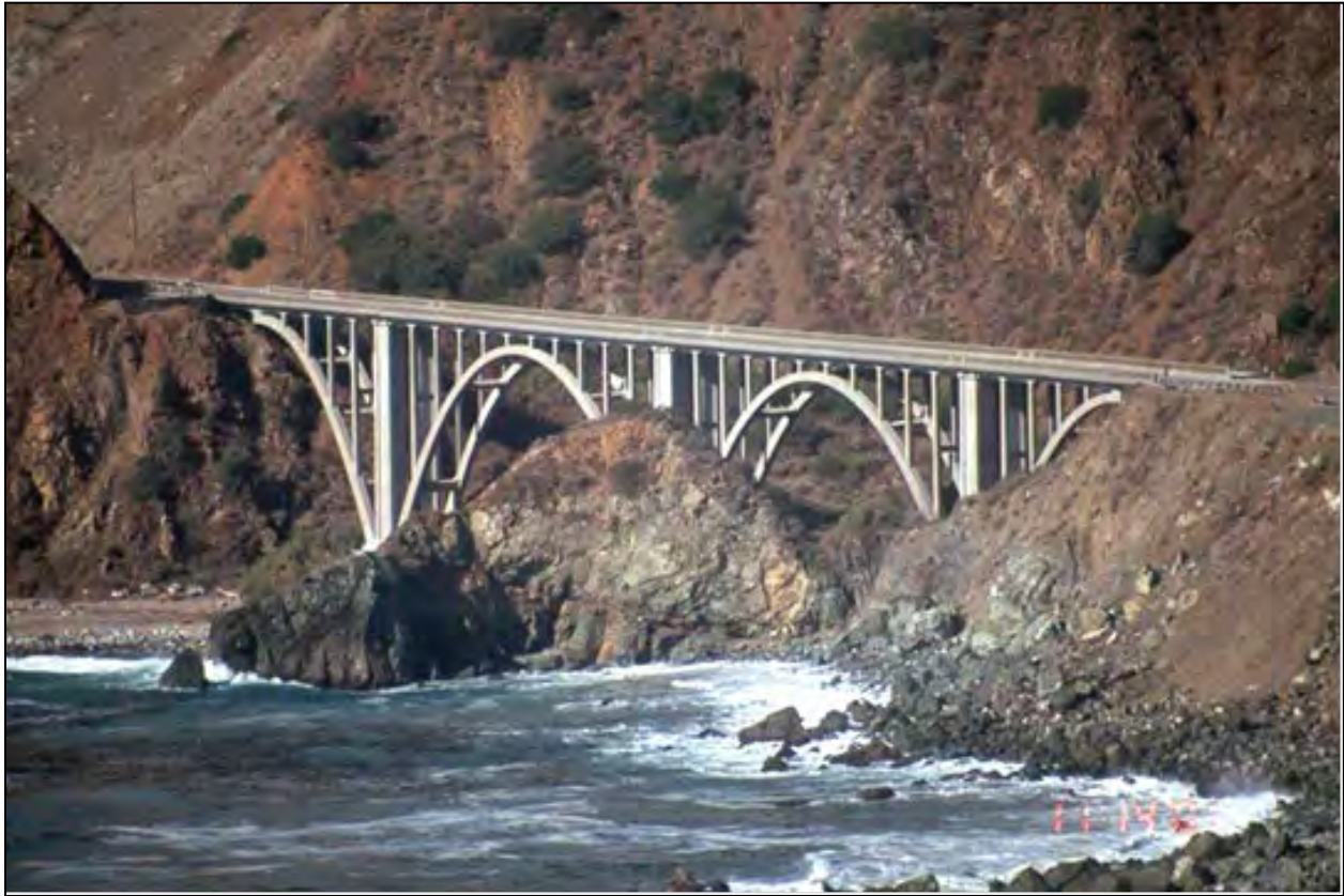
Figure 3.2. Big Creek Bridge on the Pacific Coast Highway (California SH 1)
