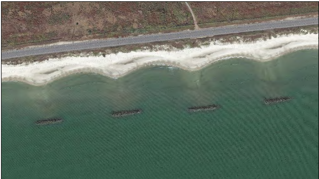
Figure 8.12. Offshore segmented breakwaters with salients in beach nourishment protecting a highway (Louisiana SH 82, Holly Beach)
