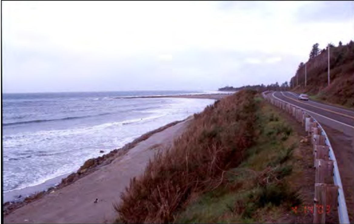
Figure 8.1. A highway initially built inland now threatened by long-term shoreline erosion. Cape Shoalwater area of Washington SH 105 (2003)
