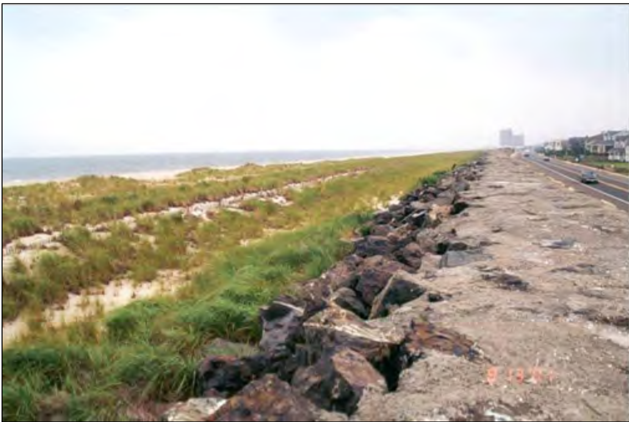
Figure 8.11. Beach nourishment seaward of a seawall protecting a road. (New Jersey SH 35, Sea Bright, 2001)
