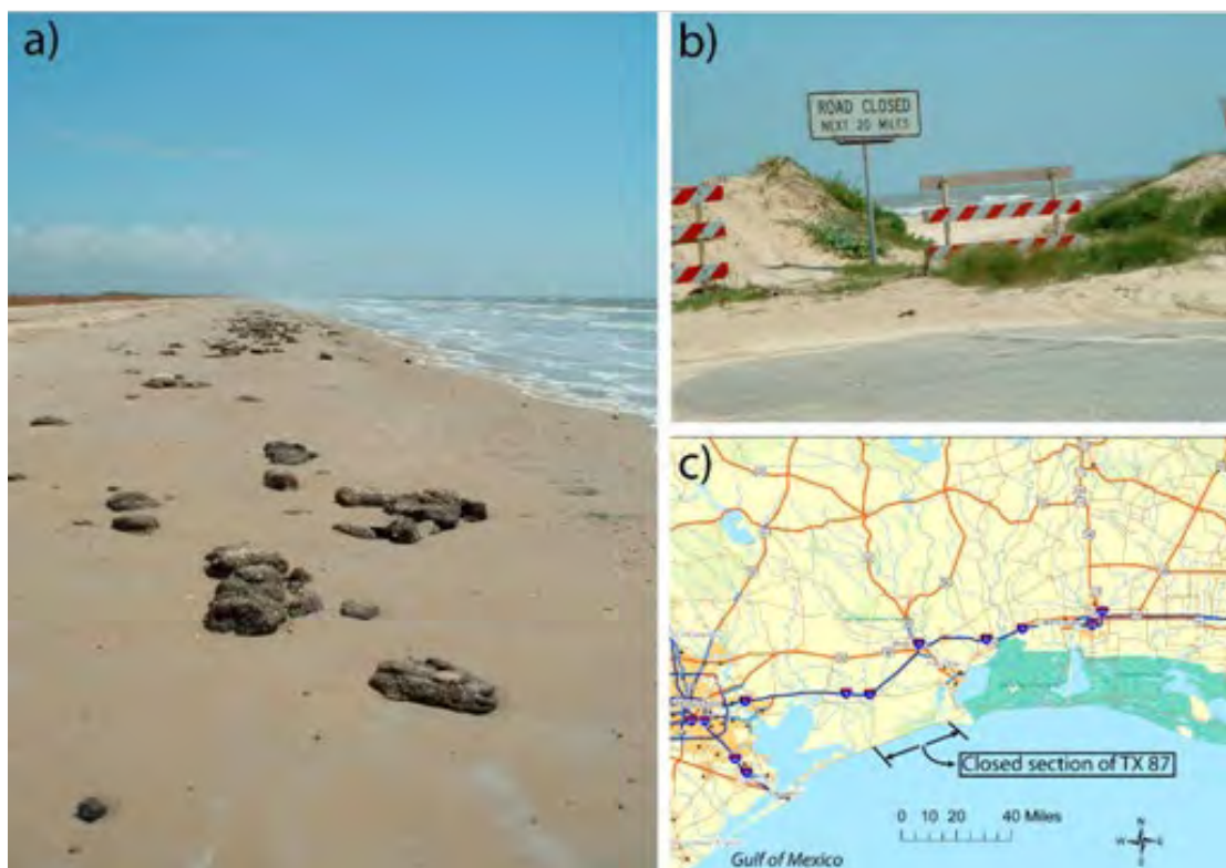
Figure 8.4. Road destroyed by shoreline recession: a) broken pavement on the beach at the old location; b) south end of the closed section; c) location map. (Texas SH 87, Jefferson County, circa 2002)
