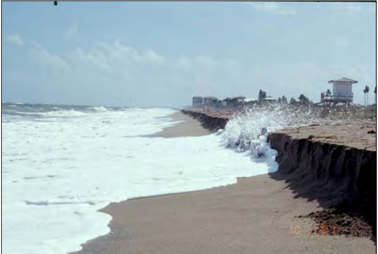
Figure 6.7. A beach scarp (Los Angeles County, California)
