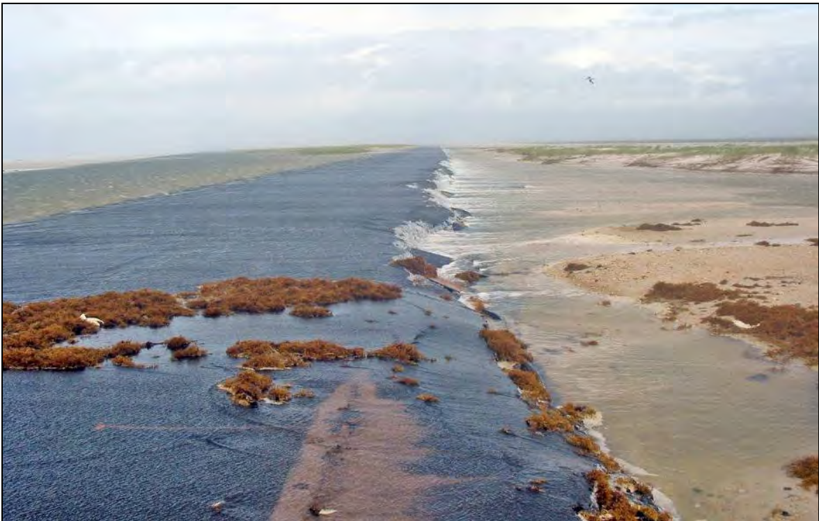
Figure 10.7. Weir-flow damage occurring. (Fort Pickens Road, Gulf Islands National Seashore, Florida, July 2005; FHWA photograph)
