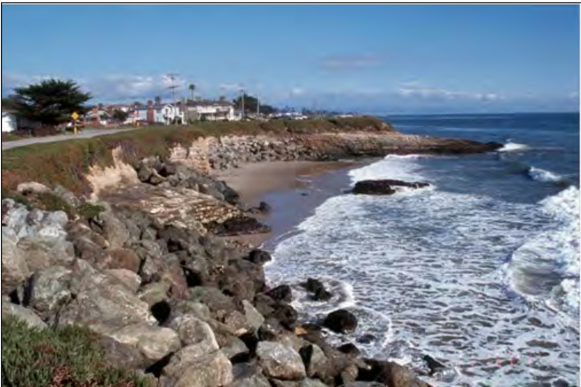
Figure 7.12. Seawall protecting a local road (West Cliff Drive, Santa Cruz, California, 2001)
