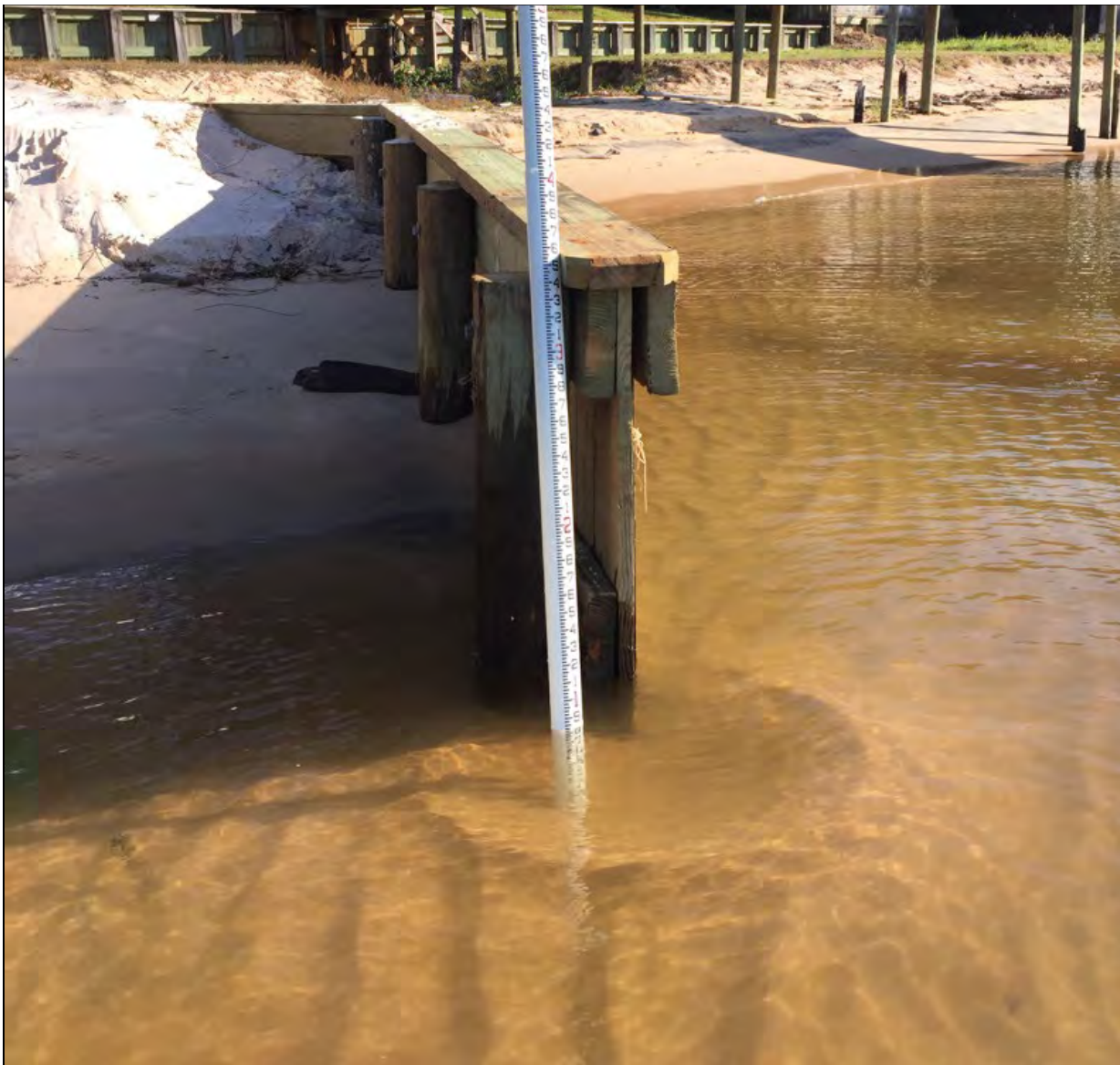
Figure 12.10. Local scour depression at the terminus of a coastal structure
