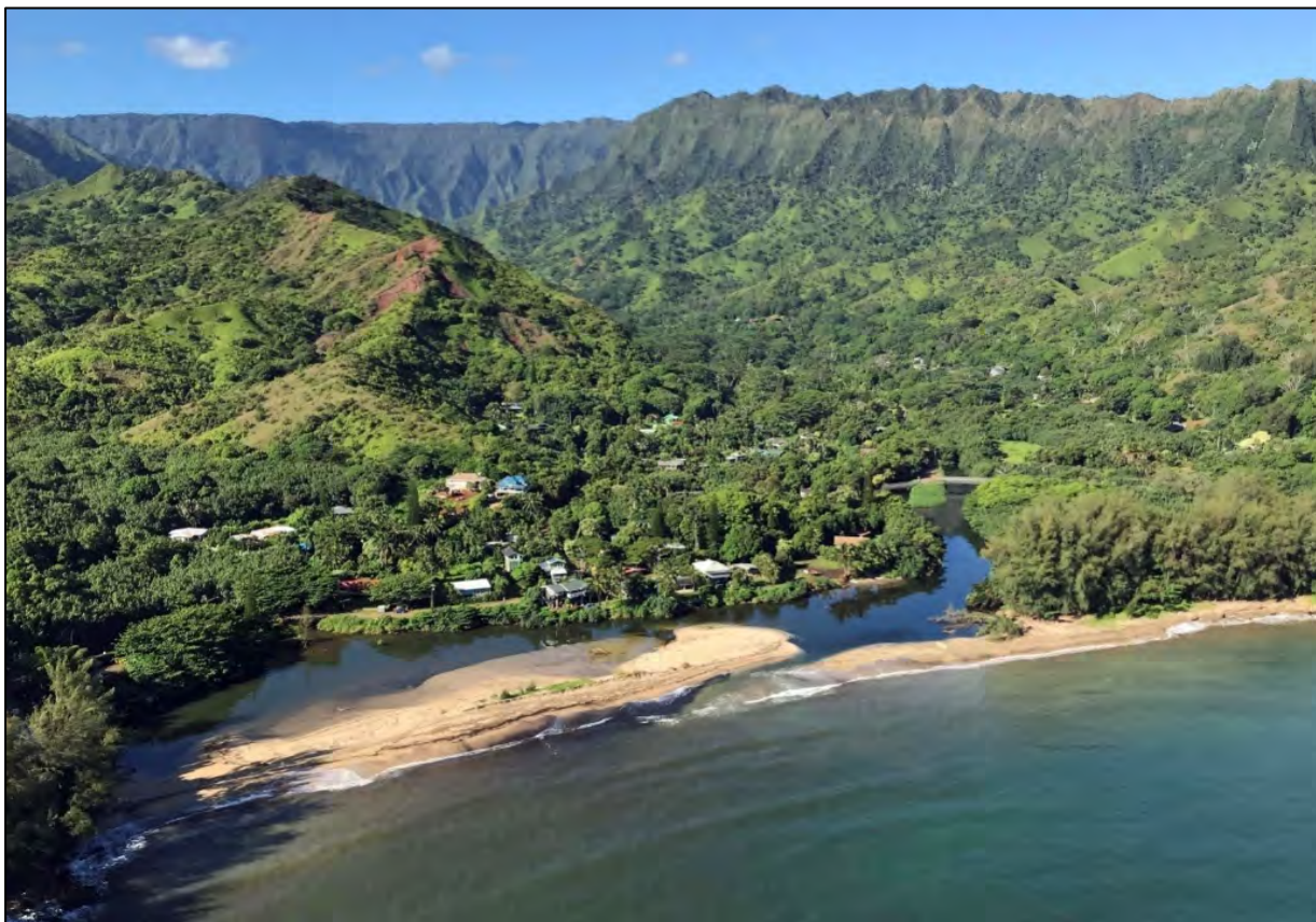
Figure 14.7. Wainiha River, on the north shore of the island of Kauai, Hawaii, is an area with an extremely high tsunami hazard and a history of tsunami-induced bridge damage
