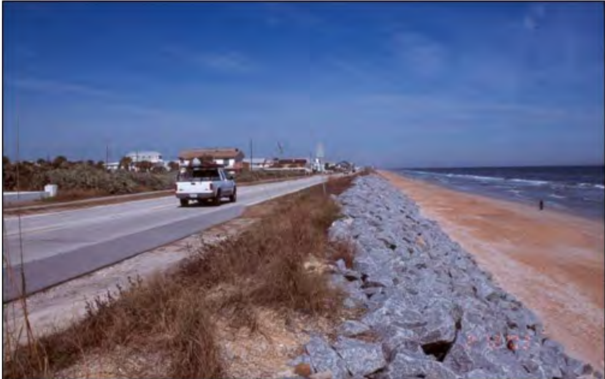
Figure 7.7. Seawall protecting a coastal highway (Florida SH A1A, Flagler Beach, 2002)
