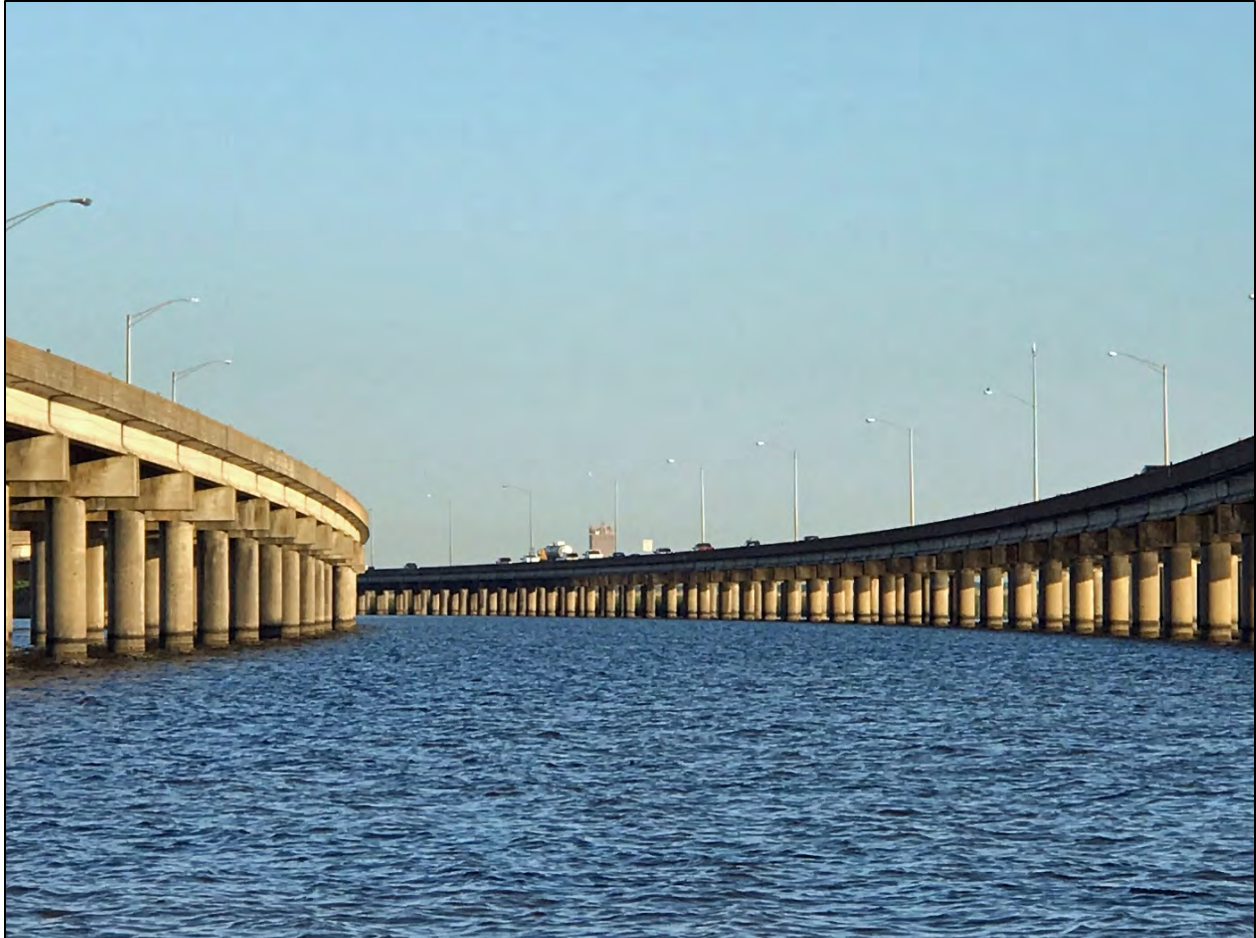
Figure 11.4. Interstate 10 bridge crossing Mobile Bay, Alabama
