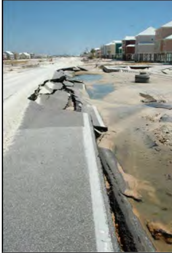
Figure 10.14. Evidence of weir-flow damage to the seaward edge of pavement due to return flow late in the storm (Alabama SH 182, after Hurricane Ivan, Gulf Shores, 2004)
