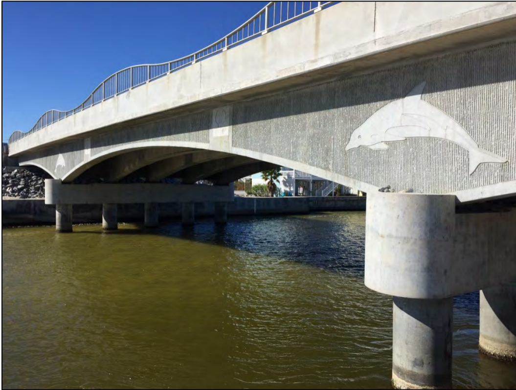
Figure 11.2. Bridge spanning a small inlet (Alabama SH 182 in Gulf Shores)
