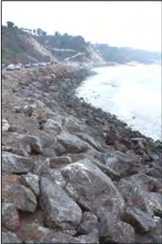
Figure 7.6. Seawall protecting a coastal highway (Pacific Coast Highway, Pacific Palisades, California, 2003)
