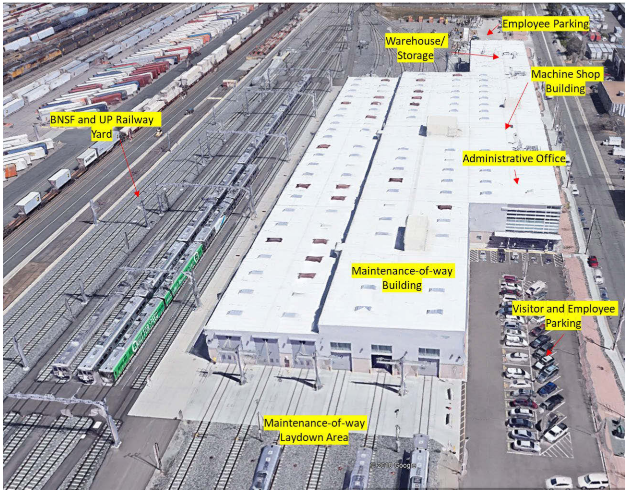
Figure 23: Bird's Eye view of the RTD Commuter Rail Maintenance Facility (by Google Earth) from the South Side
