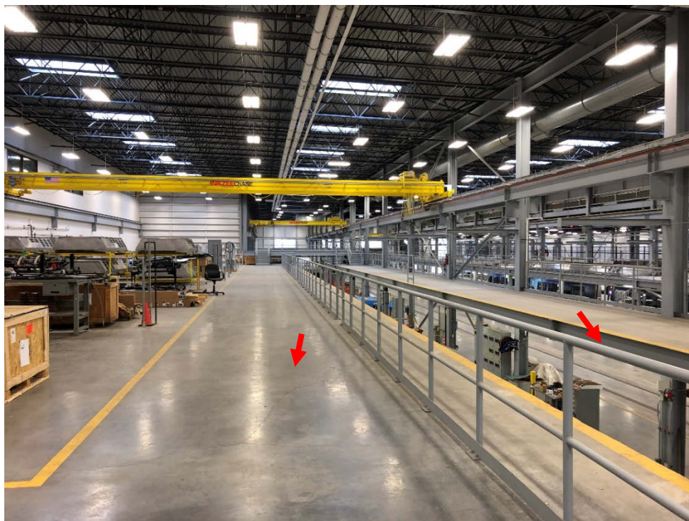
Figure 33: Single-level mezzanine area with two 3-ton overhead cranes
