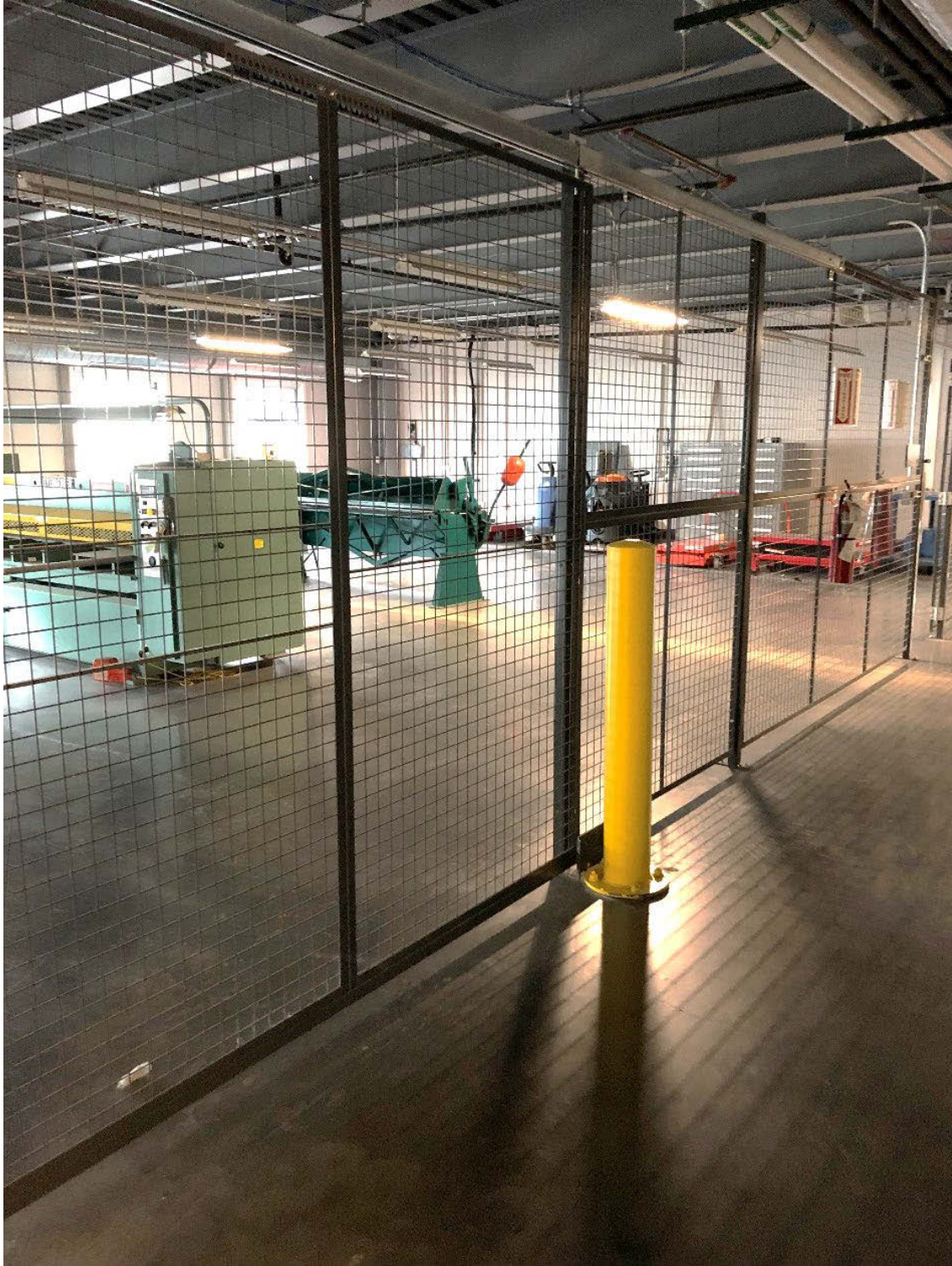
Figure 30: Machine shop and the second-floor structural system – Eastern wing of the building
