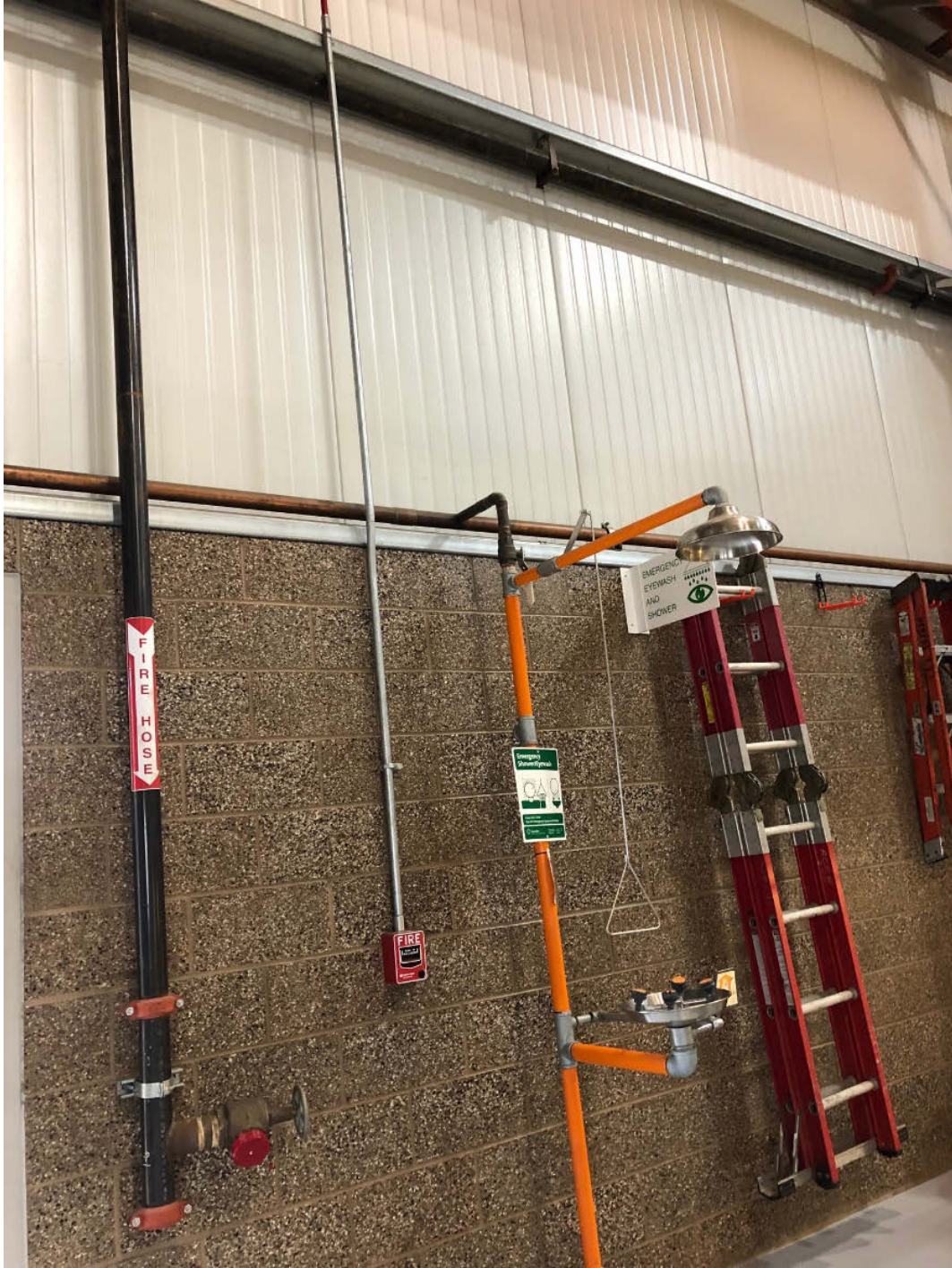
Figure 18: Building components: perimeter CMU walls and composite sidings
