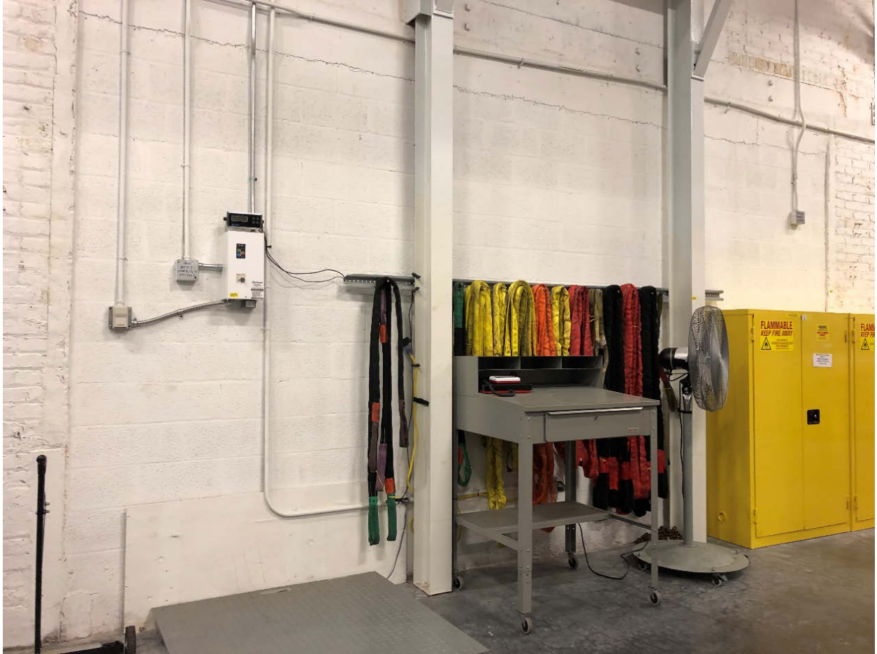
Figure 48: Materials storage building's steel framings and the perimeter masonry walls
