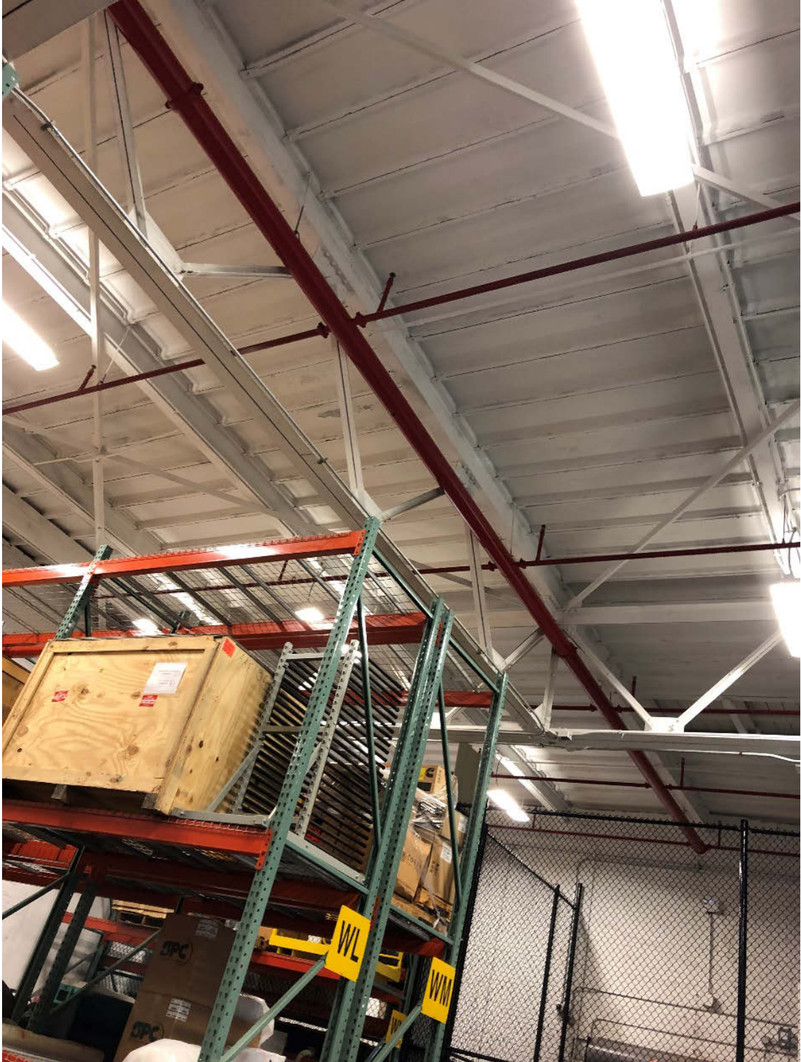
Figure 49: Two-way truss-joints supporting roof steel beams – Materials storage building
