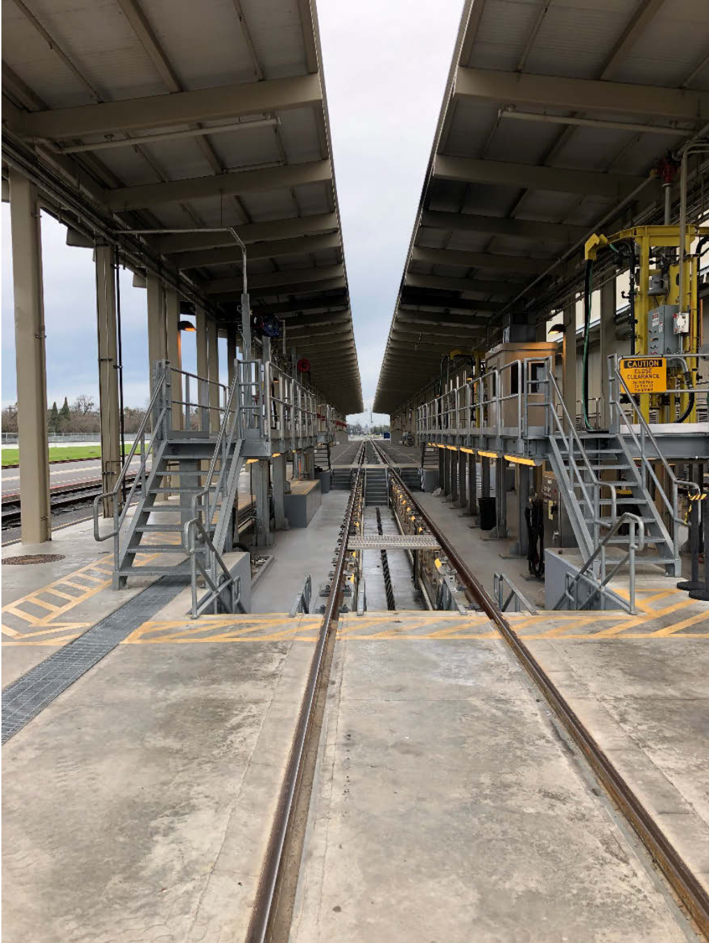
Figure 20: Steel structural framing and maintenance pit for the outdoor facility structure
