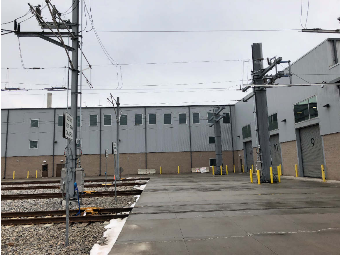
Figure 29: The building enclosure comprising CMU walls and corrugated metal sidings
