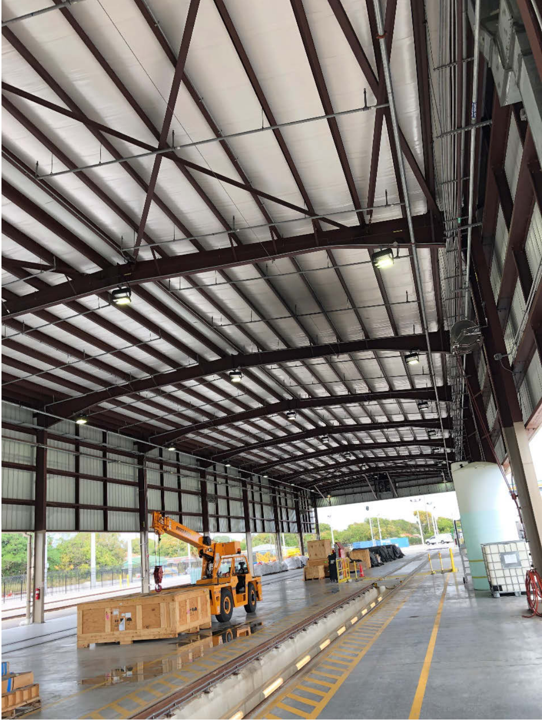
Figure 43: Building structural components: steel portal frame and horizontal steel bracing, and open perimeter
