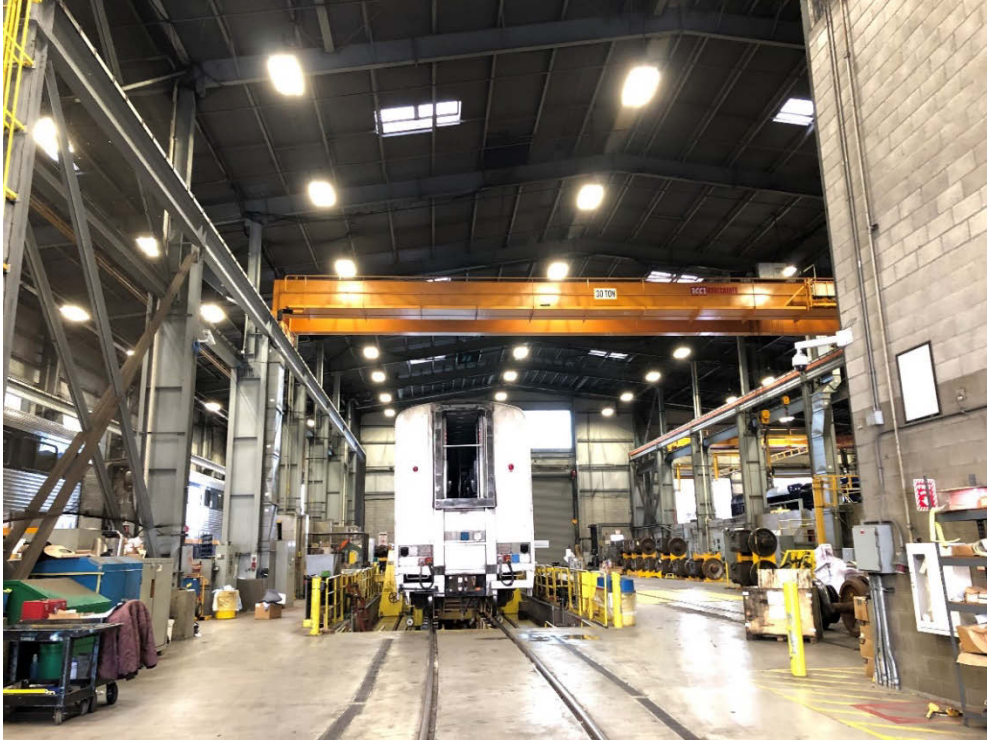
Figure 10: Building structural components, roof framings and overhead crane system
