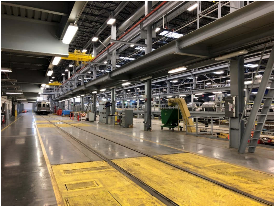
Figure 27: Building's structural components: steel columns and beams and cantilevered mezzanine levels
