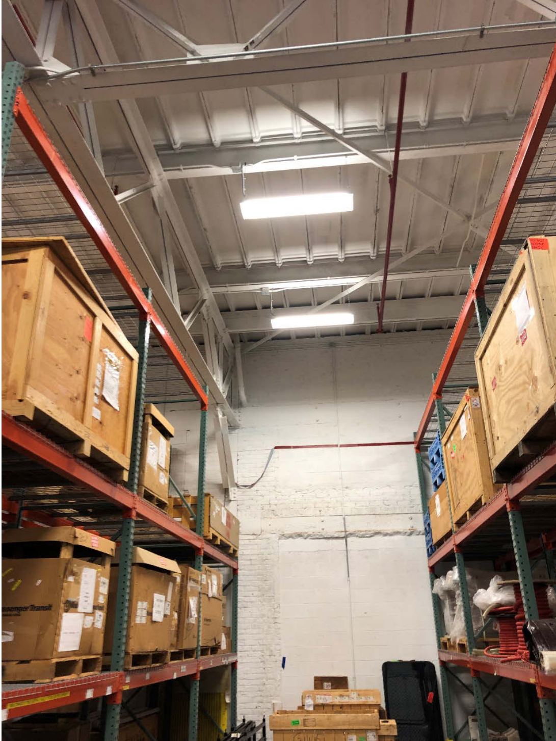
Figure 47: Materials storage building's walls and roof system
