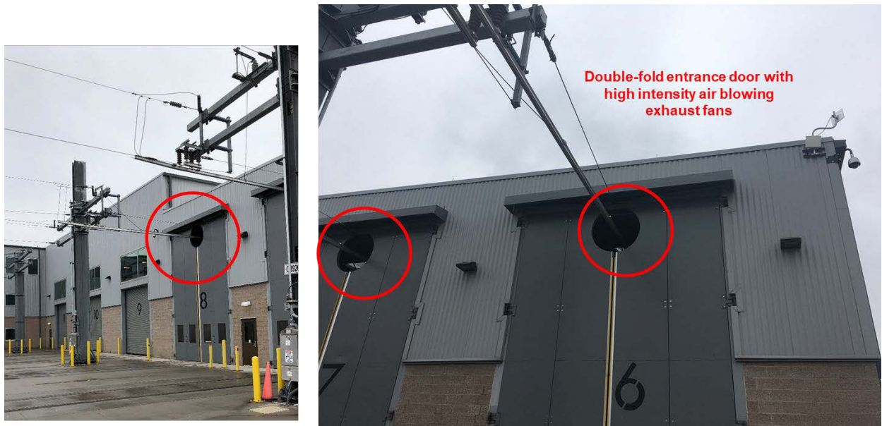
Figure 38: Double-fold entrance door with high intensity air blowing exhaust fans
