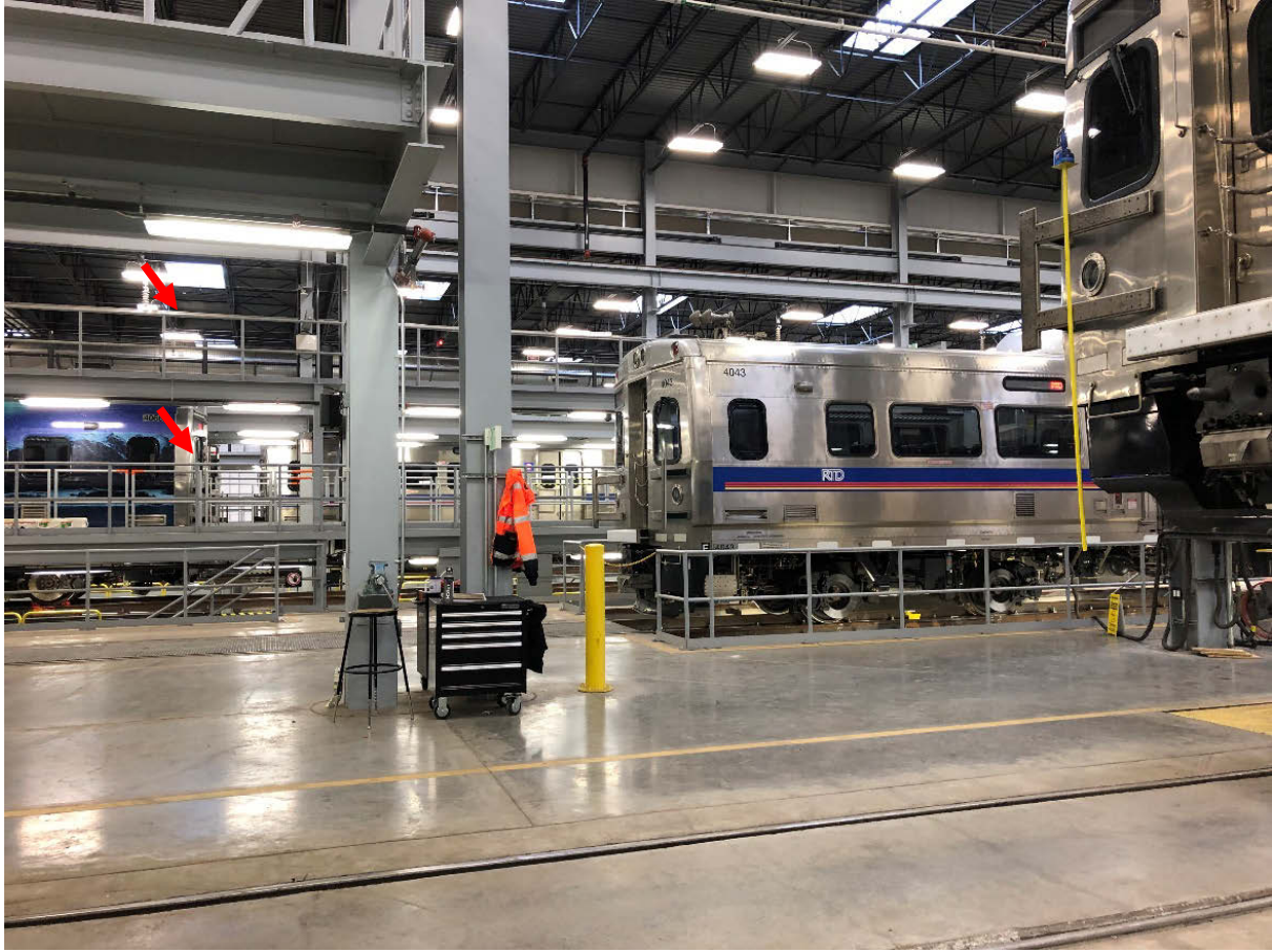
Figure 34: Two-level mezzanine floors next to a drop pit for easing access during maintenance and increasing efficiency
