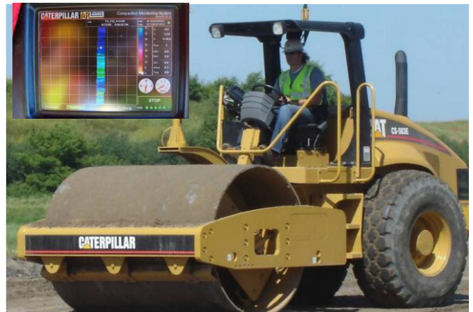
Intelligent compaction technologies improve road and subgrade densities.
