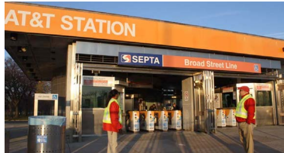
Southeastern Pennsylvania Transportation Authority AT&T Station, Philadelphia, PA.
