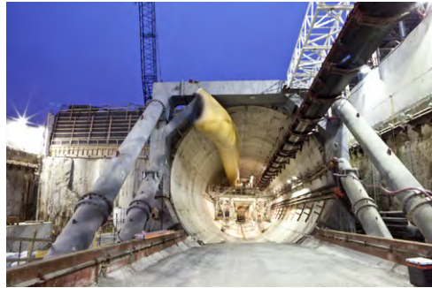
Port of Miami Tunnel Entry.
