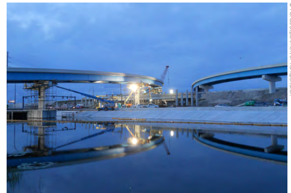
Interstate 595 Raising Ramp.
