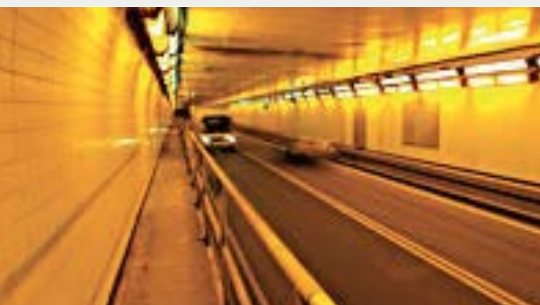
Norfolk/Portsmouth Midtown Tunnel, Virginia.
