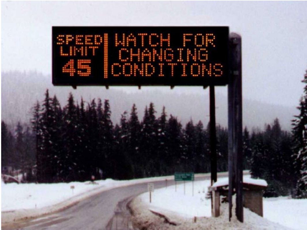
Figure 37. Photo. Example of variable speed limit sign with additional variable message sign for warning drivers of weather-related road conditions in Washington. (229)
