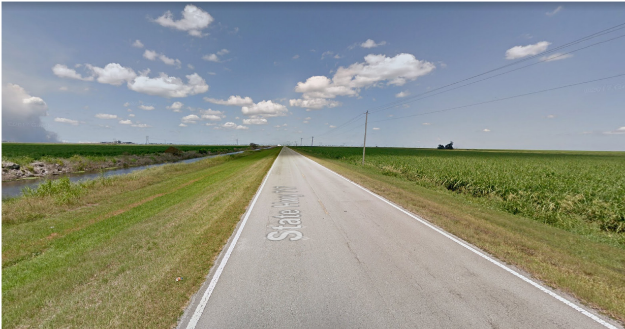
Typical view of CR-717. Image Courtesy of Google Street View, accessed 10/29/2018
