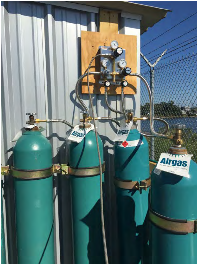
Figure 3-11 Four-Cylinder Bracket System
