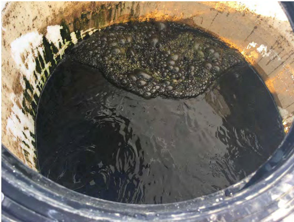
Figure 4-2 View of Algae in Decant Tank on October 4, 2017
