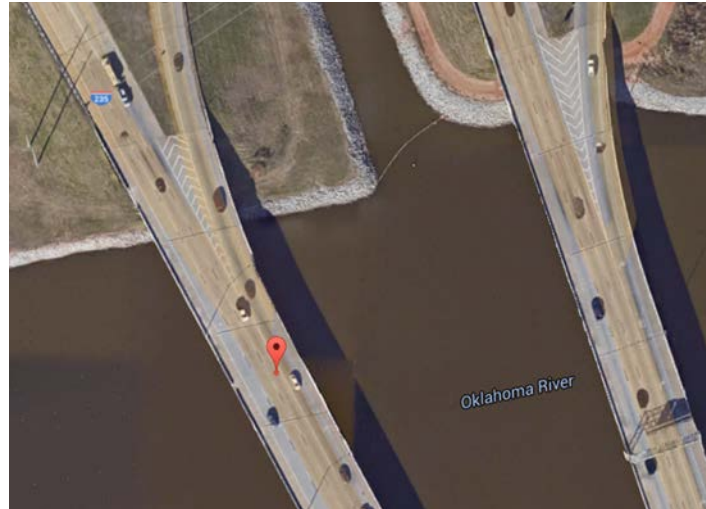
Figure 5-12 Close View of Segment 44 I-35 Intersect with The Centennial Express Way HW 235.
