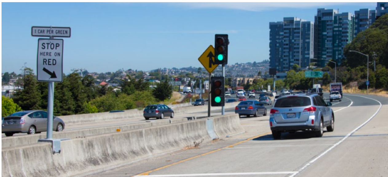
Figure 2. Typical Single Lane Metered On-Ramp on I-80 SMART Corridor (Low, 2017)
