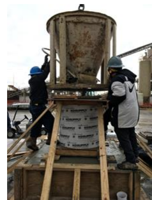
(c) Drilled shaft and base casting
