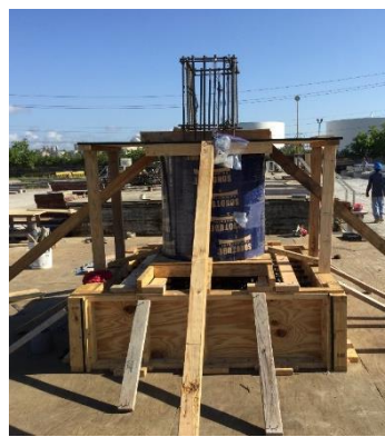
(b) Drilled shaft and base formwork
