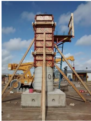
(g) Column formwork
