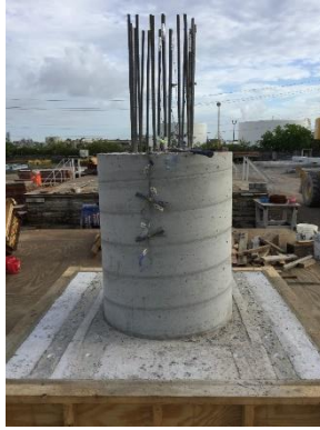
(e) Drilled shaft and base- after casting
