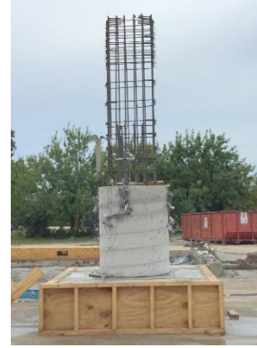
(f) Placement of column bars
