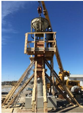
(h) Column casting
