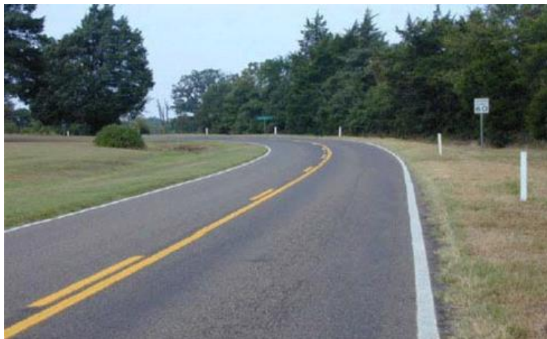
Figure 37. Presence of Delineators.
