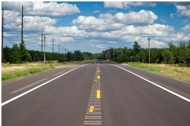
Figure 35. Centerline and Shoulder Rumble Strips.
