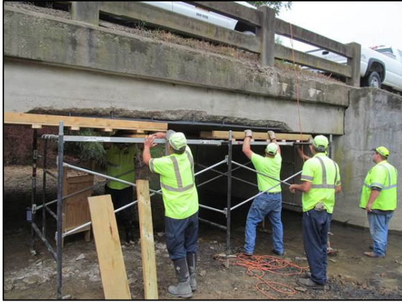
(a) Setup formwork
