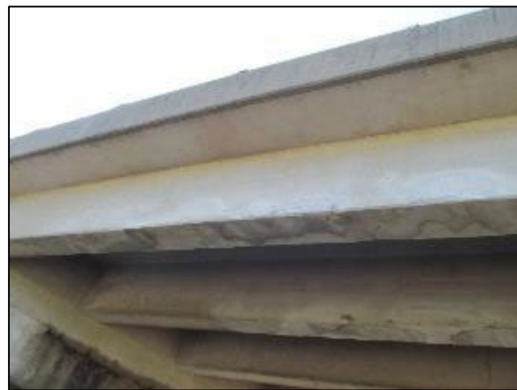
(d) Bridge girder with applied repair mortar
