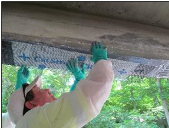
(a) CRP 070 applied with epoxy
