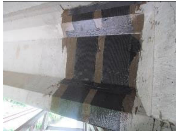
(b) TCF application over CRP
