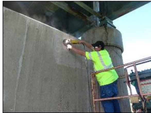
(b) Surface preparation for CatStrong UCF 115
