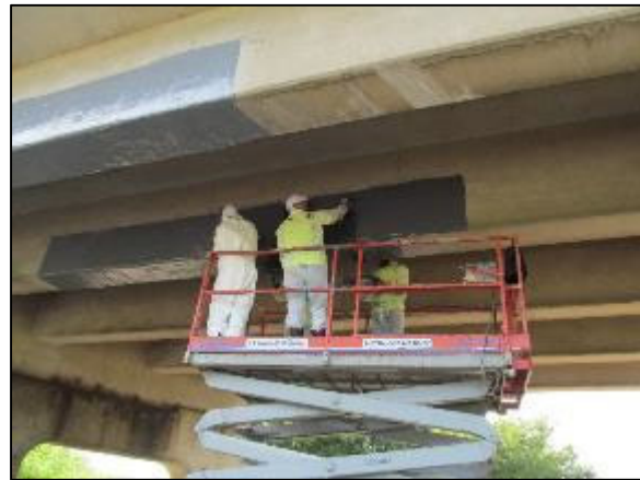
(b) TCF application over CRP
