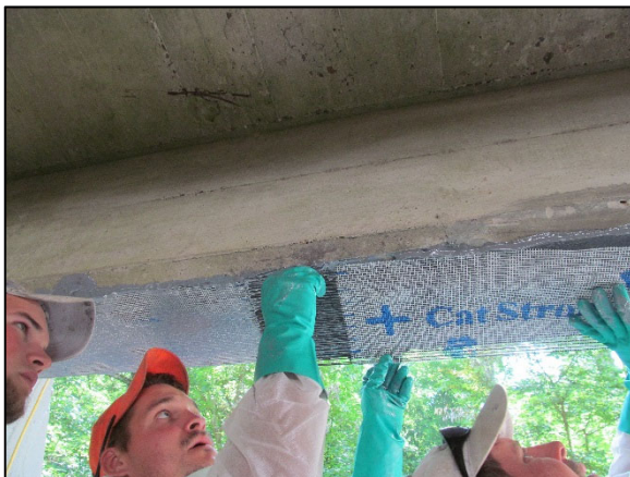
(c) Alignment of plus to minus to facilitate mesh
