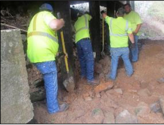
(a) Clearing area around base of timber piles
