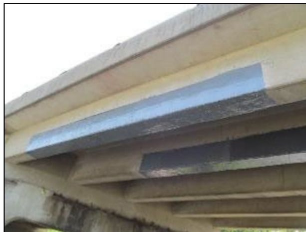
Fig. 23. Completed repairs on KY 80 over I-69 with UV protective coating
