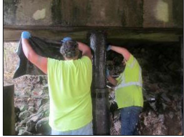
(b) Wrapping TCF 012 around timber pile
