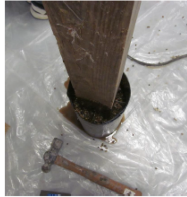
Apply epoxy mortar in layers
