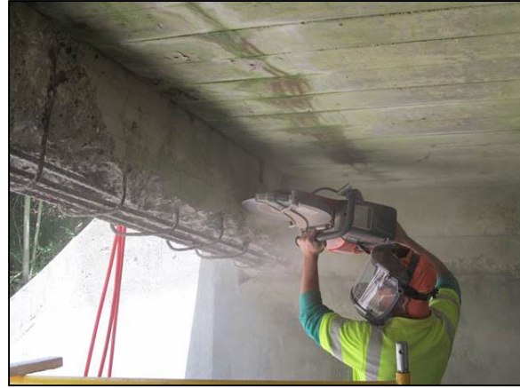
(b) Saw cuts to create simple geometric shapes
