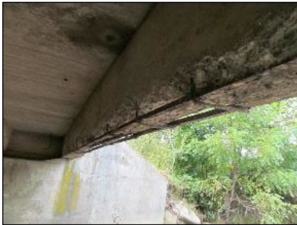
(a) Concrete removed to expose rebar
