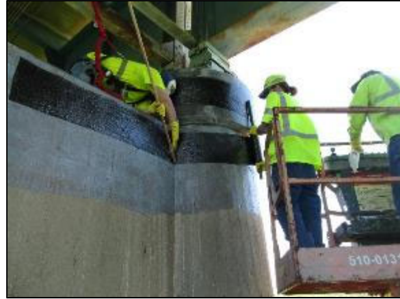
(b) UCF 115 application onto pier wall
