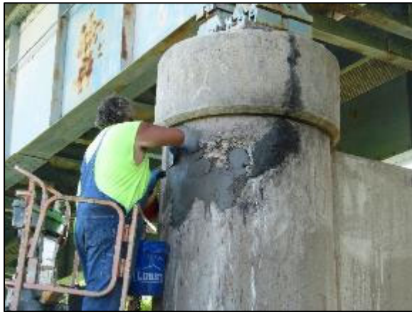
(a) Repair mortar application
