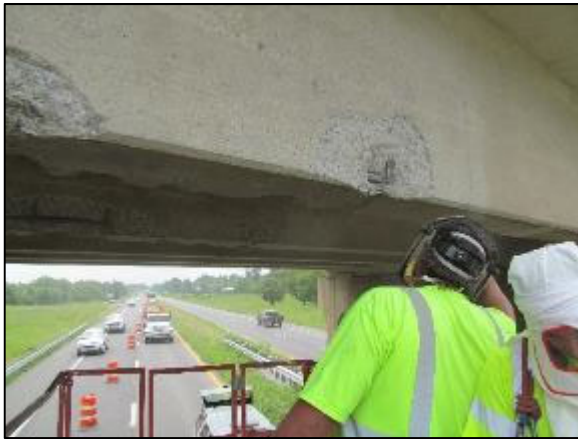
(a) Concrete removed to expose rebar
