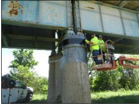
(a) Wrapping UCF 115 around column
