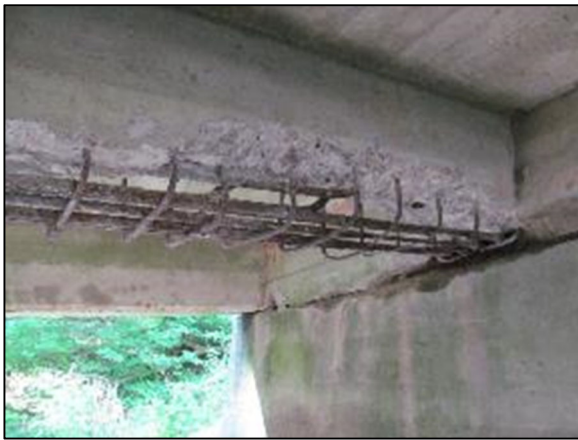
(a) Concrete removed to expose rebar
