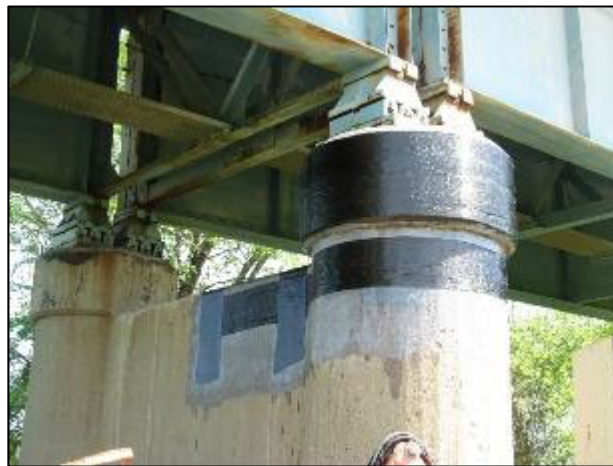
Fig. 38. Completed repairs to US 60 over Cumberland River bridge pier
