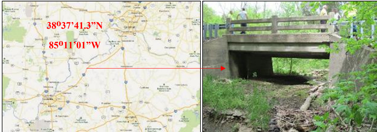
Fig. 3. Location of KY 55 over Majors Run Creek in Carrol County, Kentucky
