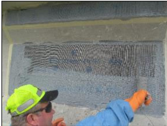
(a) Modular CRP application process
