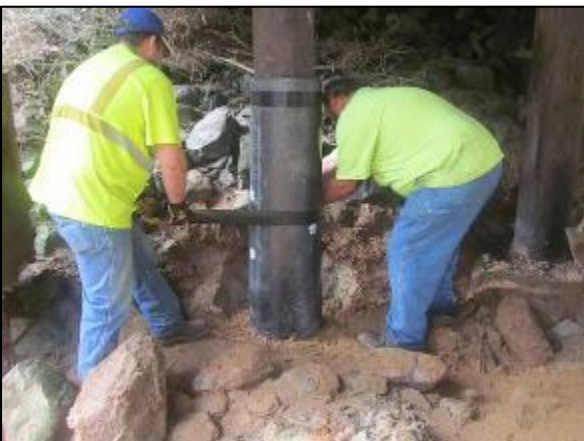
(c) Wrapping TCW 012 around spacers
