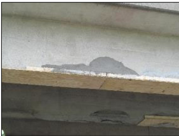
(c) Wood formwork and repair mortar application
