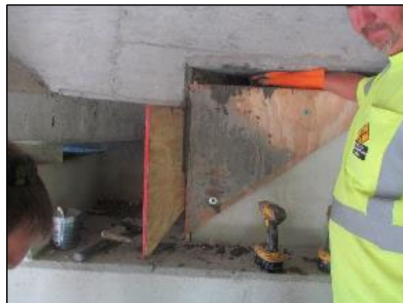
(b) Wood formwork and repair mortar application
