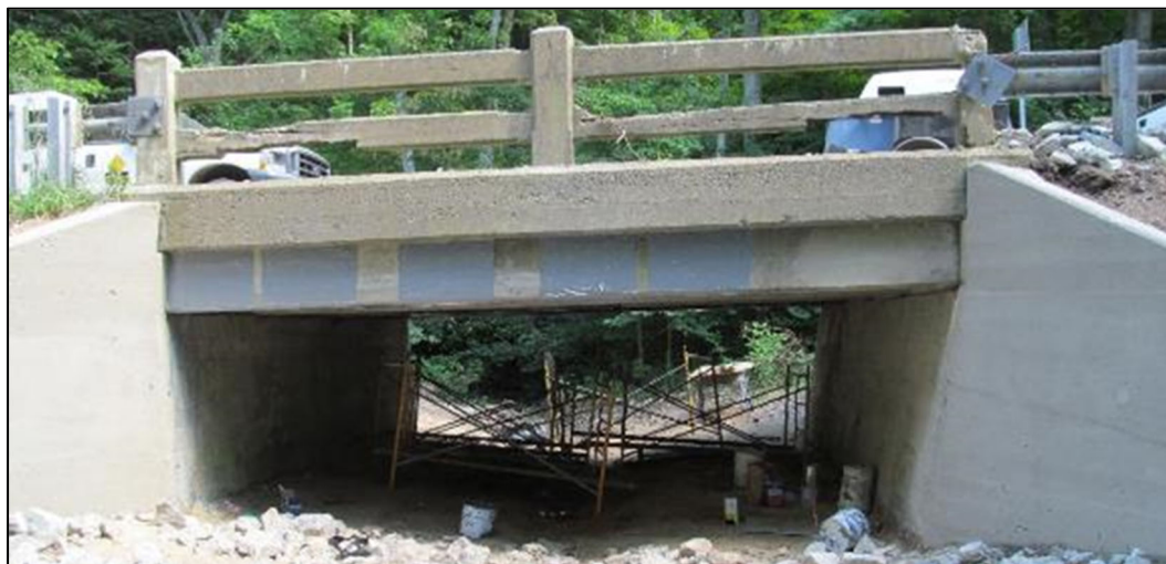
Fig. 9. Repairs complete on KY 55 over Majors Run Creek
