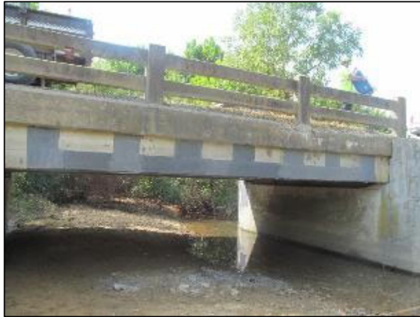
Fig. 16. Completed repairs on KY11 over Cat Creek
