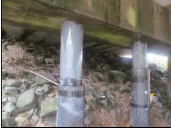
(a) Coating timber pile in primer epoxy
