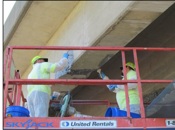
(b) Application of bonding agent
