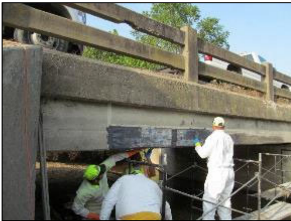
(a) CRP 070 applied with epoxy
