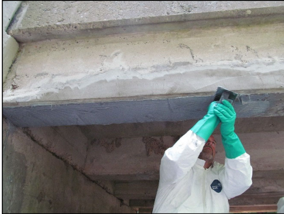
(a) Applying coat of epoxy to concrete surface
