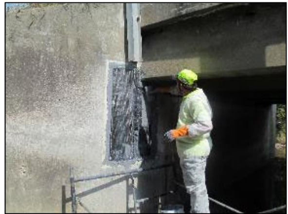
(b) TCF application over abutment crack
