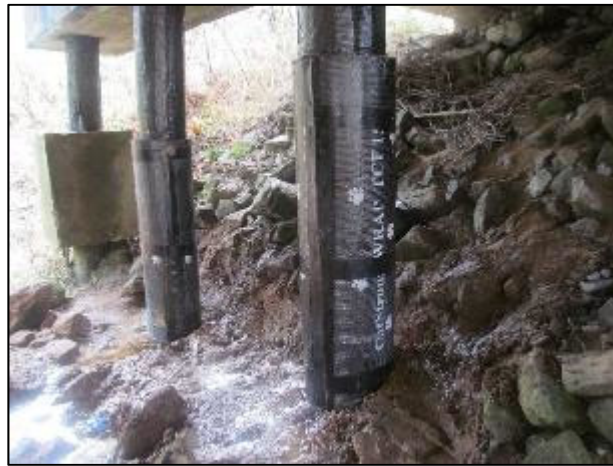
Fig. 44. Completed retrofit of KY 339 over Massac Creek timber piles
