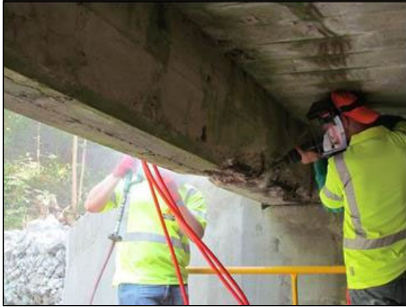
(a) Removing loose concrete
