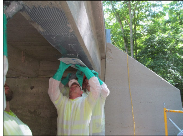
(b) Placing CatStrong over epoxy layer
