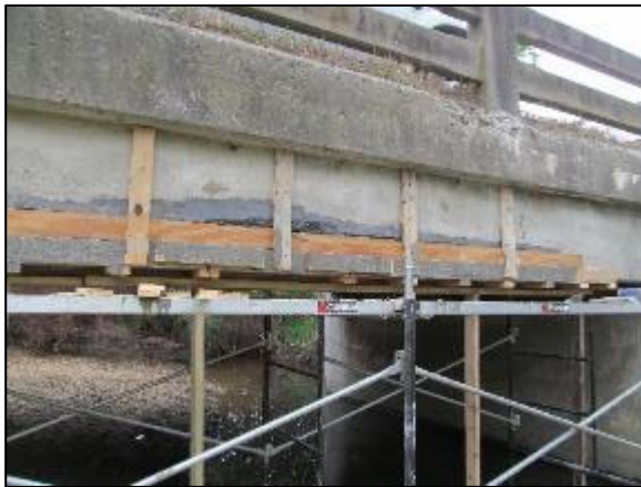
(c) Wood formwork and repair mortar application
