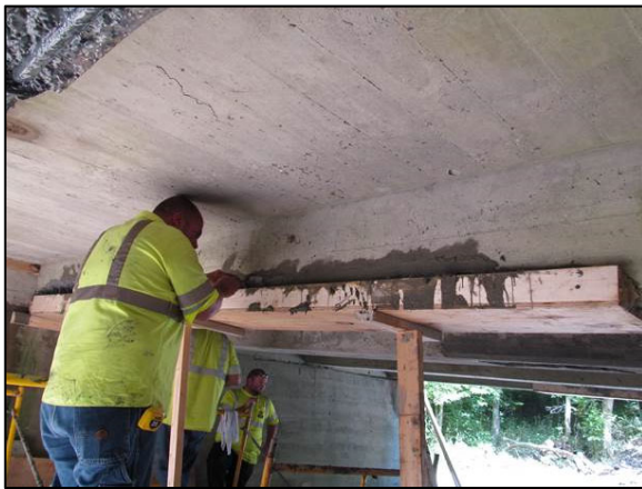
(c) Application of repair mortar
