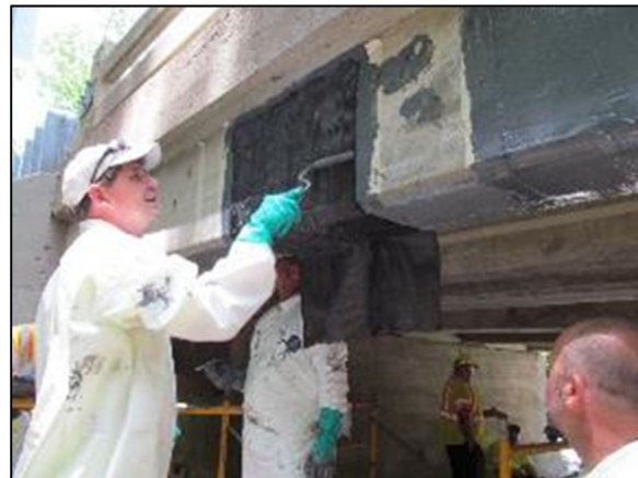
(b) TCF application with laminating rollers
