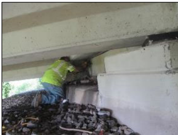
(a) Cleaning damaged areas of PC beam ends
