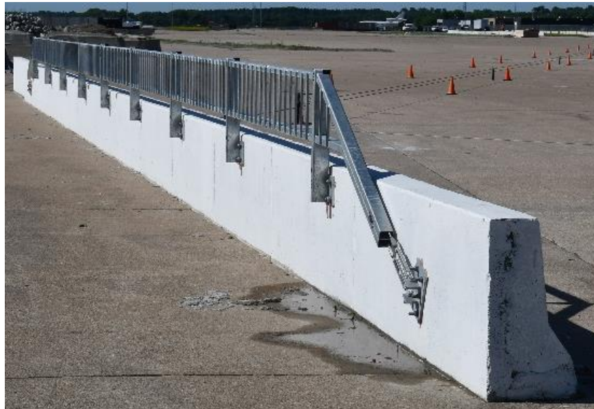
Figure 1. 2020 MwRSF Combination Bicycle and Pedestrian Bridge Railing Installation
