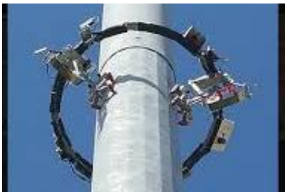
Figure 60. Visual inspection of a metal pole.
