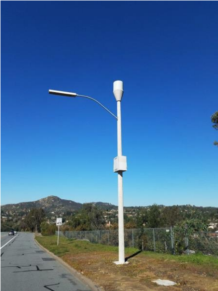
Figure 11. Small cells on streetlight poles using utility boxes that connect midway up the pole. (Left to right: Center for Electromog Prevention, n.d.; Fiber Optic Association, Inc., 2018)
