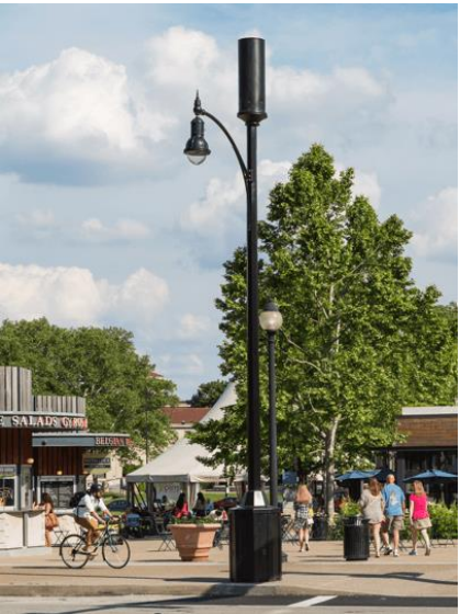
(a) A small-cell utility box on the ground. (Raycap, 2020)
