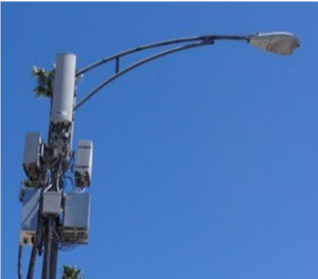
(b) Small-cell utility boxes near the top of the pole. (Tellus Venture Associates, 2016)
