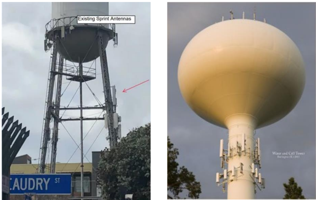
Figure 17. Small cells hosted on water towers (Left to right: E'Ville Eye, 2018; EM Watch, 2020).
