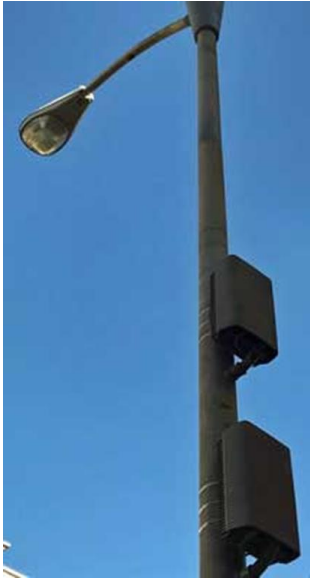
Figure 11. Small cells on streetlight poles using utility boxes that connect midway up the pole. (Left to right: Center for Electromog Prevention, n.d.; Fiber Optic Association, Inc., 2018)
