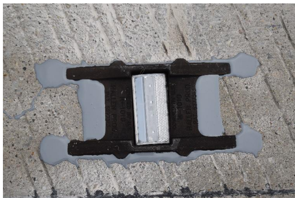
Figure 11. Example installation photo of an H1010 marker on I-70.
