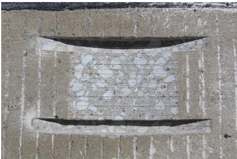
Figure 6. Completed cut for SRPMs with rails.
