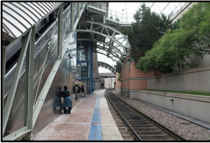
(a) Leveled platform of transit station
