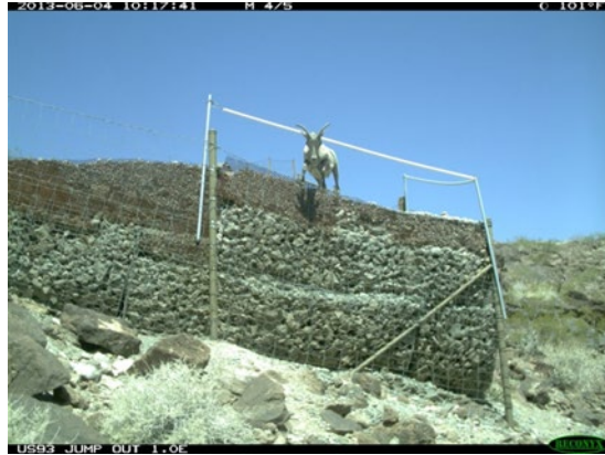
Figure 31. Bighorn Sheep Using an Escape Ramp with PVC that Accentuates the Wire
