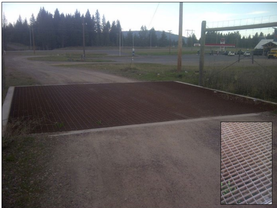
Figure 58. Montana Example of Grate-Style Wildlife Guard Along U.S. Route 93; Inset Photograph Showing Grate Detail
