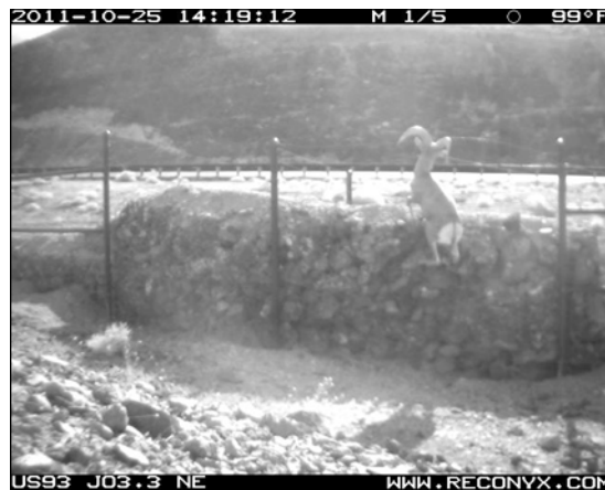
Figure 30. Wire Preventing Bighorn Sheep from Using an Escape Ramp to Enter the ROW
