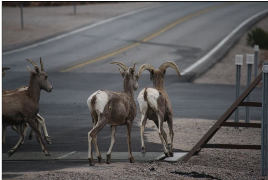
Figure 49. Ledge Allowing Animals to Access the ROW via a Wildlife Guard
