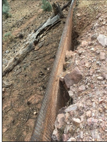
Figure 42. Soil Loss Around an Expanded Metal Mesh Retainer
