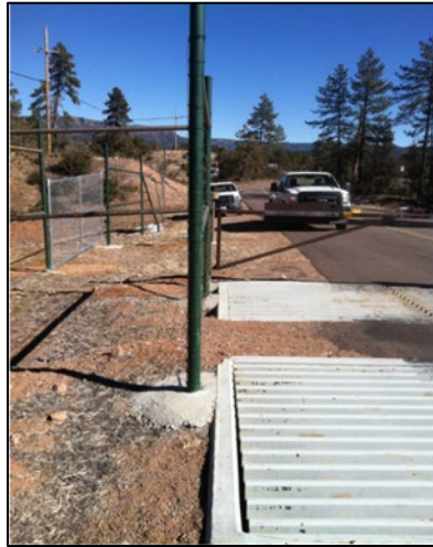
Figure 48. Large Distance Between Double Cattle Guards and Short Fence
