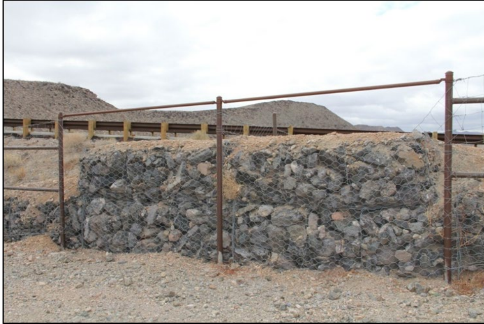
Figure 3. Gabion Basket Escape Ramp
