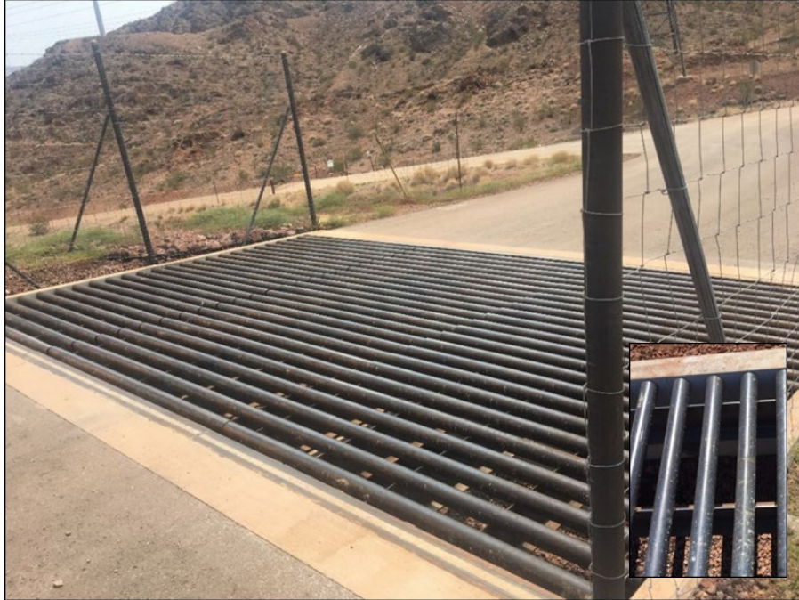
Figure 57. Wildlife Guard with Round Bars to Deter Wildlife Located on an Arizona-Nevada Joint Project Along Interstate 11; Inset Photograph Showing Round Bar Detail
