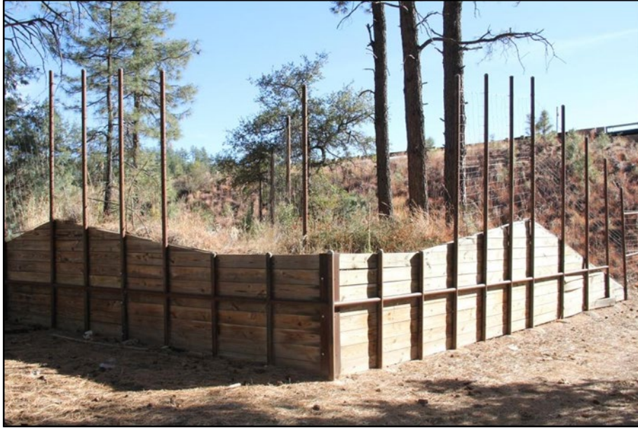
Figure 1. Wooden Escape Ramp
