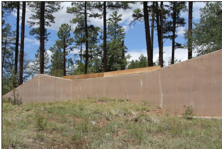
Figure 23. Board Added Along the Top of an Escape Ramp to Increase Its Height
