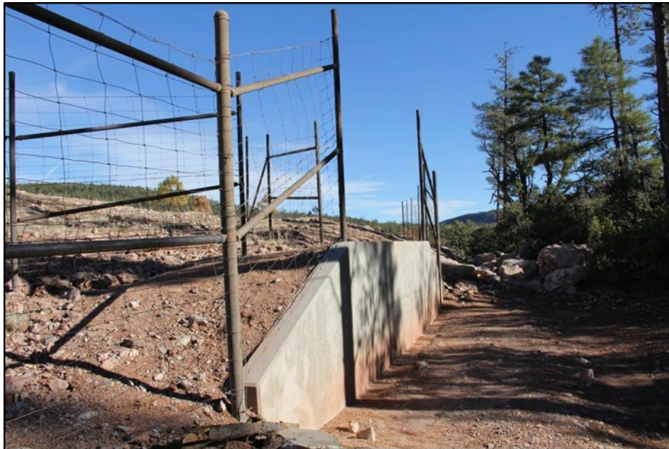
Figure 2. Concrete Escape Ramp
