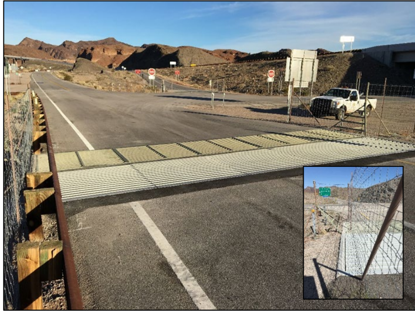
Figure 59. Wide Wildlife Guard to Deter Jumping, with Guardrail or Fence to Prevent Walking on the Vault Edge, Along U.S. 93; Inset Photograph Showing Fencing Detail
