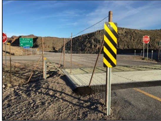
Figure 36. Double Cattle Guard with Fencing
