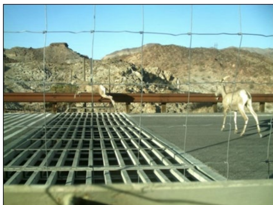
Figure 35. Bighorn Sheep Jumping a Cattle Guard at Kingman Wash TI Despite Painted Stripes
