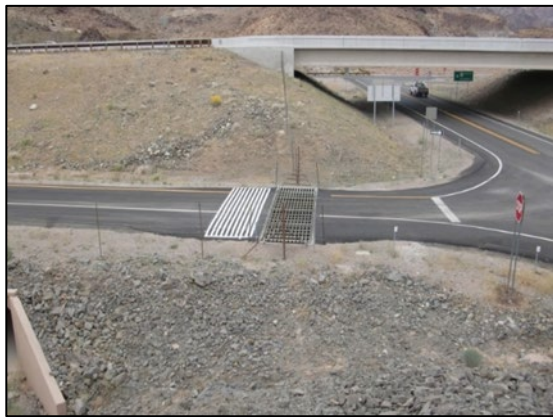
Figure 34. Painted Stripes Mimicking an Additional Cattle Guard
