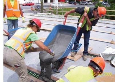
Figure 1. (a) The first UHPC bridge constructed in the U.S (in Wapello County, IA), (b) casting of longitudinal connections between deck-bulb-tee girders (Route 31 Bridge, Lyons, NY). Both figures courtesy of FHWA ( https://www.fhwa.dot.gov/publications/research/infrastructure/structures/11038/ )
