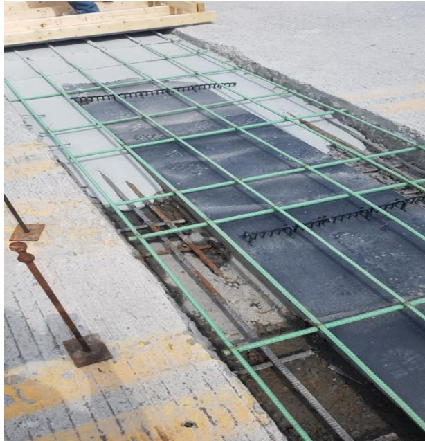
Figure 138. Transverse (LLC) joints filled with UHPC
