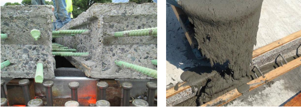
Figure 6. UHPC being used as connection joints between precast deck panels
