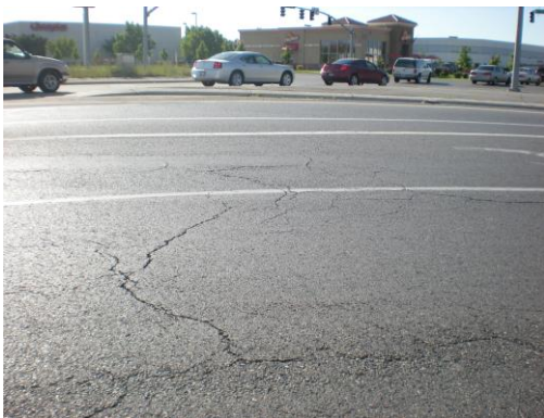
(c) Ramp facing north-west
