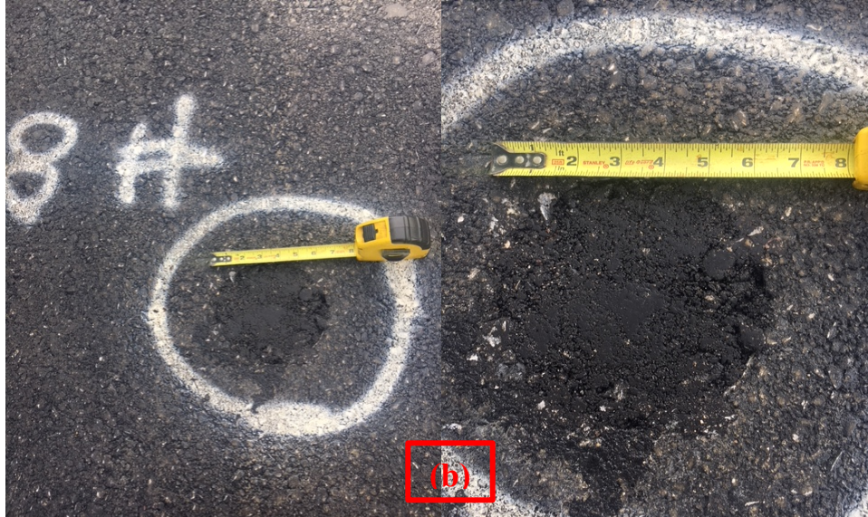
Figure 11. The process of (a) Pavement Quality Indicator and (b) Core extraction
