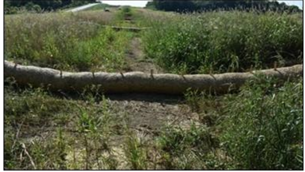
(b) 7/26/2019, installation - downstream
