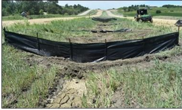
(a) 7/26/2019, installation - upstream
