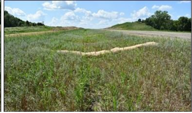
(b) 7/26/2019, installation - downstream
