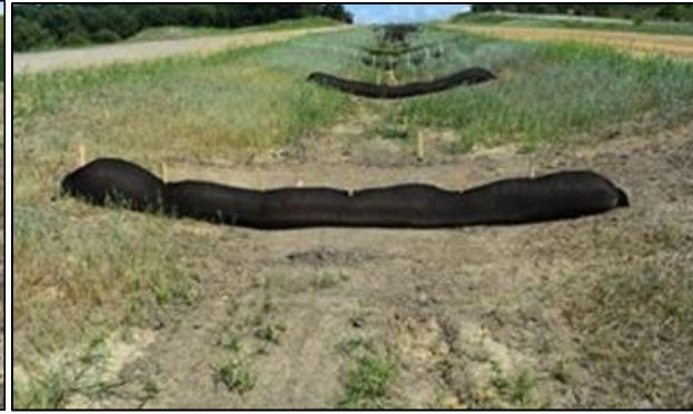
(b) 7/26/2019, installation - downstream
