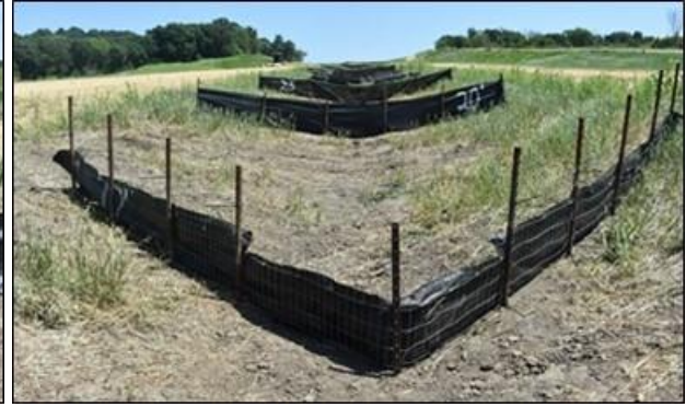
(b) 7/26/2019, installation - downstream
