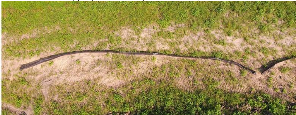
(b) Inspection 9/5/2019, 3.53 in. (8.97 cm) rainfall
