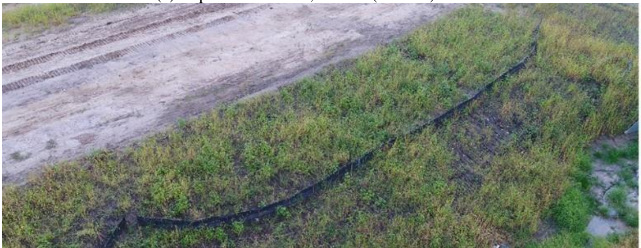
(c) Inspection 9/24/2019, 6.78 in. (17.22 cm) rainfall
