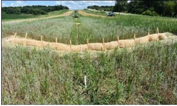
(a) 7/26/2019, installation - upstream
