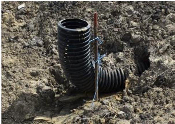
(b) Riser pipe structure
