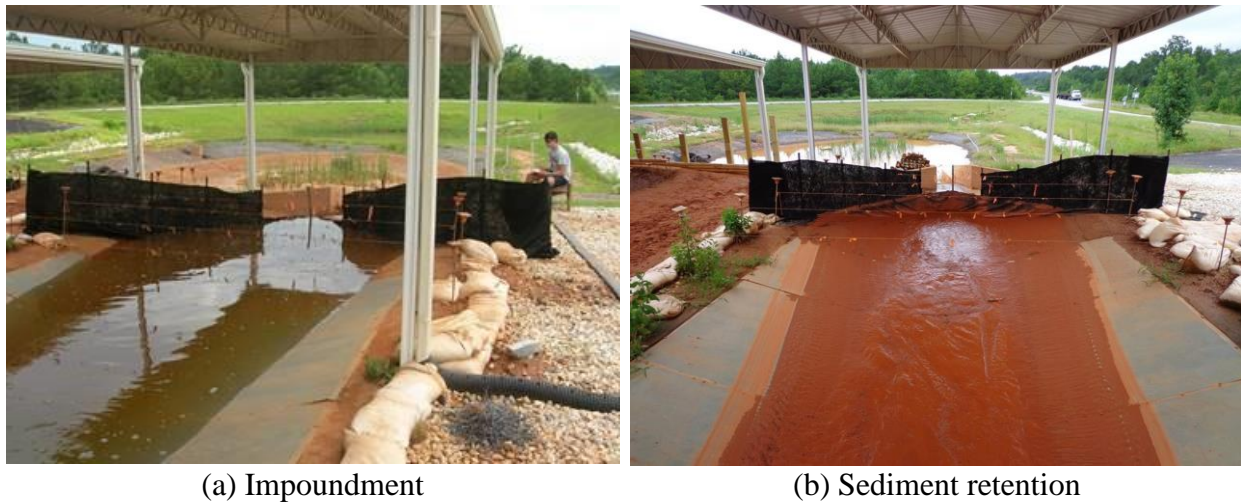
Figure 4.3. Longevity evaluation of pinned silt fence ditch check
