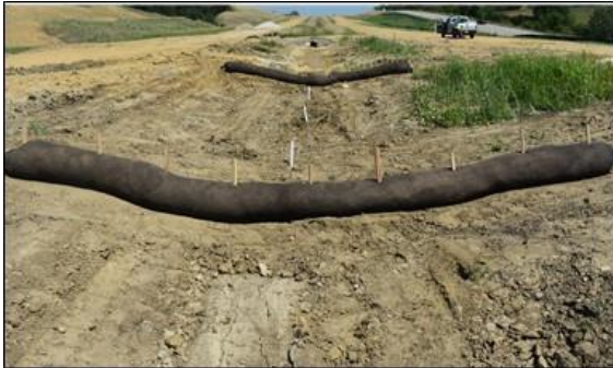
(a) 7/26/2019, installation - upstream
