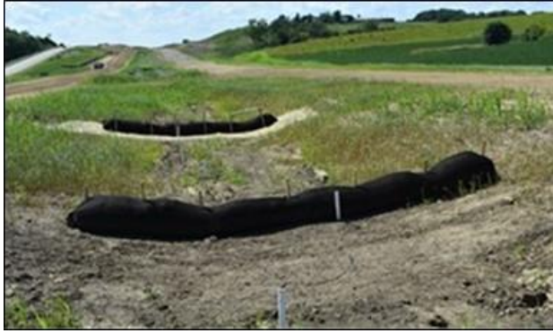
(a) 7/26/2019, installation - upstream
