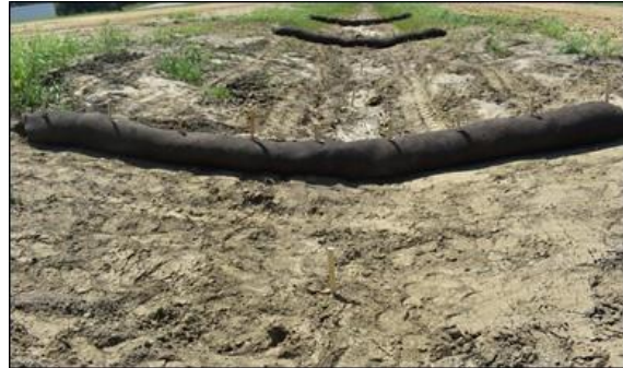
(b) 7/26/2019, installation - downstream
