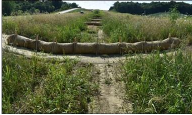
(a) 7/26/2019, installation - upstream
