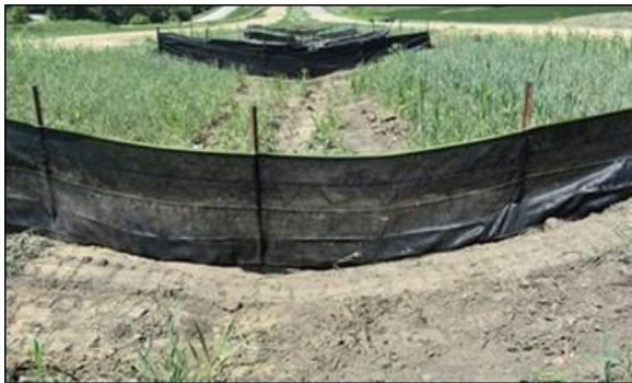
(a) 7/26/2019, installation - upstream
