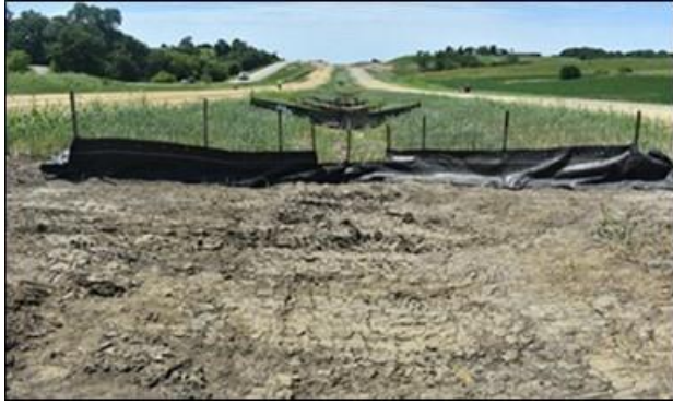
(a) 7/26/2019, installation - upstream
