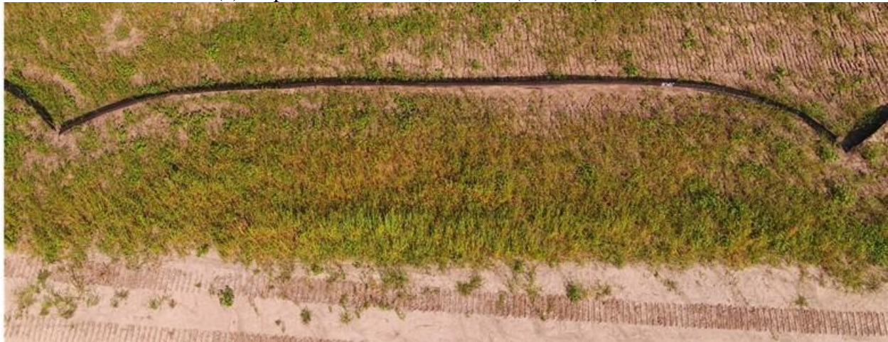
(b) Inspection 9/5/2019, 3.53 in. (8.97 cm) rainfall
