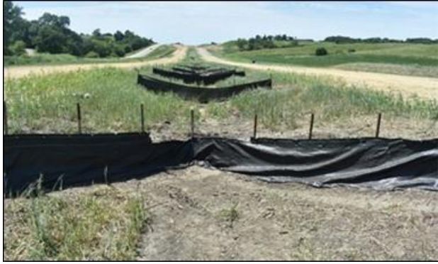
(a) 7/26/2019, installation - upstream
