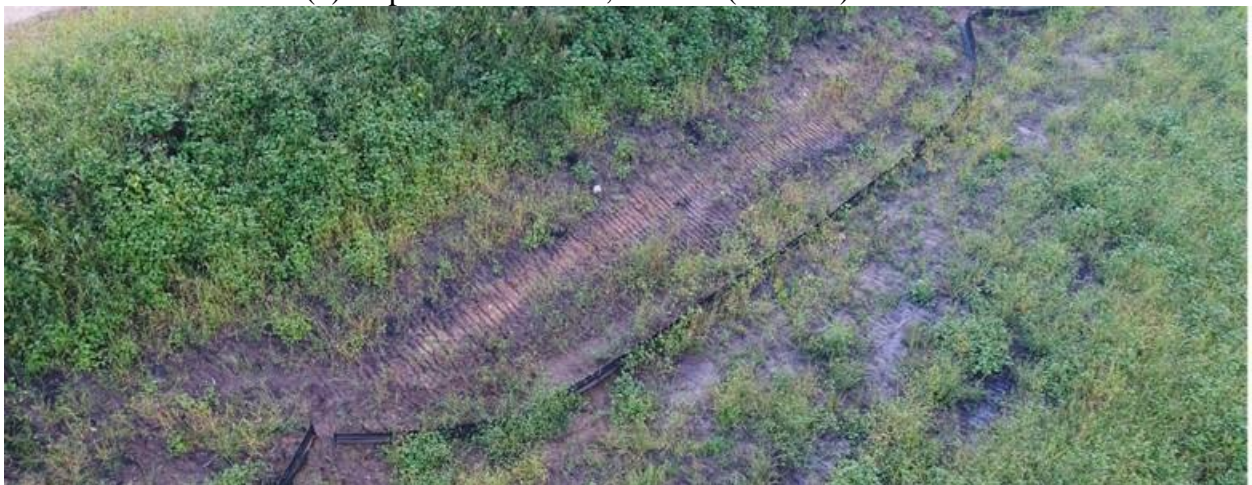
(c) Inspection 9/24/2019, 6.78 in. (17.22 cm) rainfall
