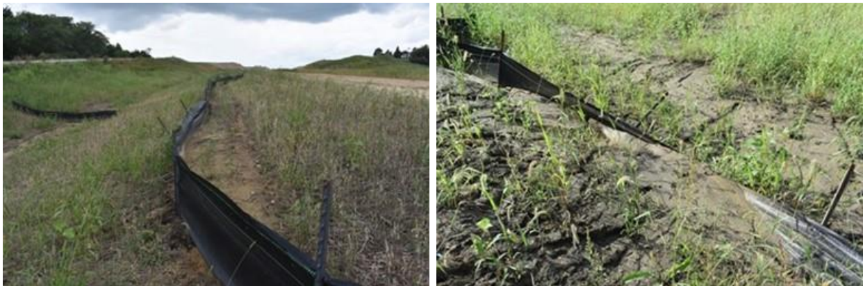
(a) Post deflection on SF-PC-S1 (9/5/2019) (b) Post deflection on SF-PC-S2 (9/5/2019)
