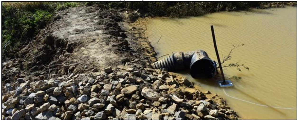
(b) Sample float system at discharge
