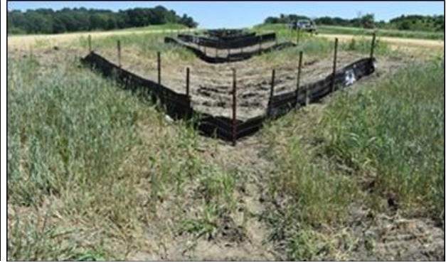
(b) 7/26/2019, installation - downstream
