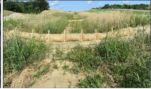
(b) 7/26/2019, installation - downstream
