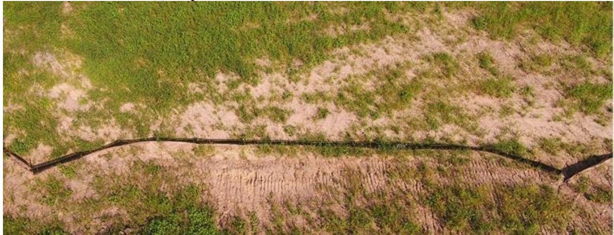
(b) Inspection 9/5/2019, 3.53 in. (8.97 cm) rainfall
