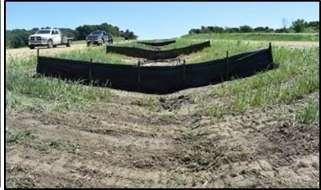
(b) 7/26/2019, installation - downstream
