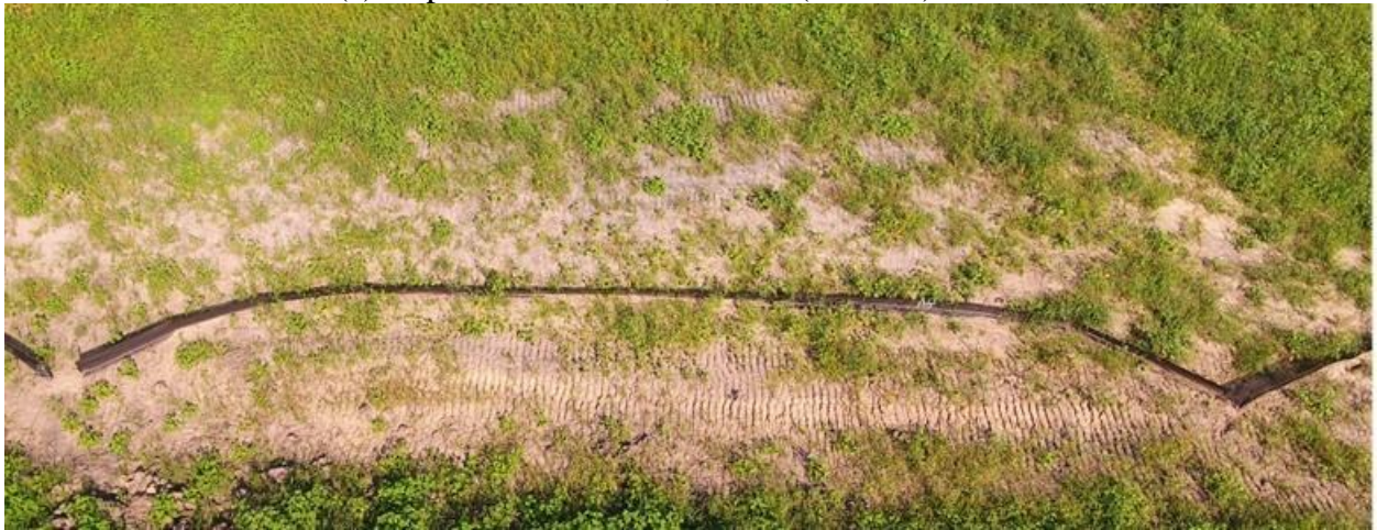
(b) Inspection 9/5/2019, 3.53 in. (8.97 cm) rainfall
