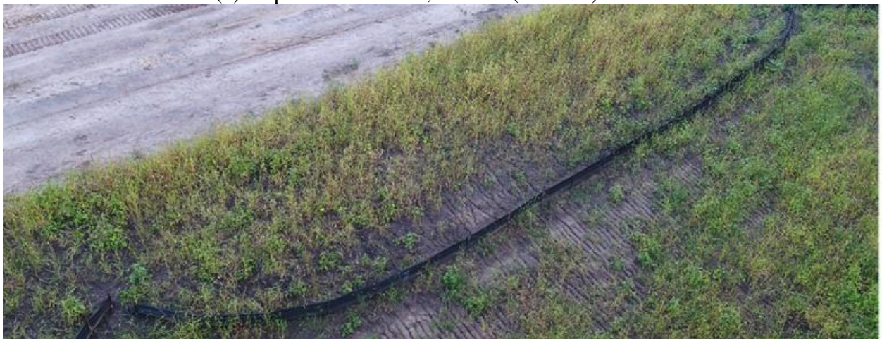
(c) Inspection 9/24/2019, 6.78 in. (17.22 cm) rainfall
