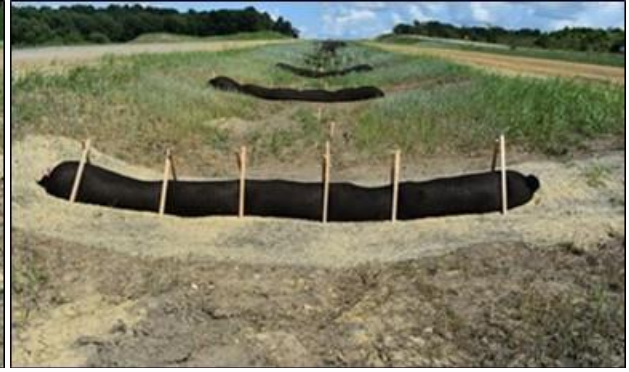
(b) 7/26/2019, installation - downstream
