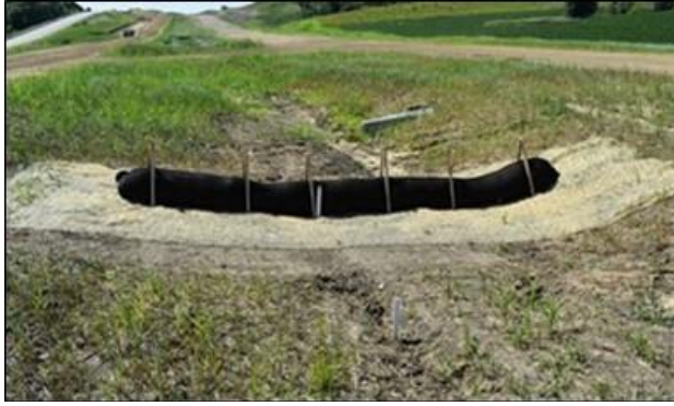
(a) 7/26/2019, installation - upstream
