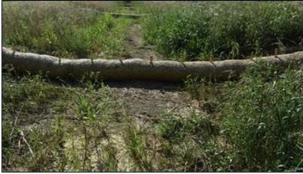
(a) 7/26/2019, installation - upstream
