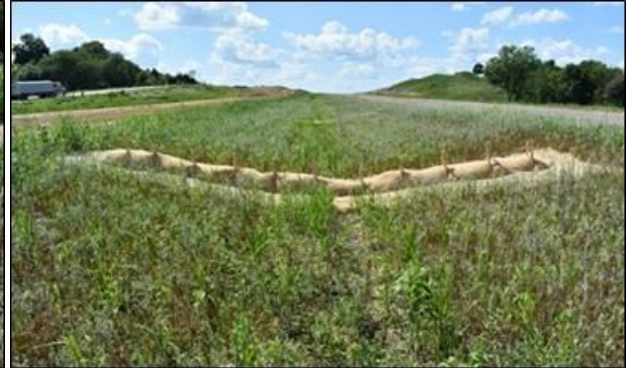
(b) 7/26/2019, installation - downstream
