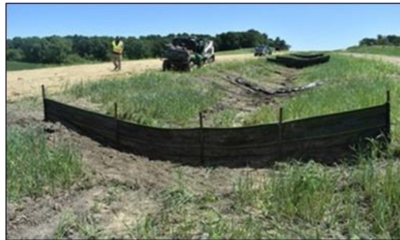
(b) 7/26/2019, installation - downstream
