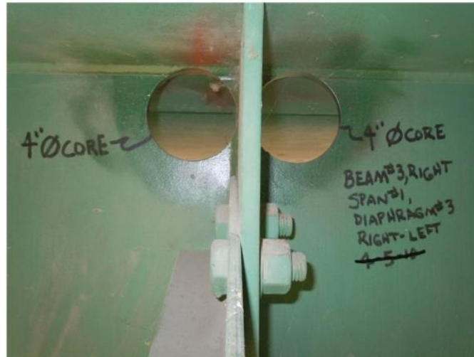
Figure 2.5. Arrest holes drilled in diaphragm stiffener
