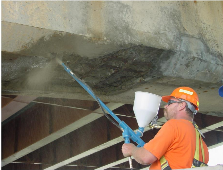
Figure 2.7. Shooting material for shotcrete repair
