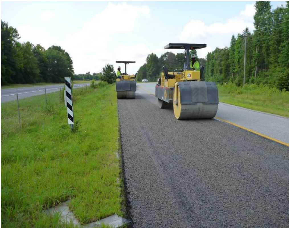
Figure 6. Compaction Using Steel Rollers
