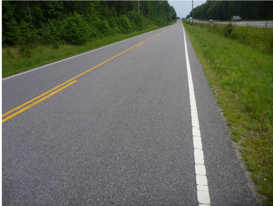
Figure 20. FiberMat With Microsurfacing After 3 Years
