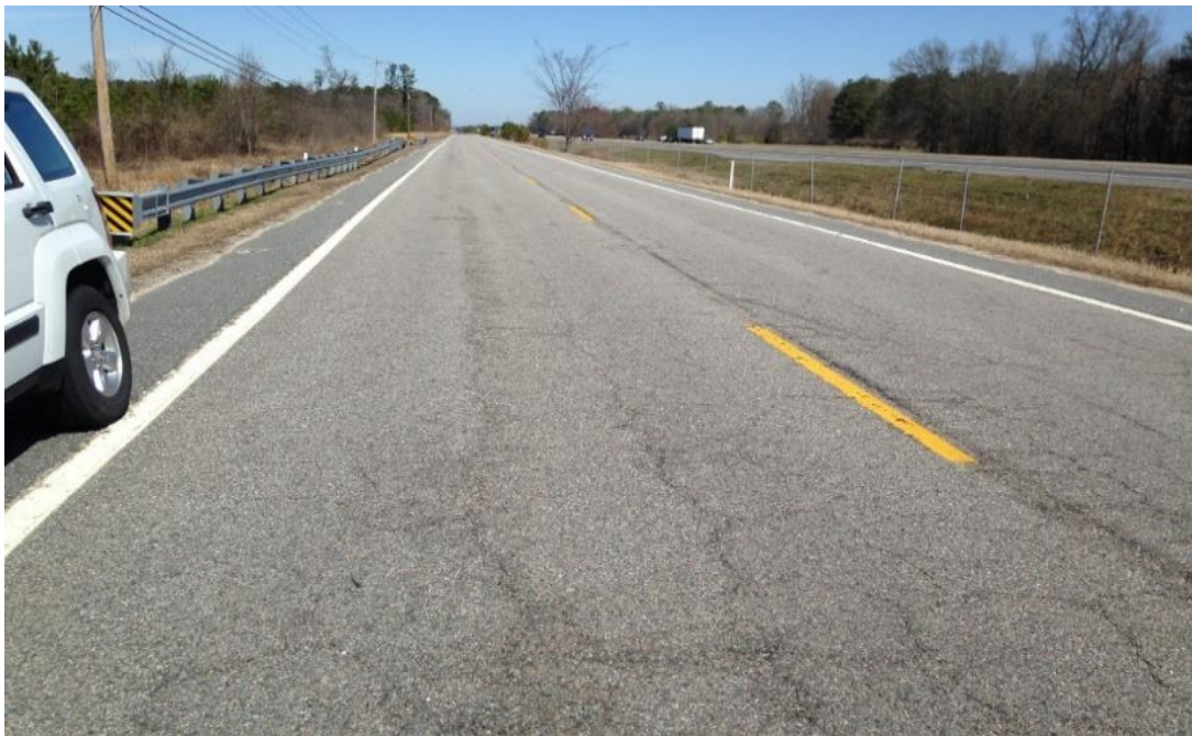
Figure 10. Section With Moderate Amount of Cracking
