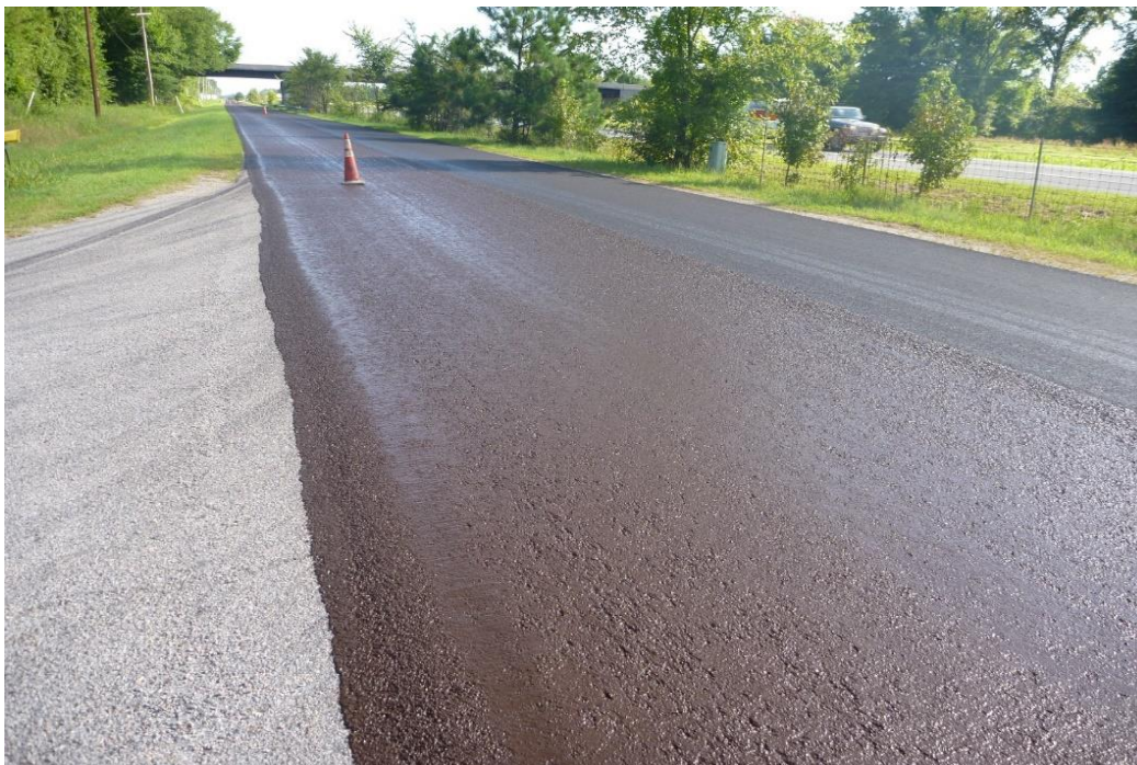
Figure 8. Microsurfacing Before Opening to Traffic
