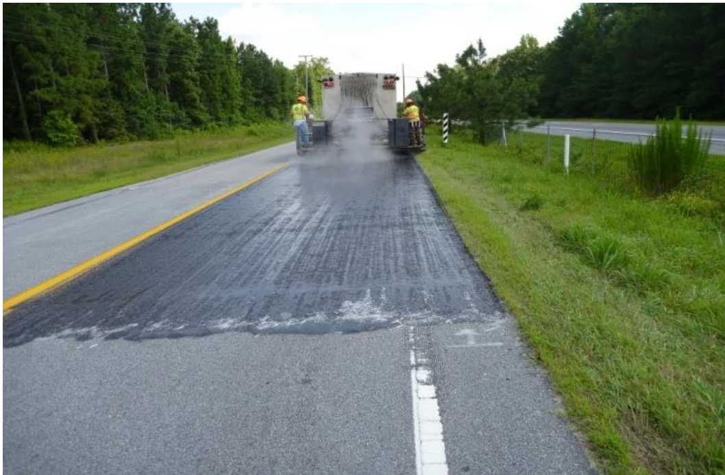
Figure 2. Placement of Fibers and Emulsion
