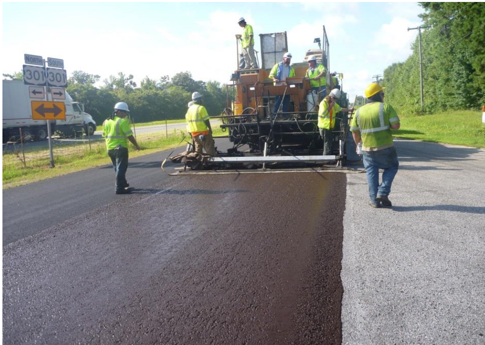
Figure 7. Microsurfacing Placement
