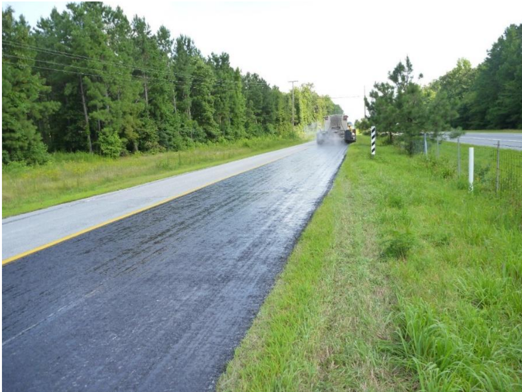
Figure 4. Emulsion With Fibers in Between
