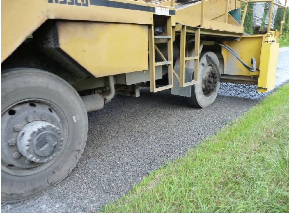
Figure 5. Aggregate Spreading
