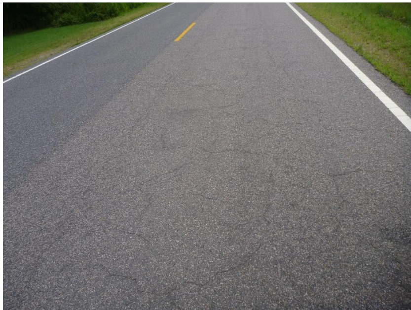
Figure 23. Microsurfacing Section After 3 Years
