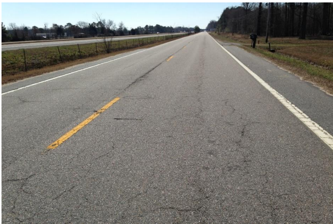
Figure 11. Section With Lower Amount of Cracking
