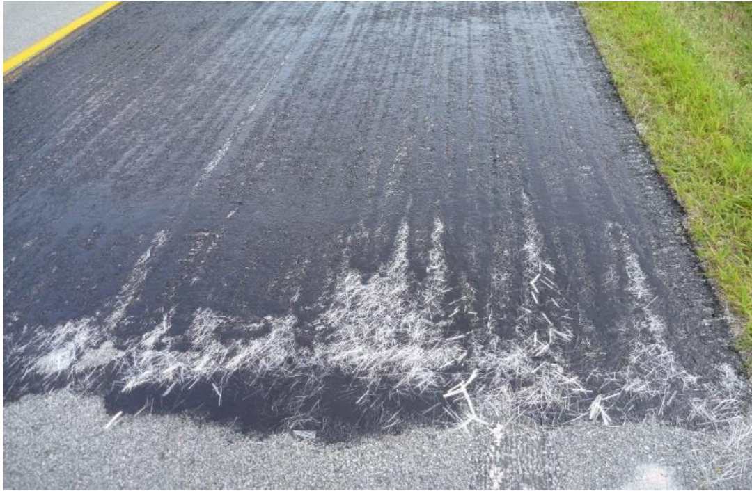
Figure 3. Placement Showing Fibers at Beginning of Section
