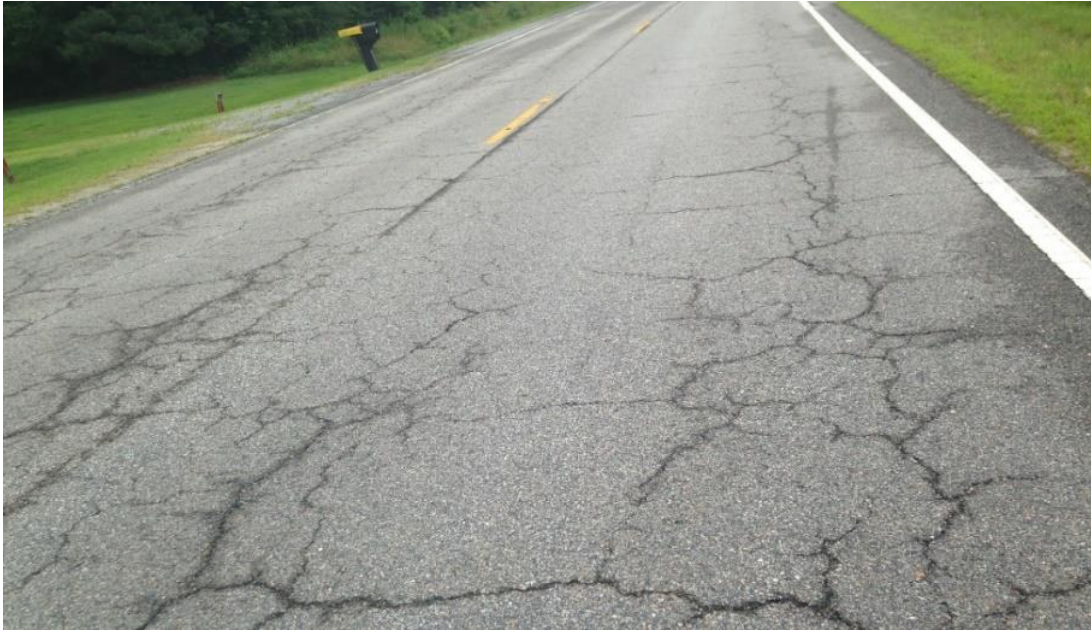
Figure 9. Section With Large Amount of Cracking
