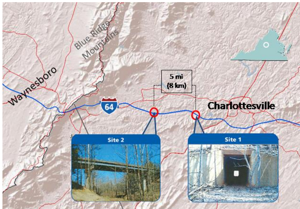
Figure 1. Locations of Existing Underpass Study Sites (Donaldson et al., 2016)
