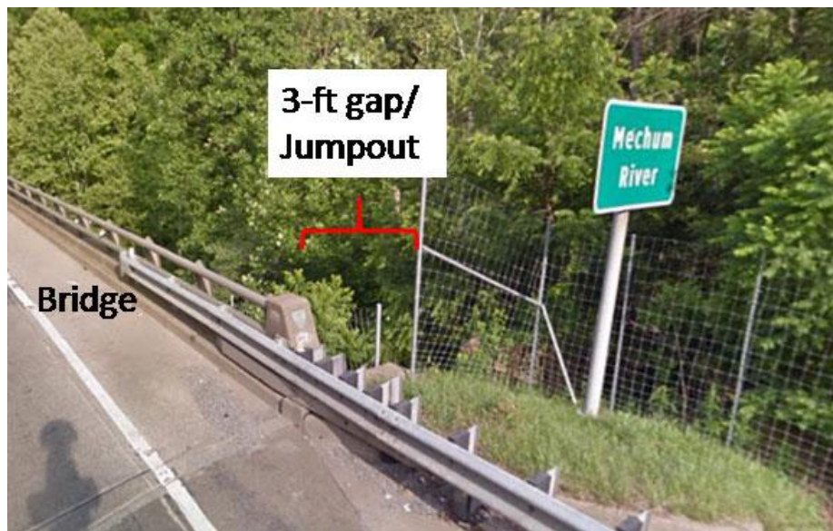
Figure 3. Fence at Site 2 Underpass. The gap between the fencing and the bridge was designed to serve as a jumpout to allow wildlife on the traffic side of the fence to access the underpass below.
