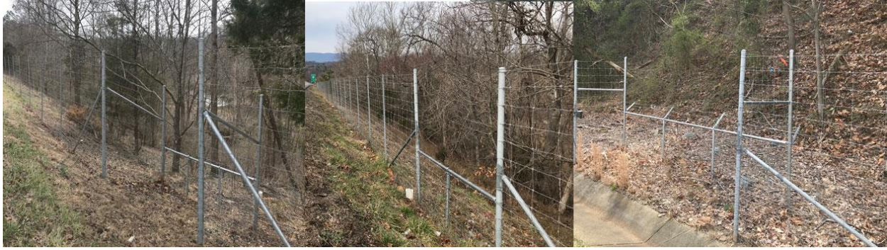
Figure 5. Jumpout Designs at Study Sites: left, jumpout set farther back from the road and on a downslope (with no angled attachment); center, jumpout in line with the fence and on a downslope (with no angled attachment); right, jumpout set farther back from the road on level ground (with the angled attachment)
