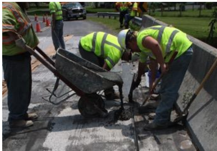
Figure 99. Dumping VHPC from Wheelbarrow
