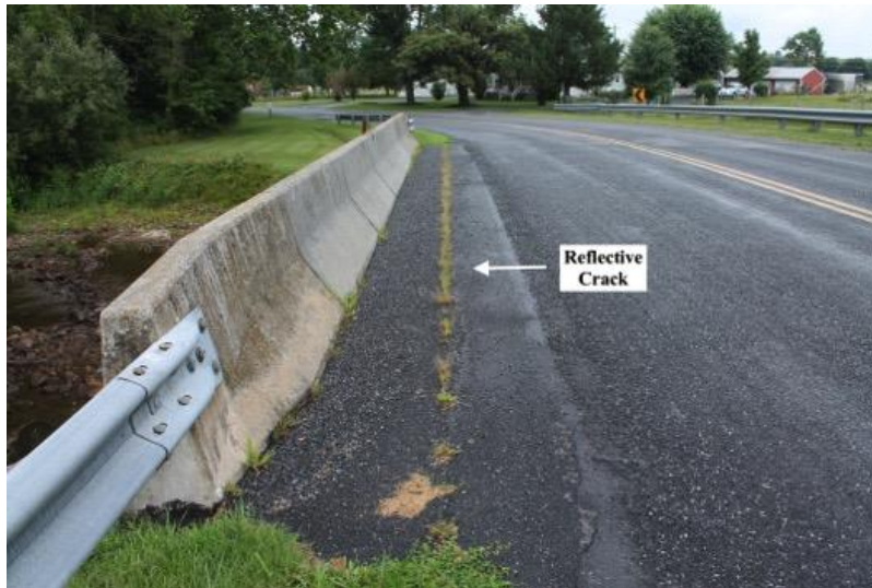
Figure 1. Reflective Cracking
