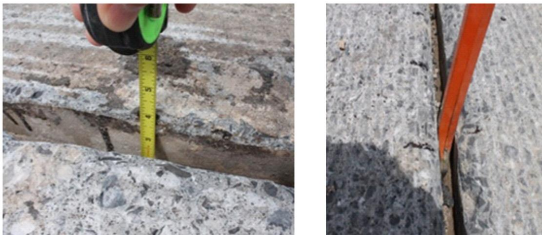
Figure 91. Typical Depth of Cleared Joints and Removing Grout from Joints with (a) Bonded Grout and (b) Deteriorated, Sandy Grout
