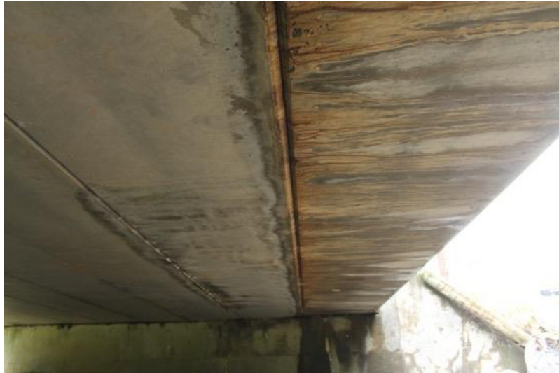
Figure 2. Leaking Joint
