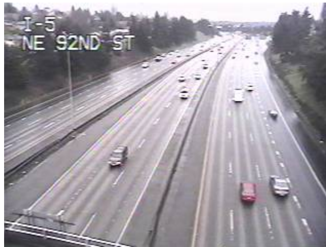
Figure 7-4: Southbound I-5 Near the NE 92 nd Street Over-crossing
