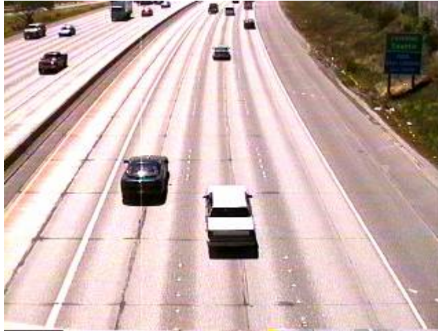
Figure 7-1: Southbound I-5 Near the NE 145 th Street Over-crossing
