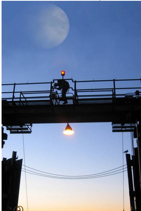
Fig 6 – Antenna installation on terminal
