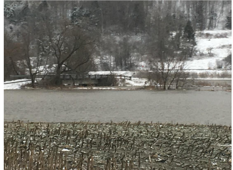
View to southwest to bridge outlet, from Brusso Rd, 12/22/2018
