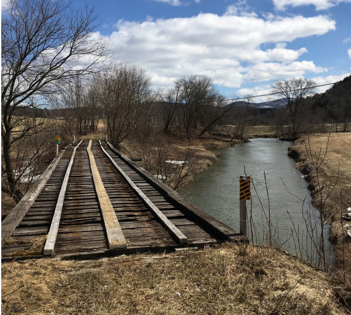
4 April 2019, view to east of bridge decking
