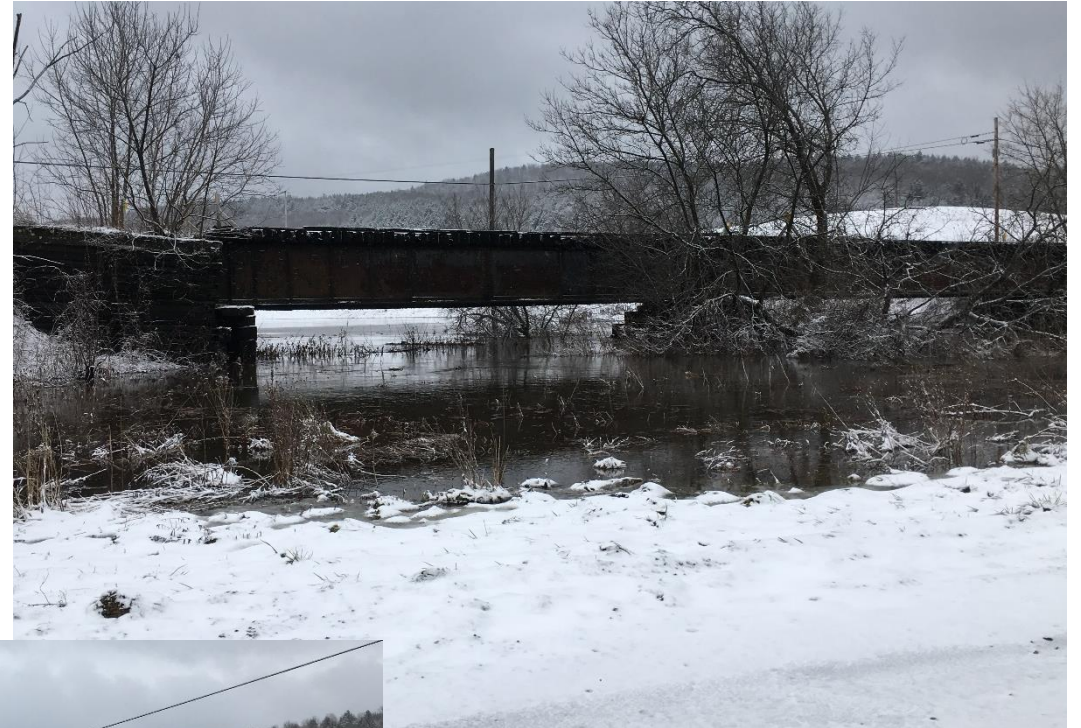
View upstream to bridge outlet from Elm Brook Rd, 12/22/2018
