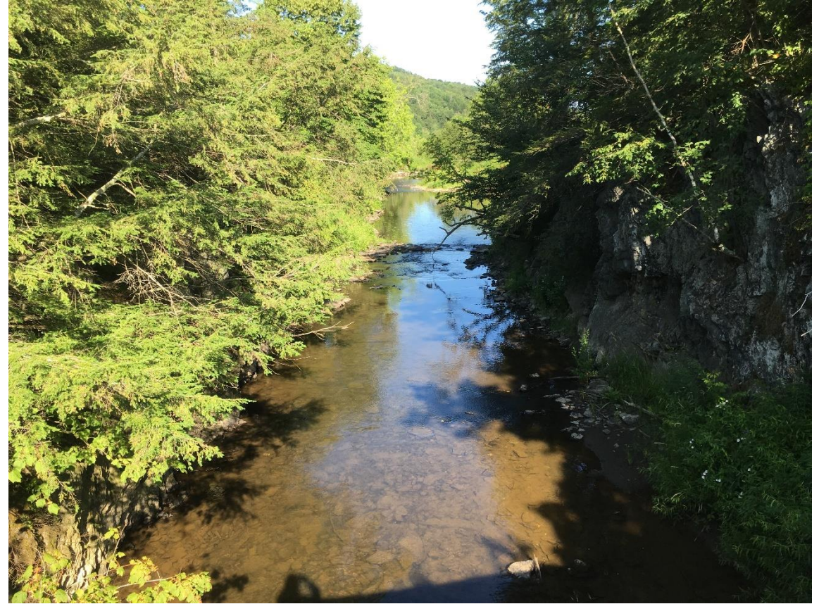
View downstream from bridge deck, 7/24/2019, through blasted bedrock channel
