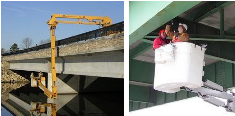
Figure 2.1 Visual Inspection Techniques for Bridges
