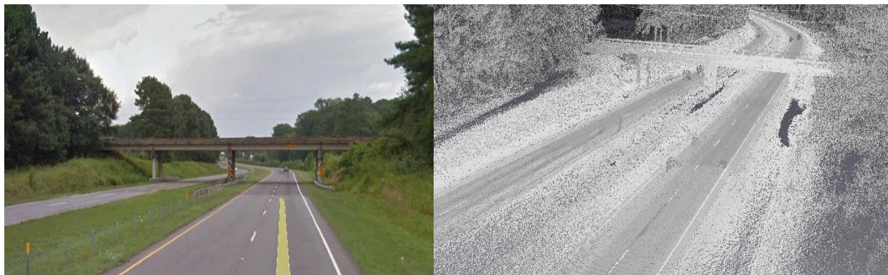
Figure 4.18 Example of LiDAR point cloud and corresponding picture
