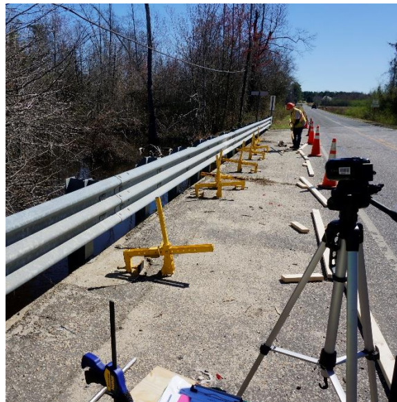
Figure 16. Preparation for Installation Activities
