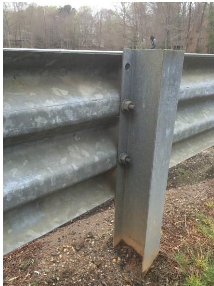
Figure 98 - Guardrail Type 25, post variation # 2
