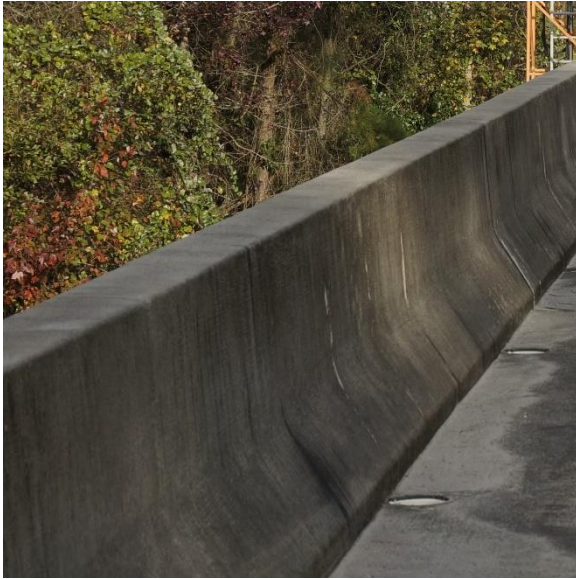
(a) Jersey barrier guardrail
