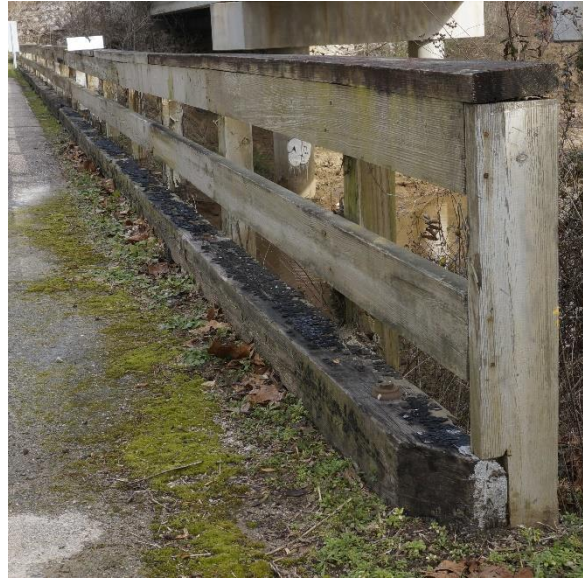
(b) Timber guardrail
