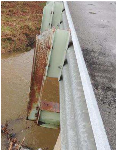
Figure 97 - Guardrail Type 25, post variation # 1
