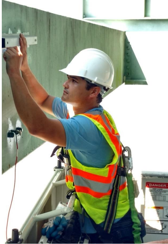
Figure 23. Installation of the VW Strain Gages by Graduate Student Justin Alexander
