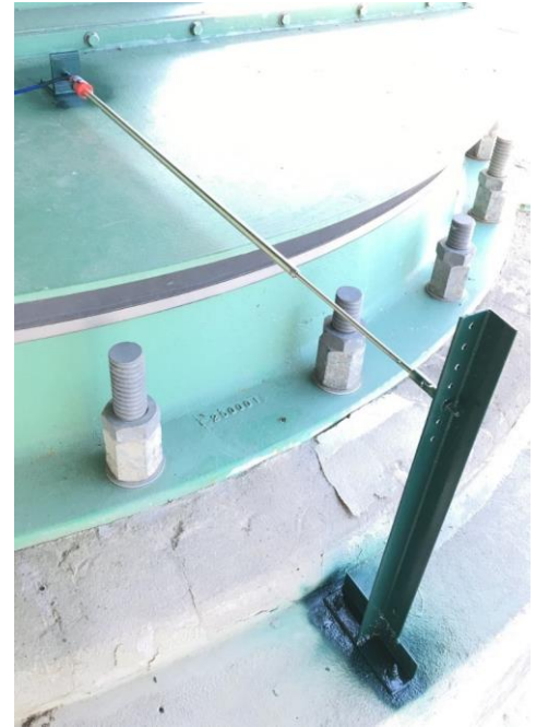
Figure 24. VW Displacement Gage Installation at Pier A (Pier C similar)
