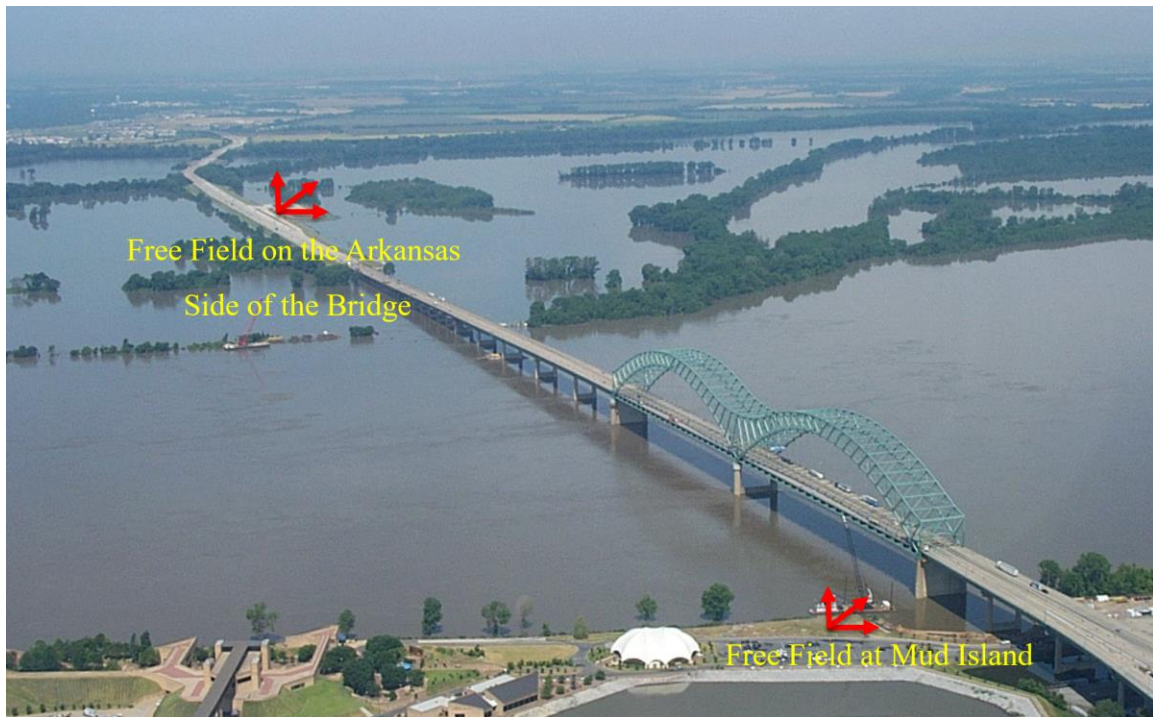
Figure 5. Free-field sensor locations. Note that this photo was taken during the May, 2011 flood. On May 10, 2011 the Mississippi river crested in Memphis at 47.8 feet above flood stage. Normally the weigh station is about a mile west of the unflooded river bank.
