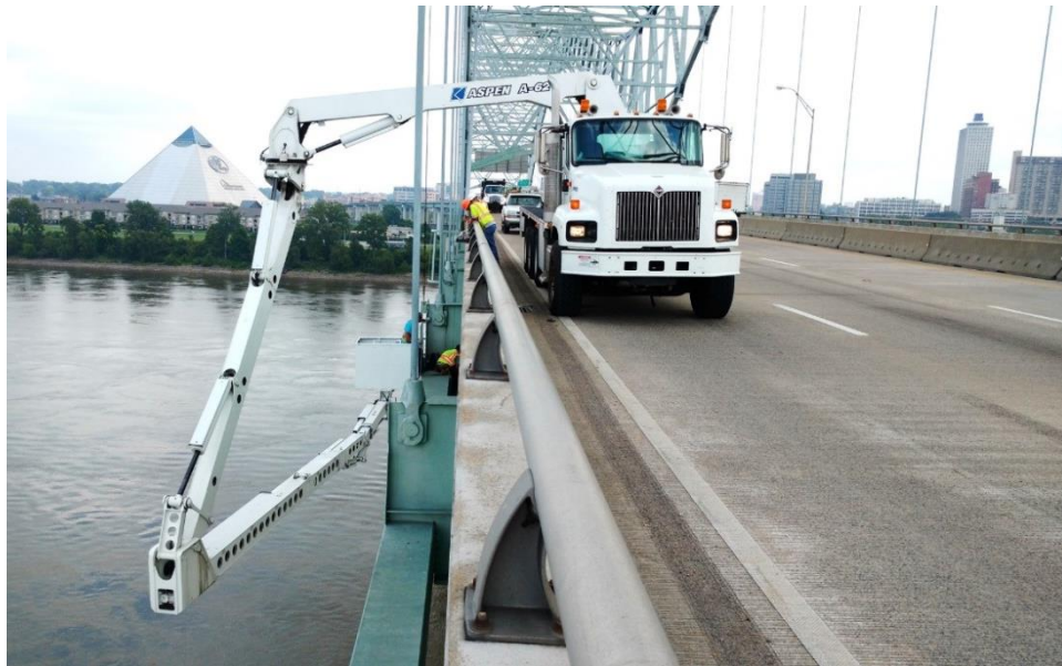
Figure 22. Installation of VW Strain Gages along the Lower Chord
