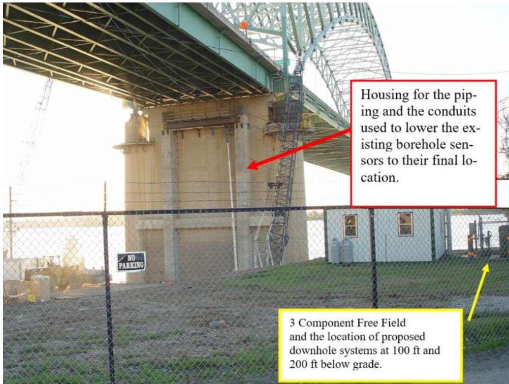
Figure 7. The location where the piping and of the downhole instruments at Pier C and the location of the downhole systems at 100 ft and 200 ft below grade. The sensors at 100 and 200 ft below grade were part of a separate activity and are currently inoperable pending funding to replace the instruments.
