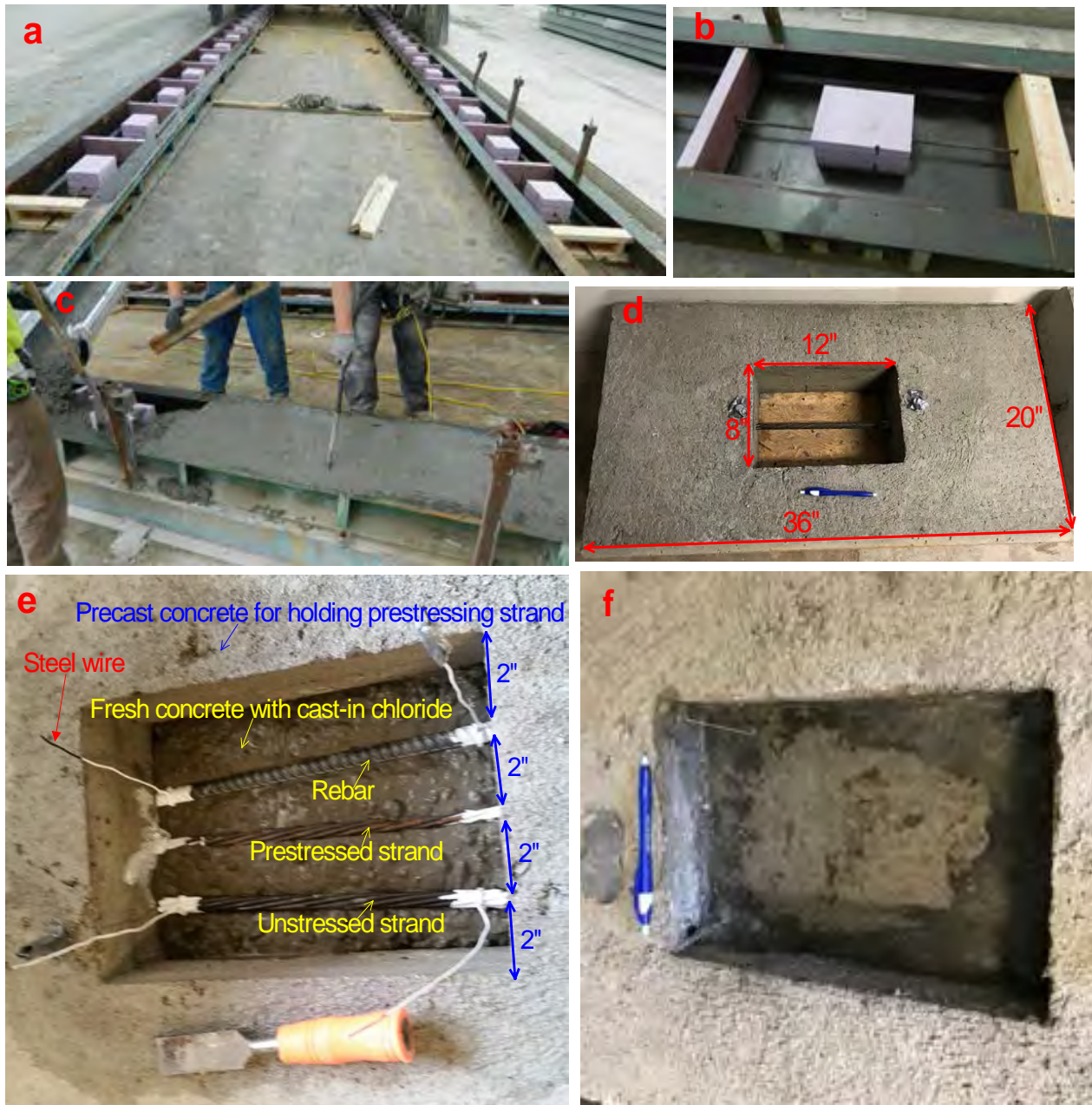
Figure 3.3 Specimen preparation for comparing corrosion among rebar, prestressed strand, and unstressed strand using cast-in sodium chloride: (a) Precast/prestressing concrete bed, (b) Close-up view of bed with stressed strand, (c) Pre-casting concrete for holding stressed strand, (d) Precast concrete after demolding, (e) Placing concrete with cast-in chloride and setting rebar and unstressed strand, and (f) Air curing specimen with cast-in chloride, rebar, prestressed strand, and unstressed strand
