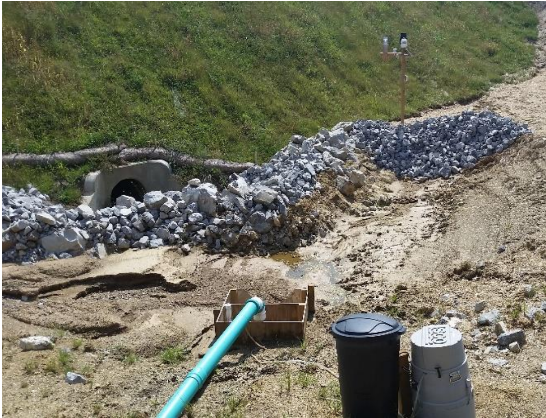
Figure 2.5. Knox County sediment basin outlet pipe and downstream condition.
