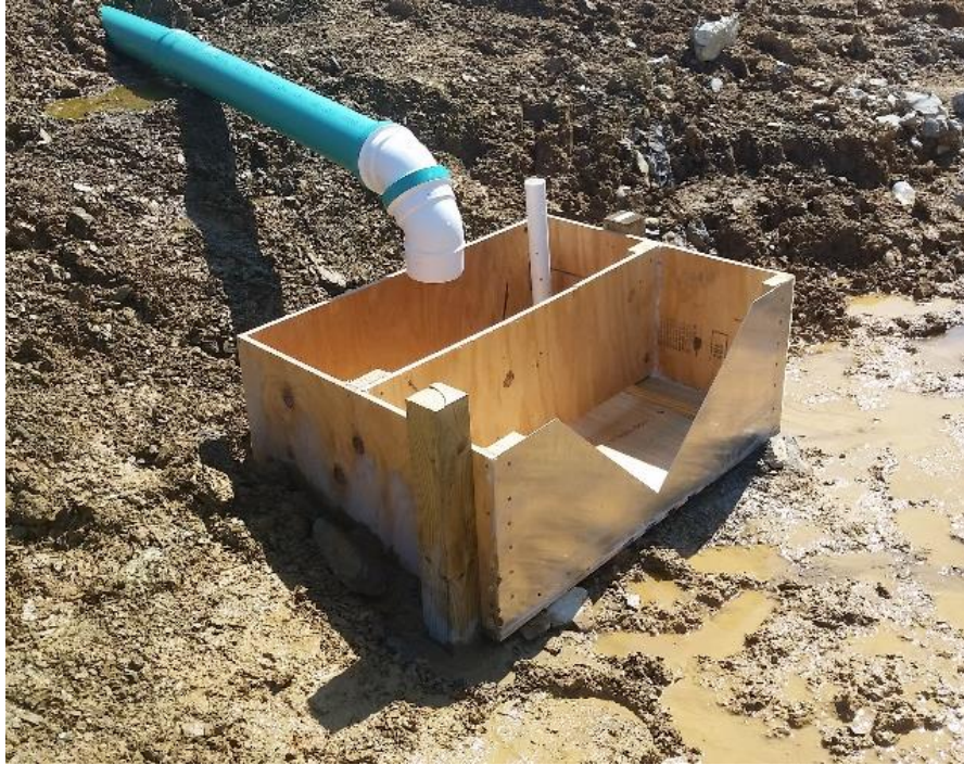
Figure 2.9. Knox County sediment basin outlet 90-degree V-notch weir box and outlet pipe.
