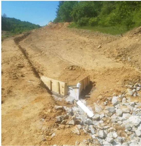
Figure 2.2. Morgan County sediment basin drainage area and inlet H-flume.
