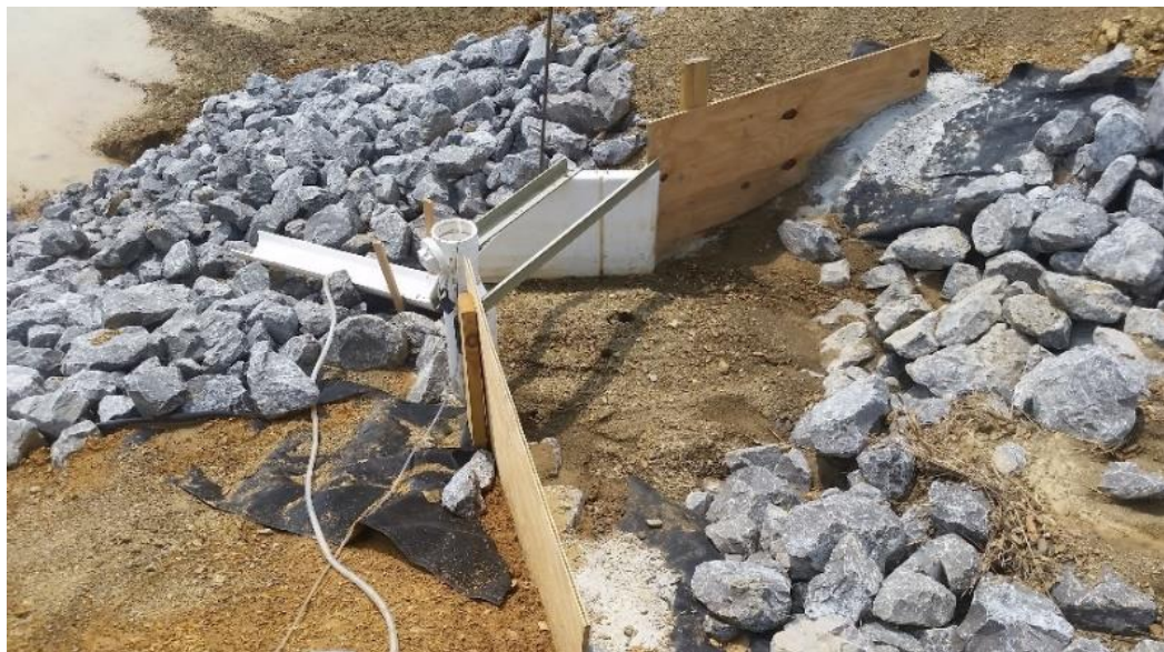
Figure 2.8. Knox County sediment basin inlet monitoring flume and accompanying materials.
