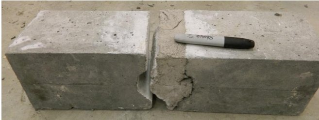
Figure A25 – Specimen broke at demolding for Phoscrete VO-Plus for all substrate surface moisture conditions (Mix #25)
