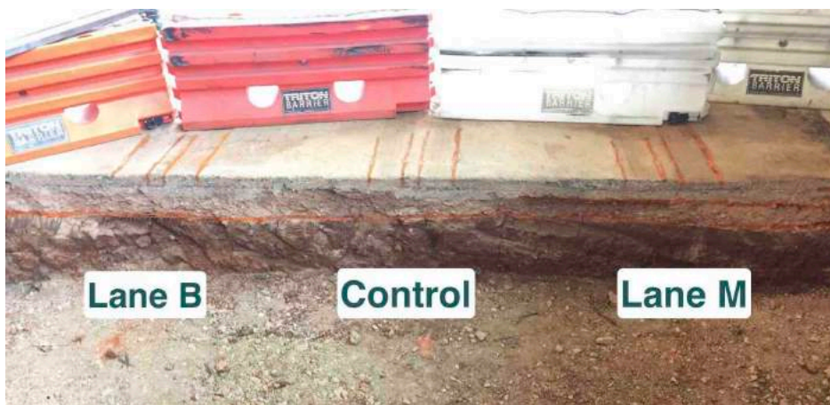
Figure 6.95: Resulted Cross Section from Trenching
