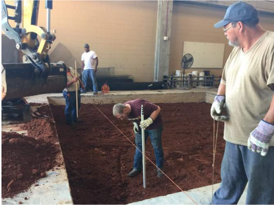
Figure 5.4: Controlling the Thickness of Subgrade
