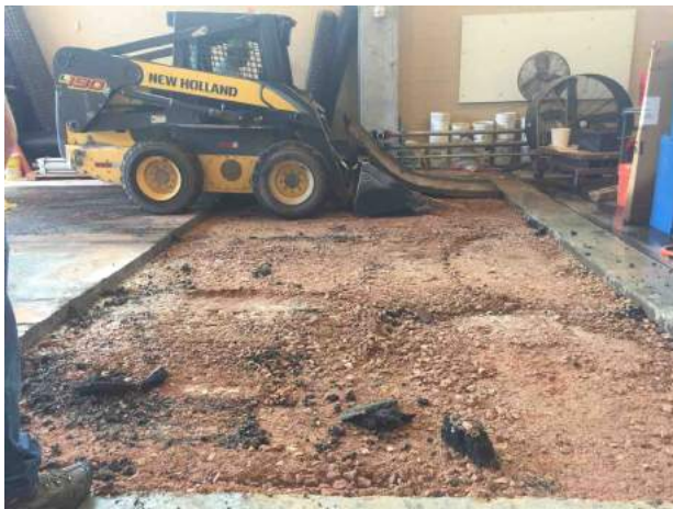
(c) Cleaning Asphalt Layer
