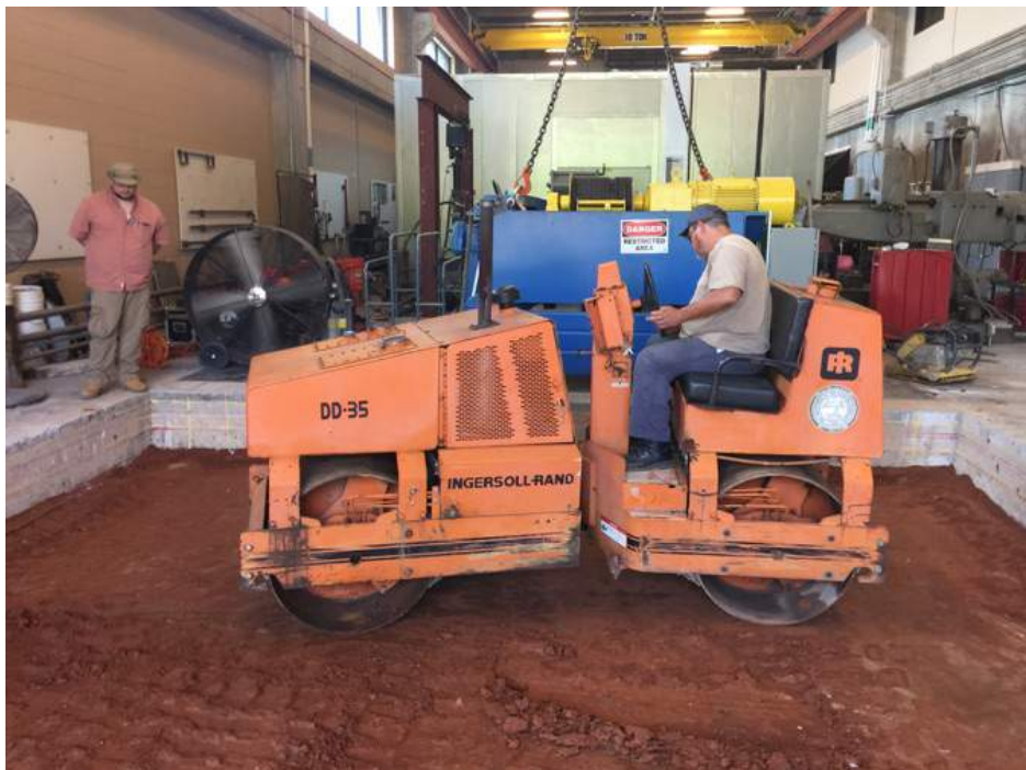
Figure 5.3: Compacting and Leveling Subgrade Soil with a Steel Wheel Roller
