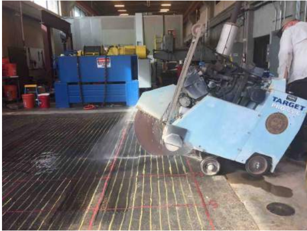
(a) Cutting Asphalt Layer
