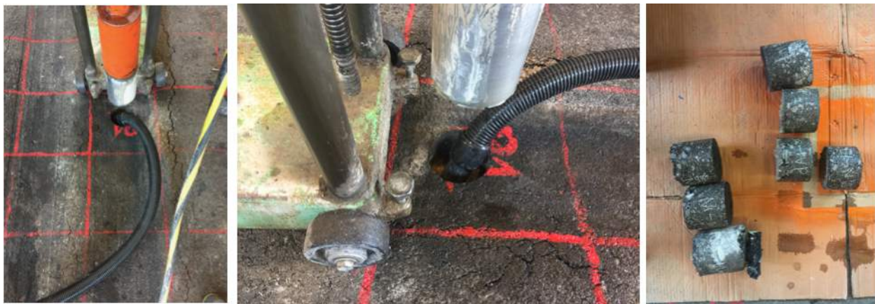
Figure 4.44: Core Drilling (Round 1)
