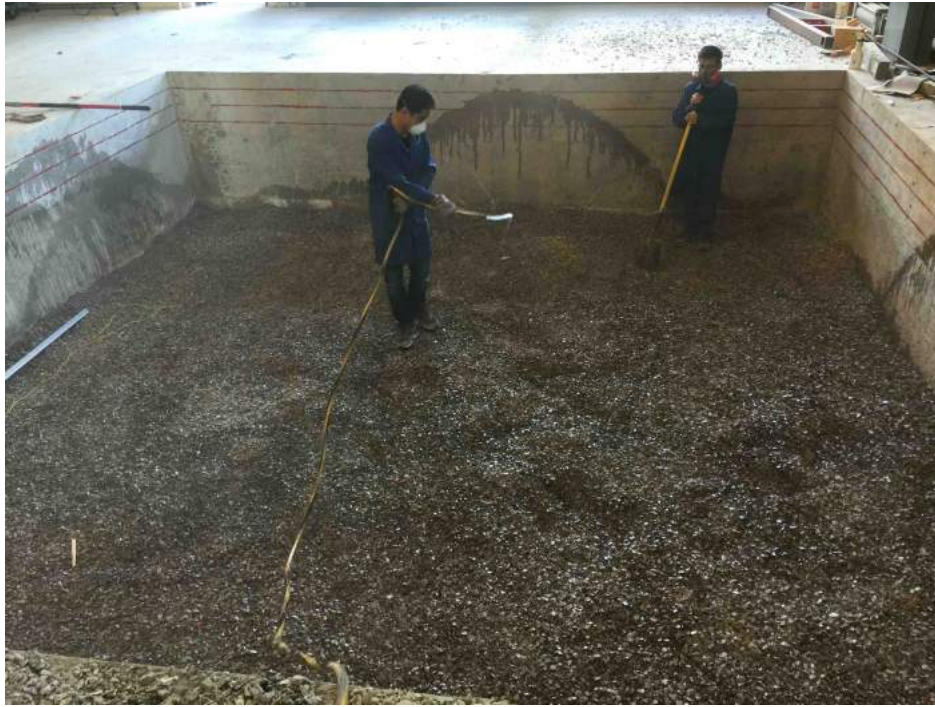
Figure 4.4: Leveling Test Pit for Subgrade Construction
