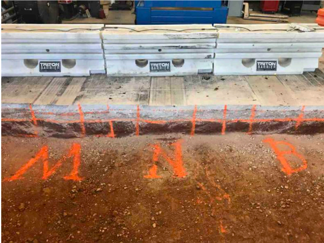
Figure 5.65: Overview of Trenched Test Pit
