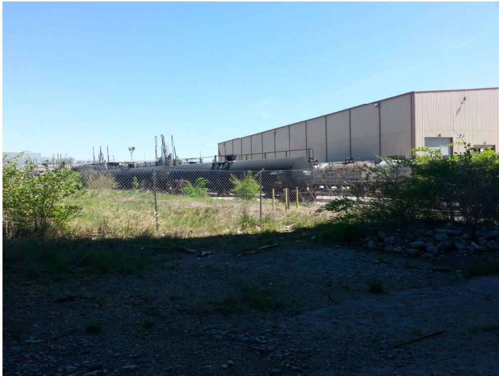
Figure 13: Example of co-location with dangerous substances. This photo is of liquid propane rail cars as seen from under the bridge deck
