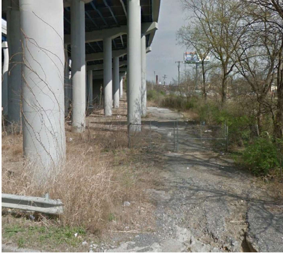
Figure 11: Example of partially controlled abutment vehicular access
