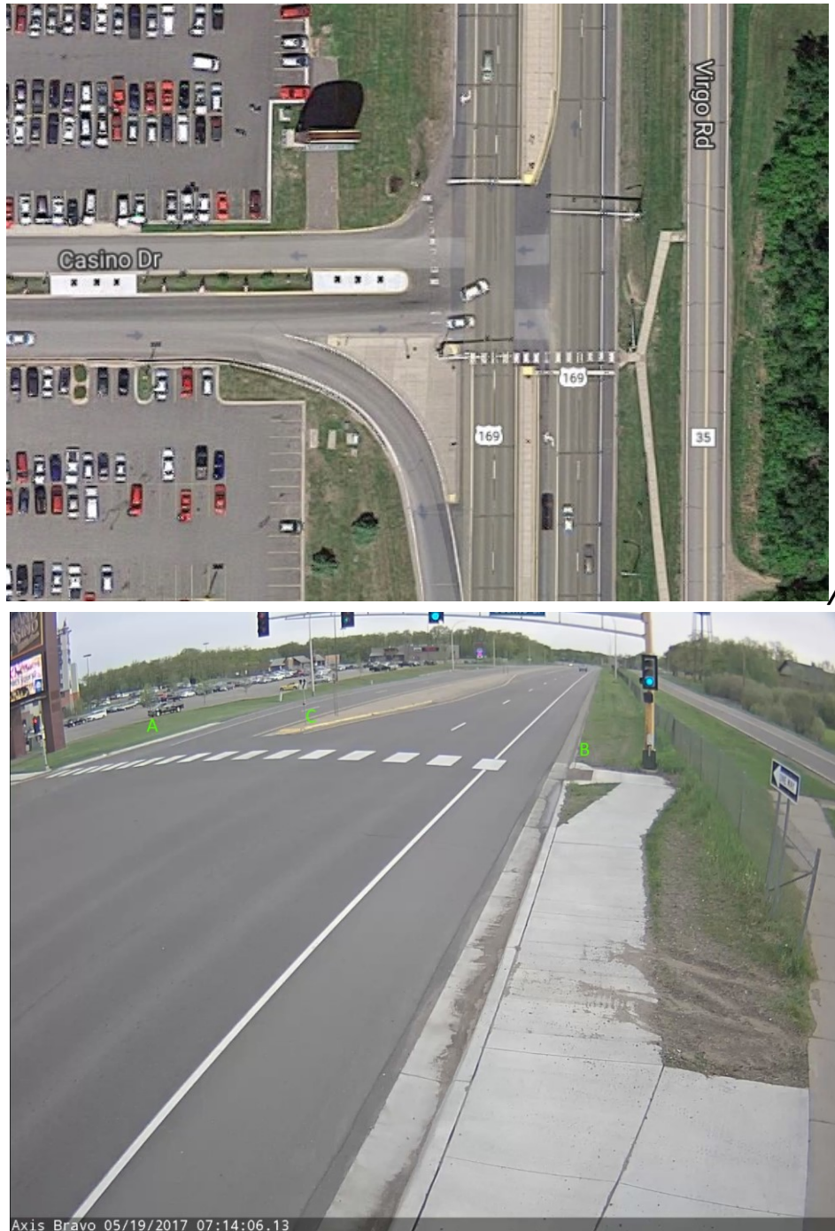
Figure 4.29 TH 169-Casino Drive Intersection: Plan View and Marked Crosswalk, Facing North.
