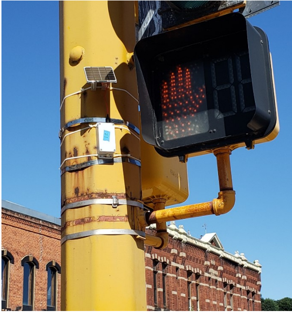
Figure 2.10 Images of Bluetooth Devices Attached to Signal Poles at Nelson St.
