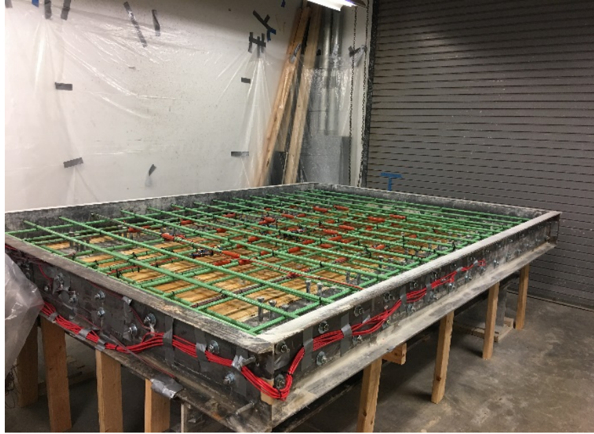
Figure 1. Photo. Deck before the pour.
