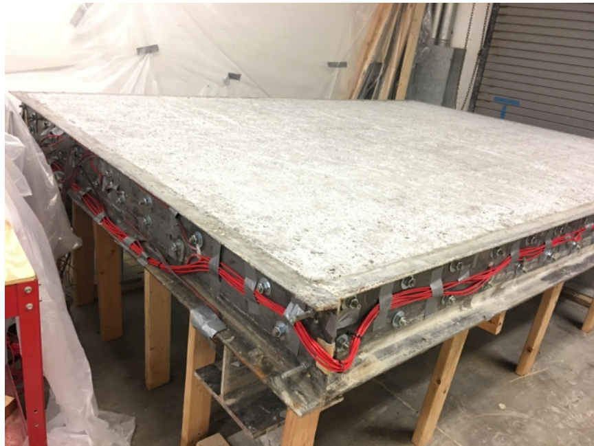
Figure 2. Photo. Concrete deck after the pour.
