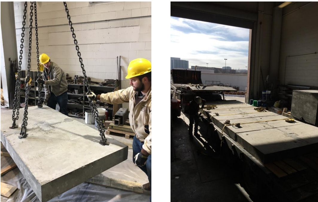
Figure 3.8: Slab Transportation
