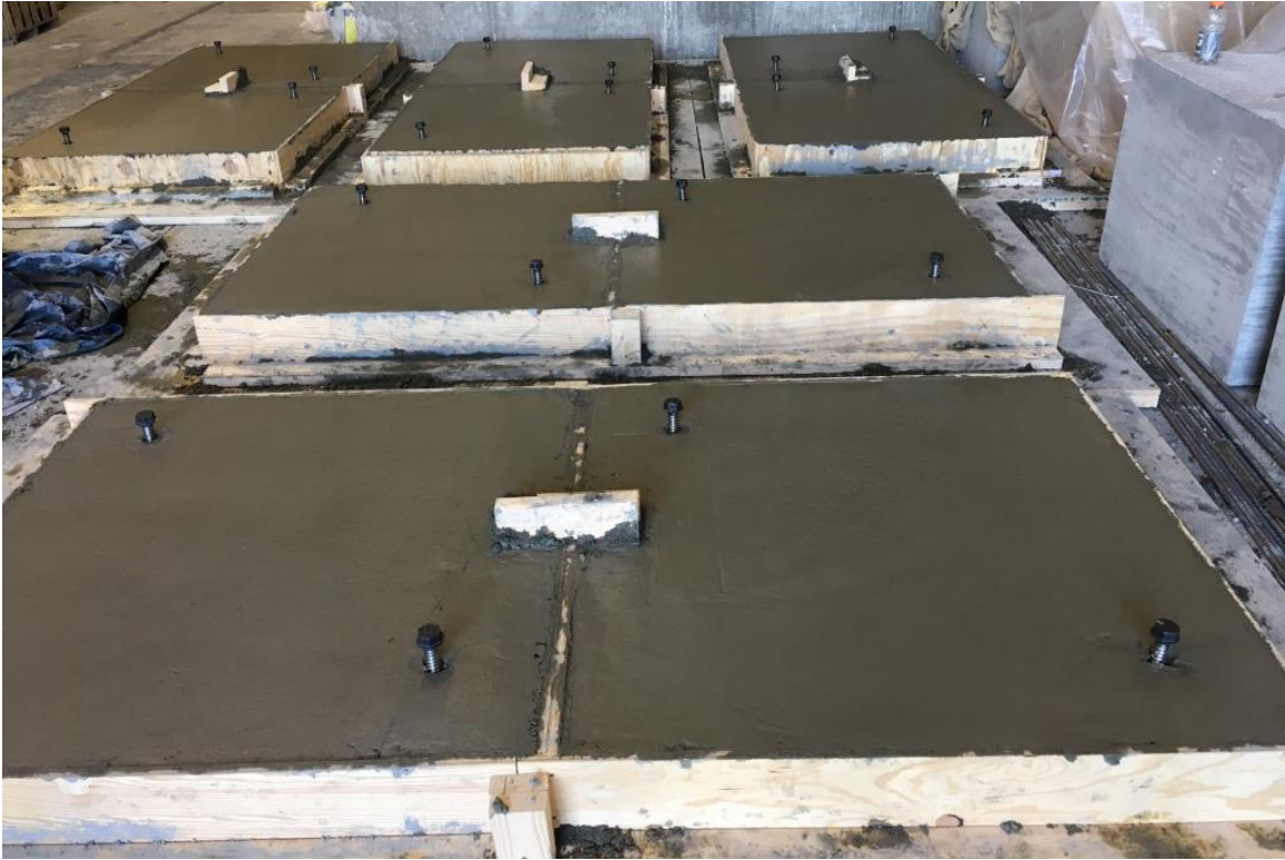
Figure 3.6: Finished Slabs After Anchor Placement
