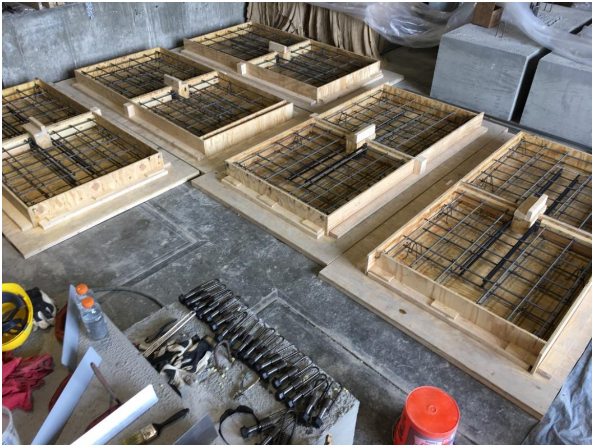
Figure 3.5: Formwork for Mechanical Connection Slab Panels
