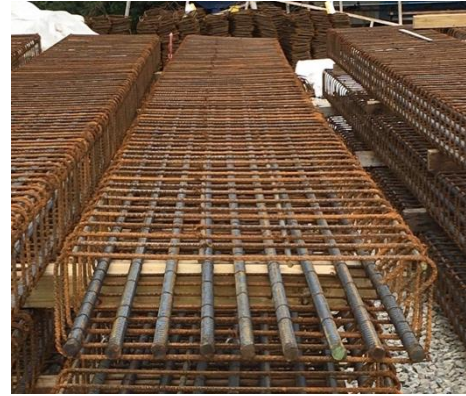
(b) Reinforcing steel cages
