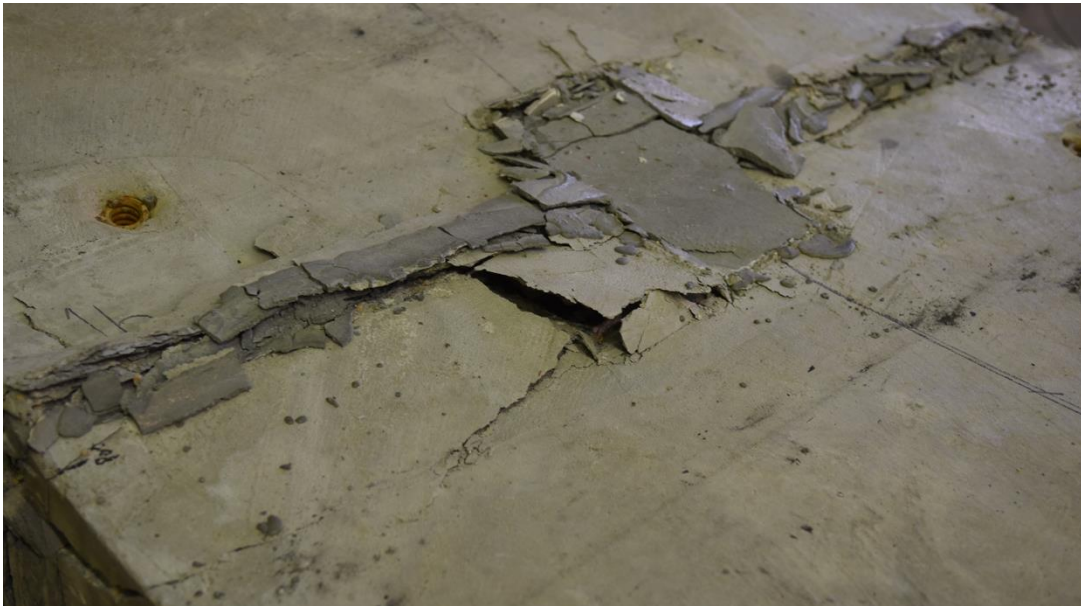
Figure 3.16: Specimen F-F-1 Joint Close-up Photo after Failure
