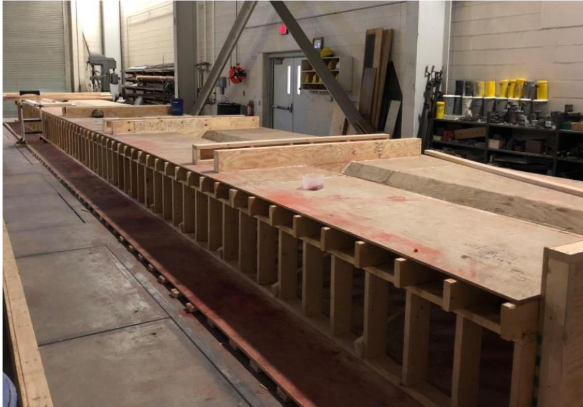
Figure 4.3: Full-Scale Formwork Assembly
