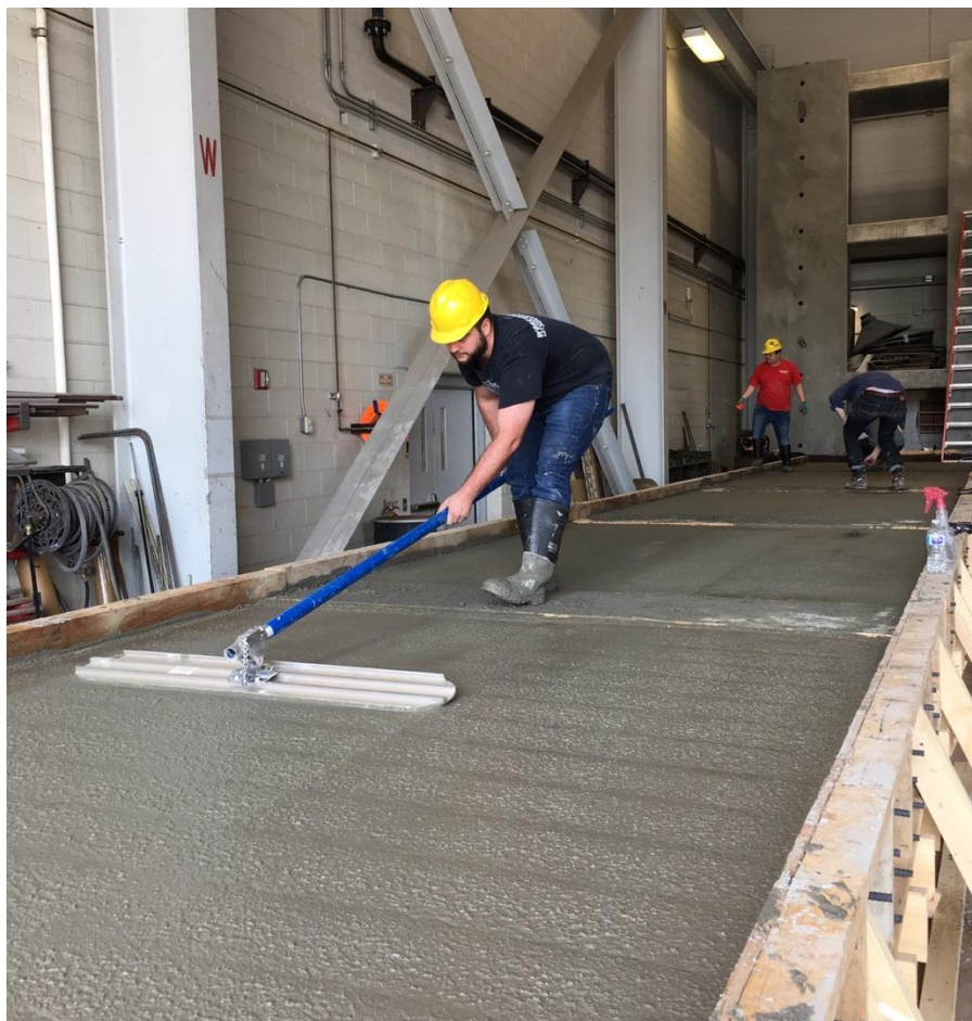
Figure 4.8: Finishing the Full-Scale Bridge Specimens
