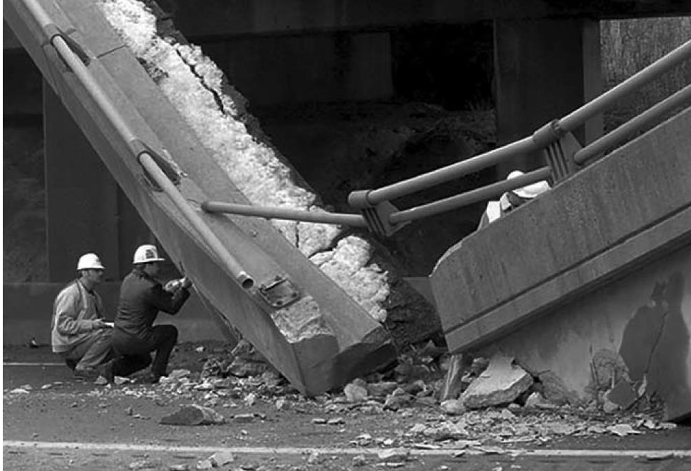
Figure 2.9: Forensic Examination of Non-composite Adjacent Precast Prestressed Concrete Box Beam Bridge Failure in Pennsylvania (retrieved from Naito et al., 2010)
