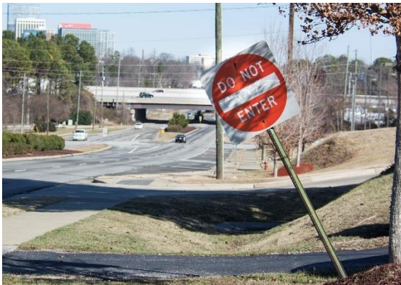
Figure 1.4 Example of damaged Signs: Non-aligned and Spray Painted
