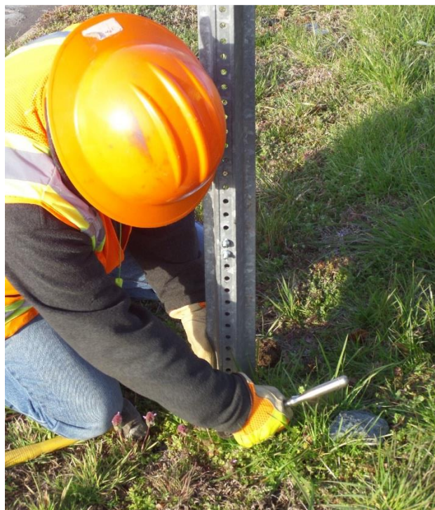
Figure 12.10 Worker Attaching the New Sign Pole to the Base Pole
