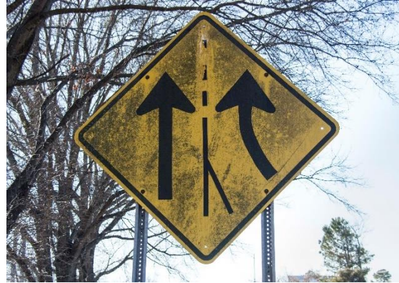
Figure 1.3 Example of Deteriorated and Damaged Signs: Faded and Tree Sap Content
