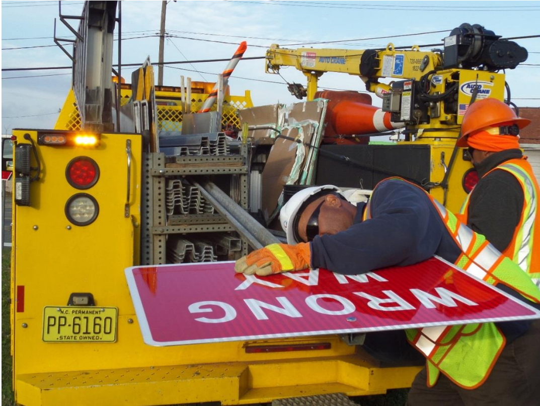
Figure 12.7 Assemble of the New Sign to the Pole
