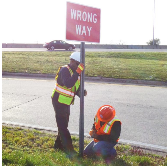
Figure 3.5 Crew Members Installing a Wong Way Sign
