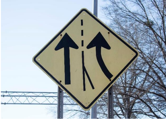
Figure 1.3 Example of Deteriorated and Damaged Signs: Faded and Tree Sap Content
