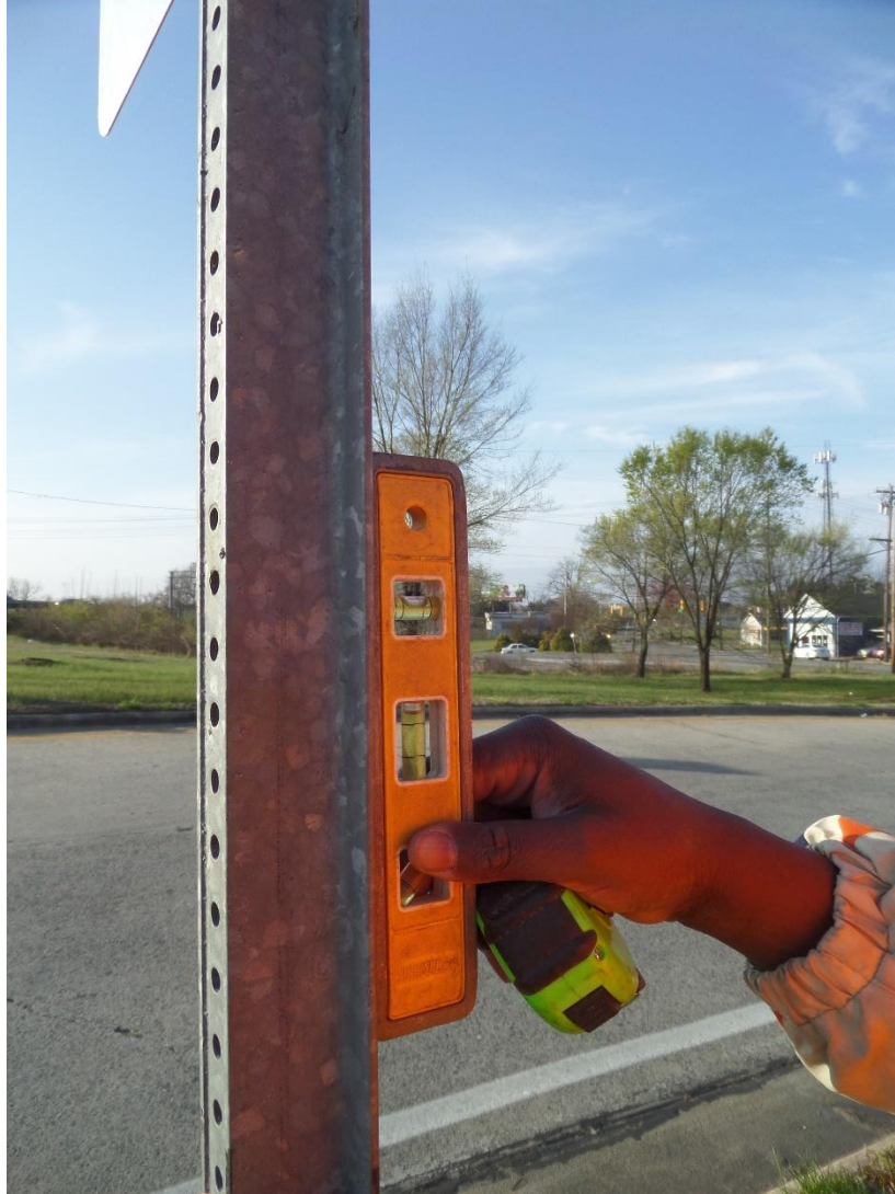
Figure 12.11 Crew Member Checking with a Level the Pole Alignment
