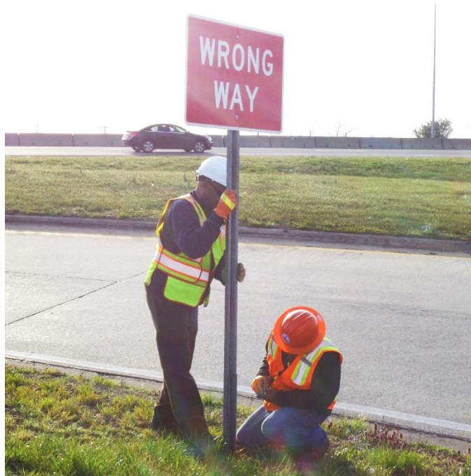
Figure 12.9 Crew Members Installing a New Sign
