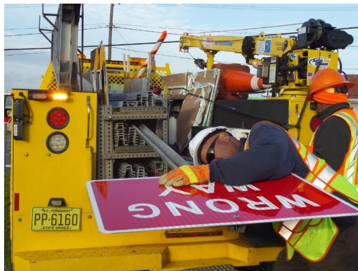
Figure 3.4 Assemble of a Wong Way Sign to the Pole
