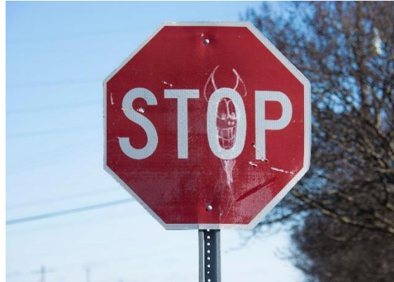
Figure 1.4 Example of damaged Signs: Non-aligned and Spray Painted
