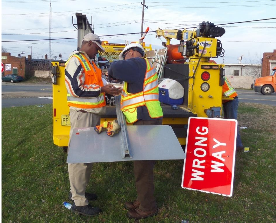
Figure 12.5 Separating the Deficient Sign from the Sign Pole
