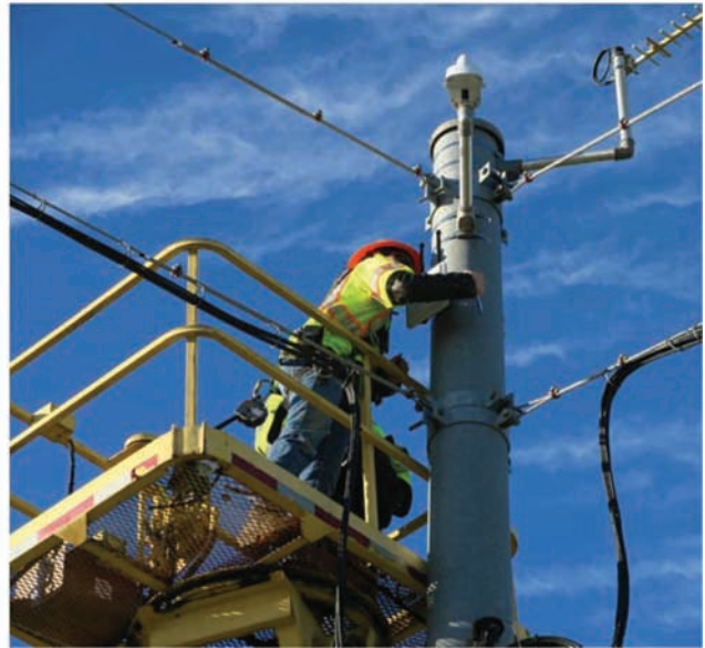
Figure 2.9 RSU deployment at US 231/Martin Jischke Drive in West Lafayette, IN.
